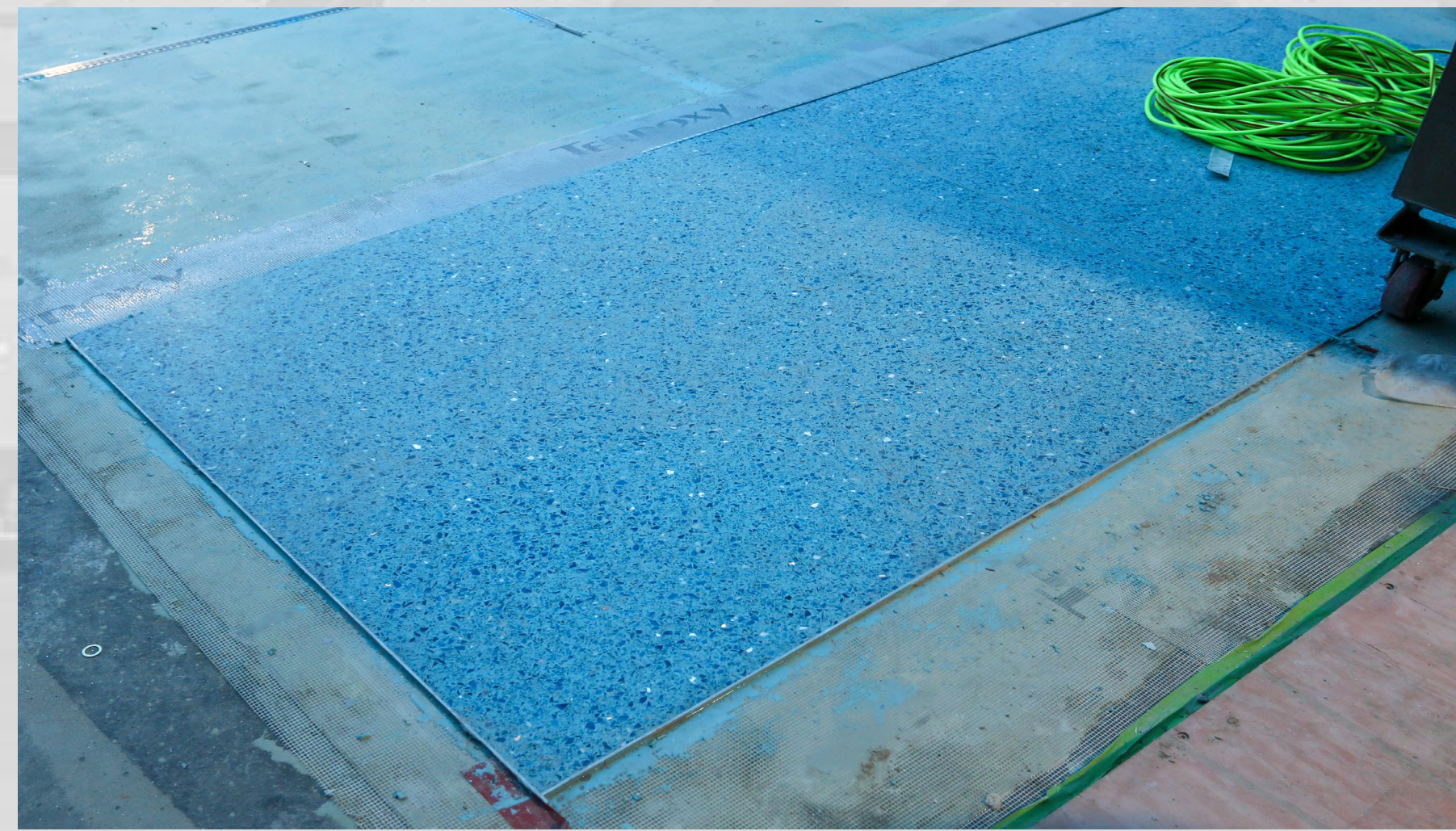
Terrazzo Floor Mock-up
