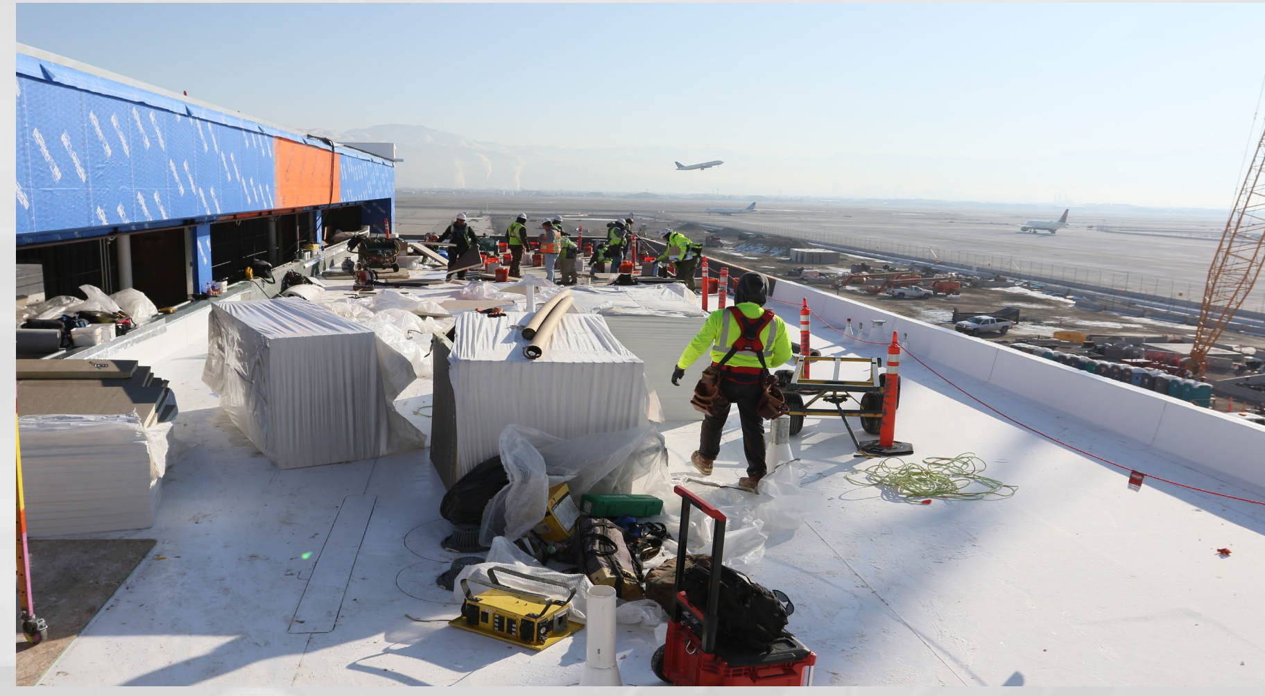
Low Roofing Installation
