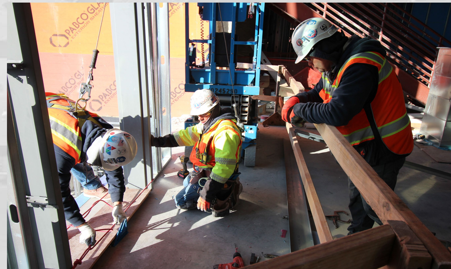
Level 2 Passenger Boarding Door Framing
