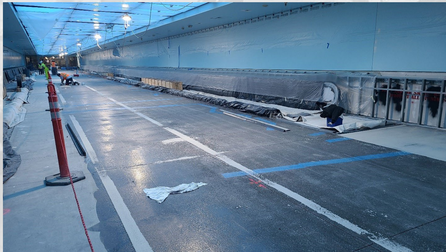
Central Tunnel Finishes
