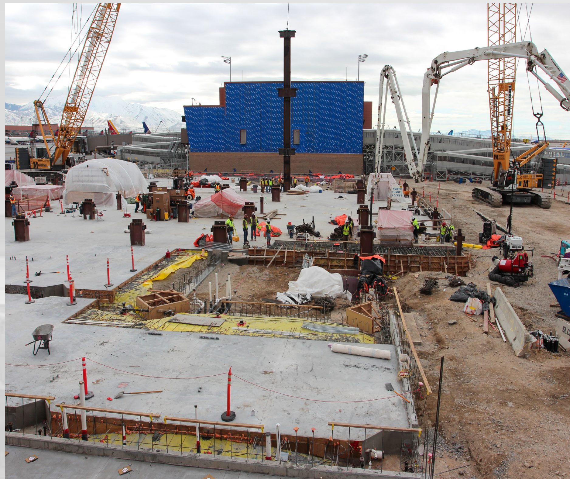
Steel Erection Day One – 2/20/2023
