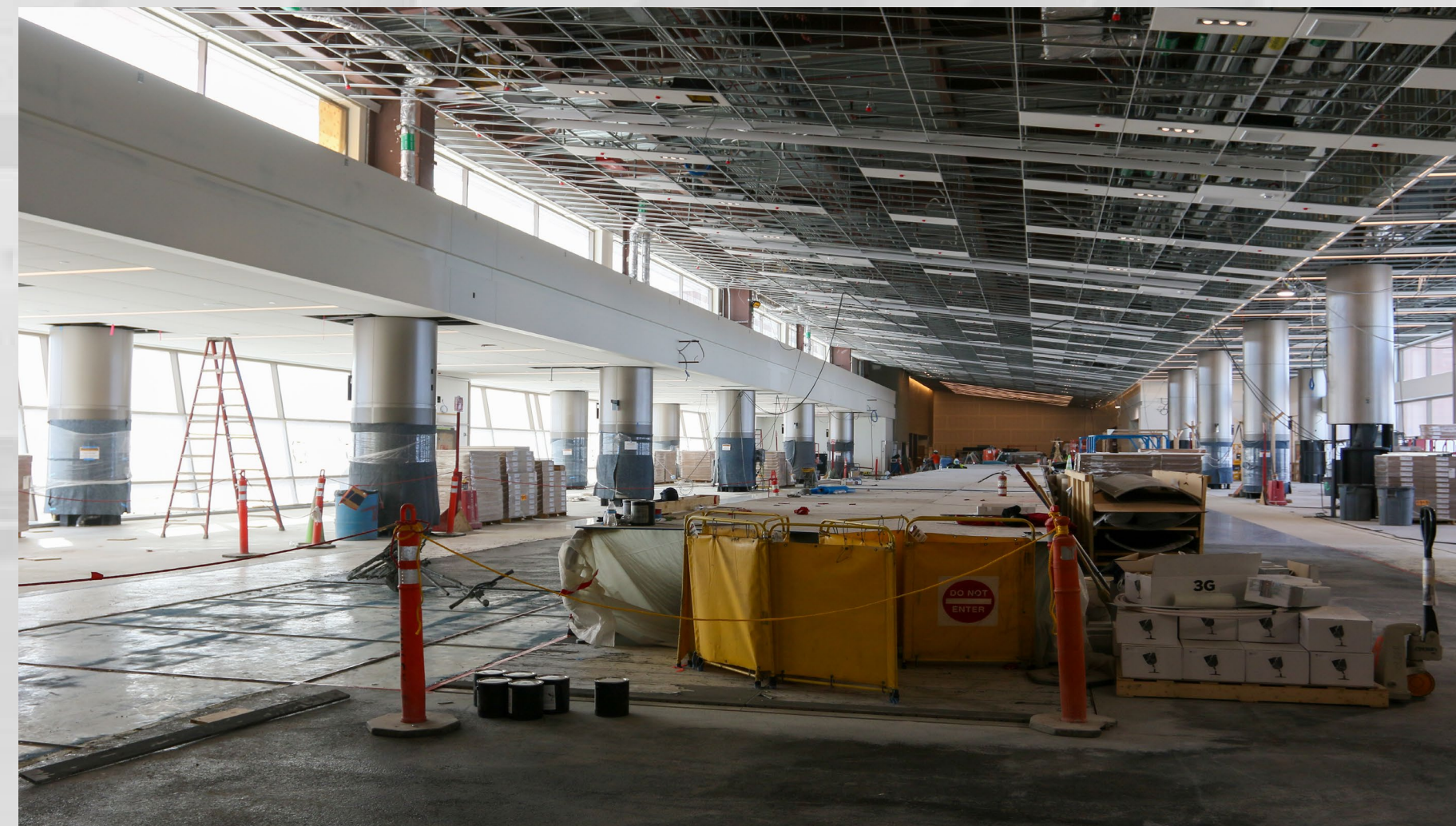
Area D Looking West at Temp Wall
