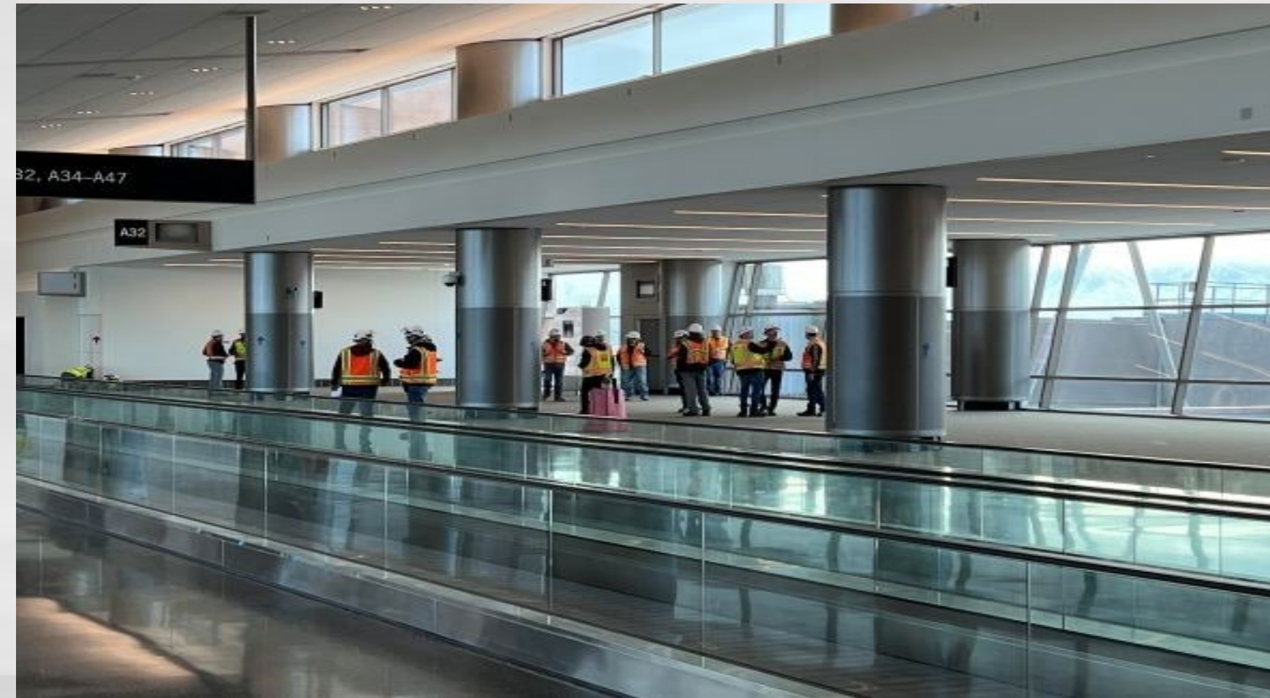
Holdroom Punchlist Underway
