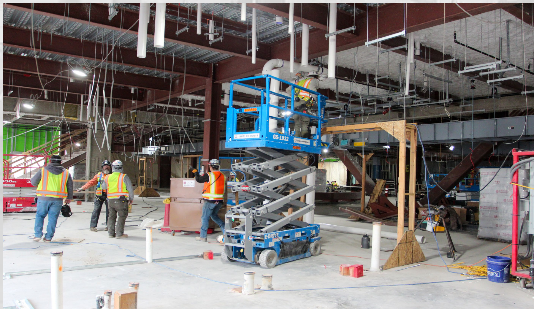
Level 1 Mech, Elec, Plumbing Rough-in
