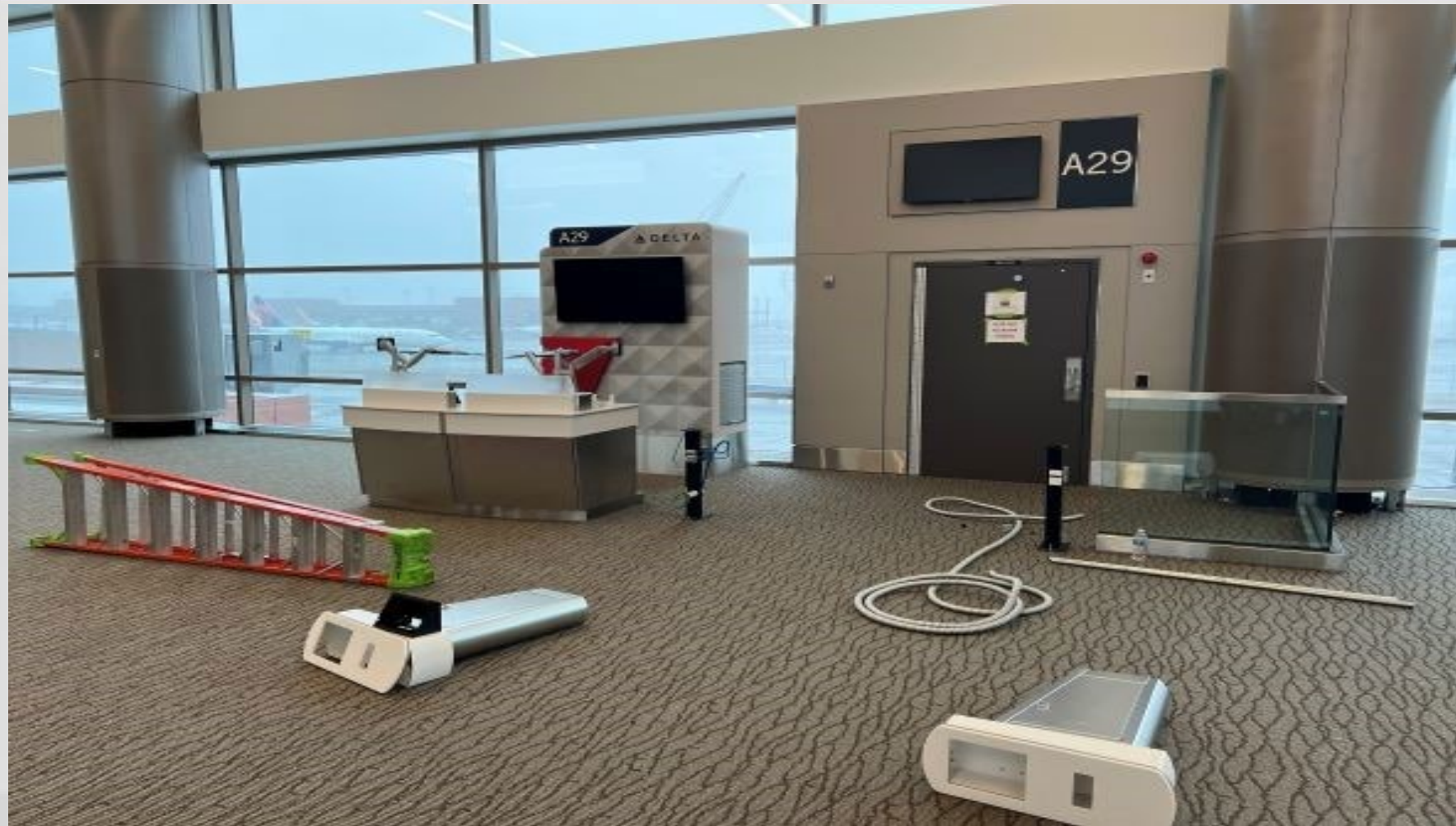
Gate IT Installation
