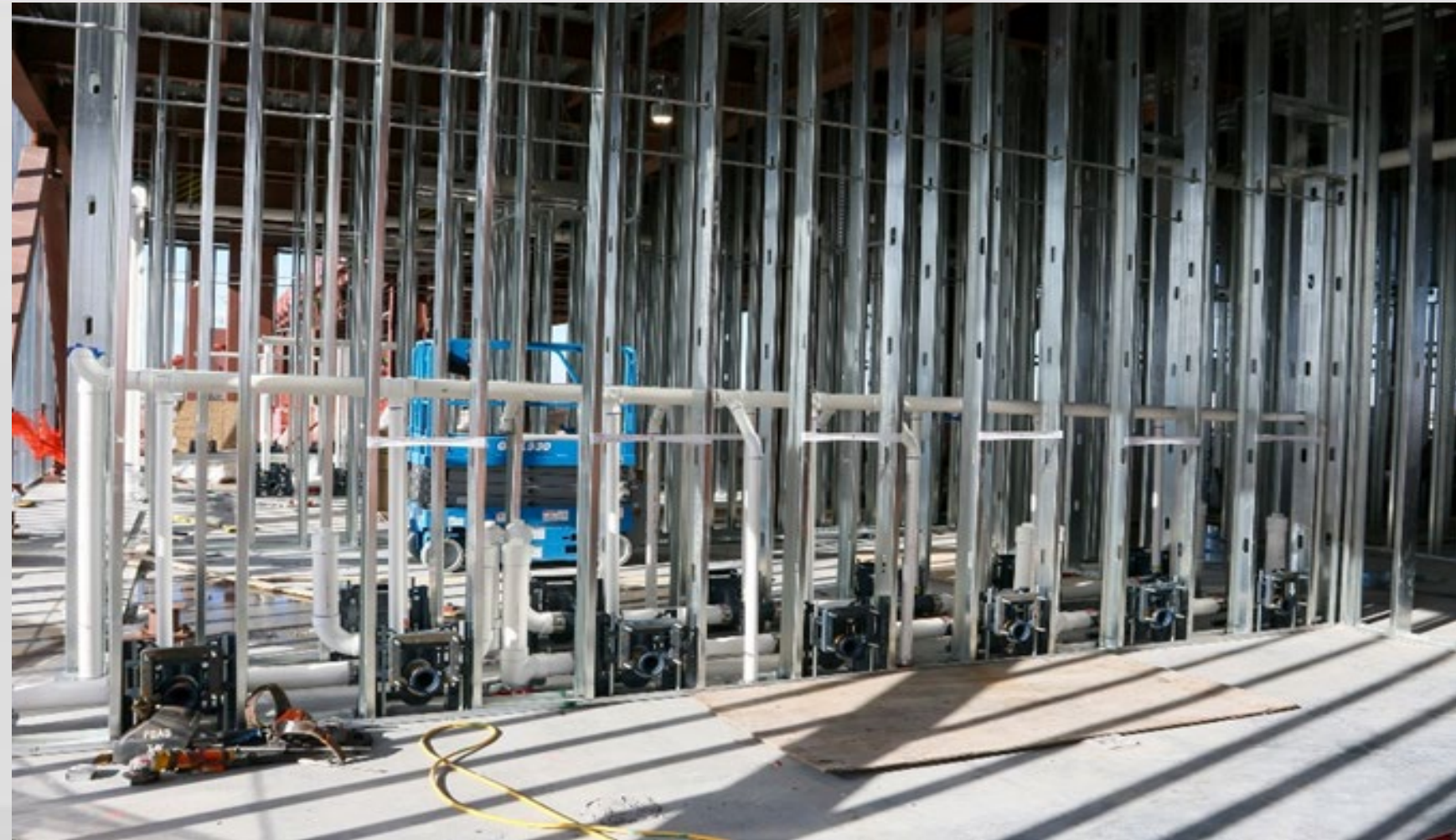
Public Restroom Studs and Carriers
