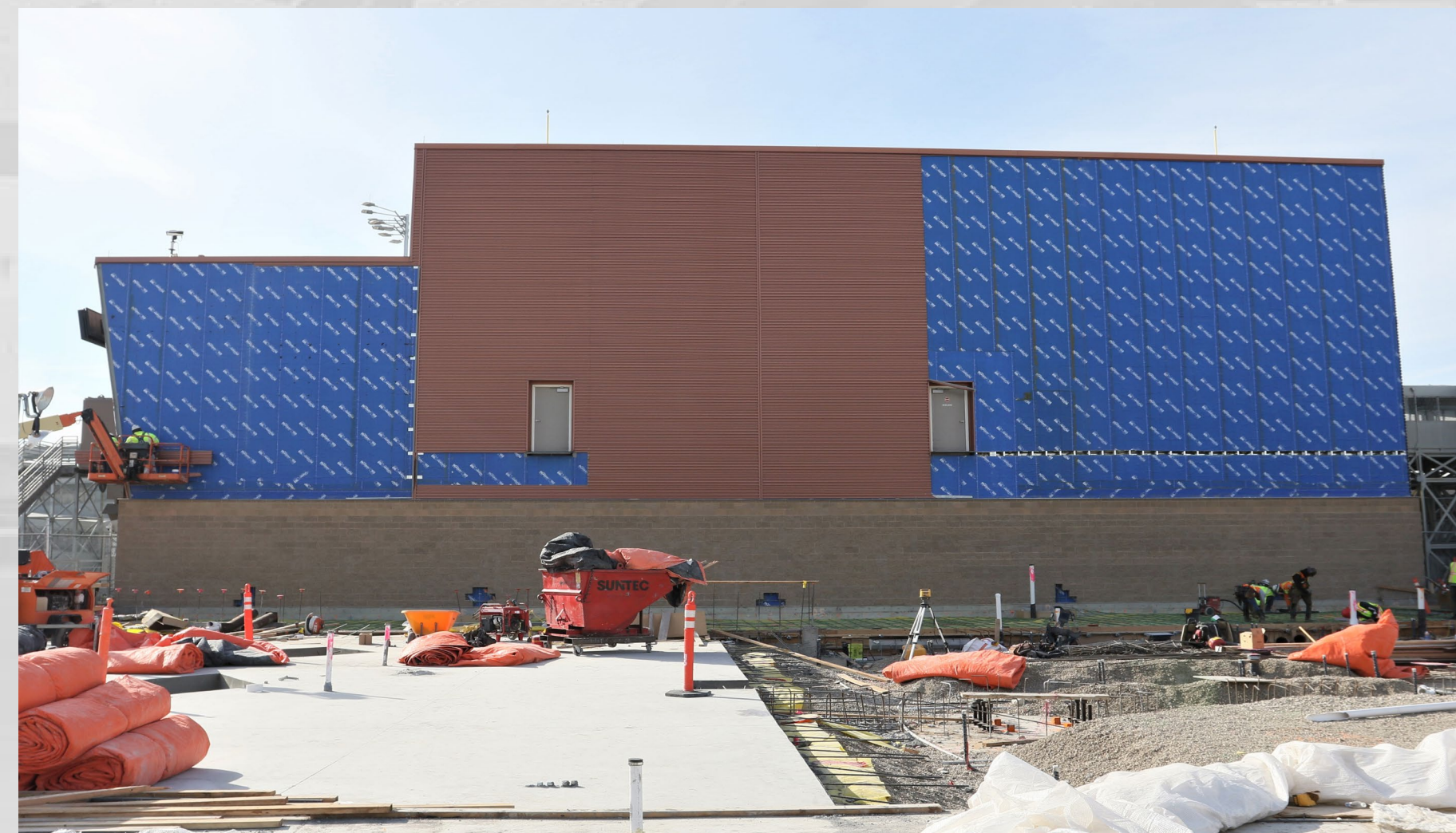
Phase 1 Exterior Panel Removal
