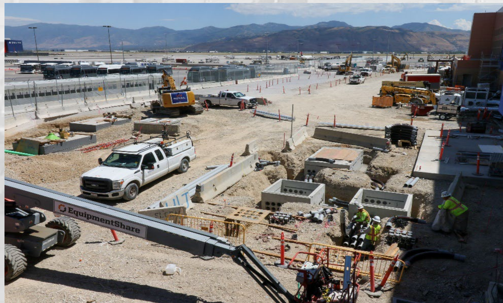
South Side Apron Paving
