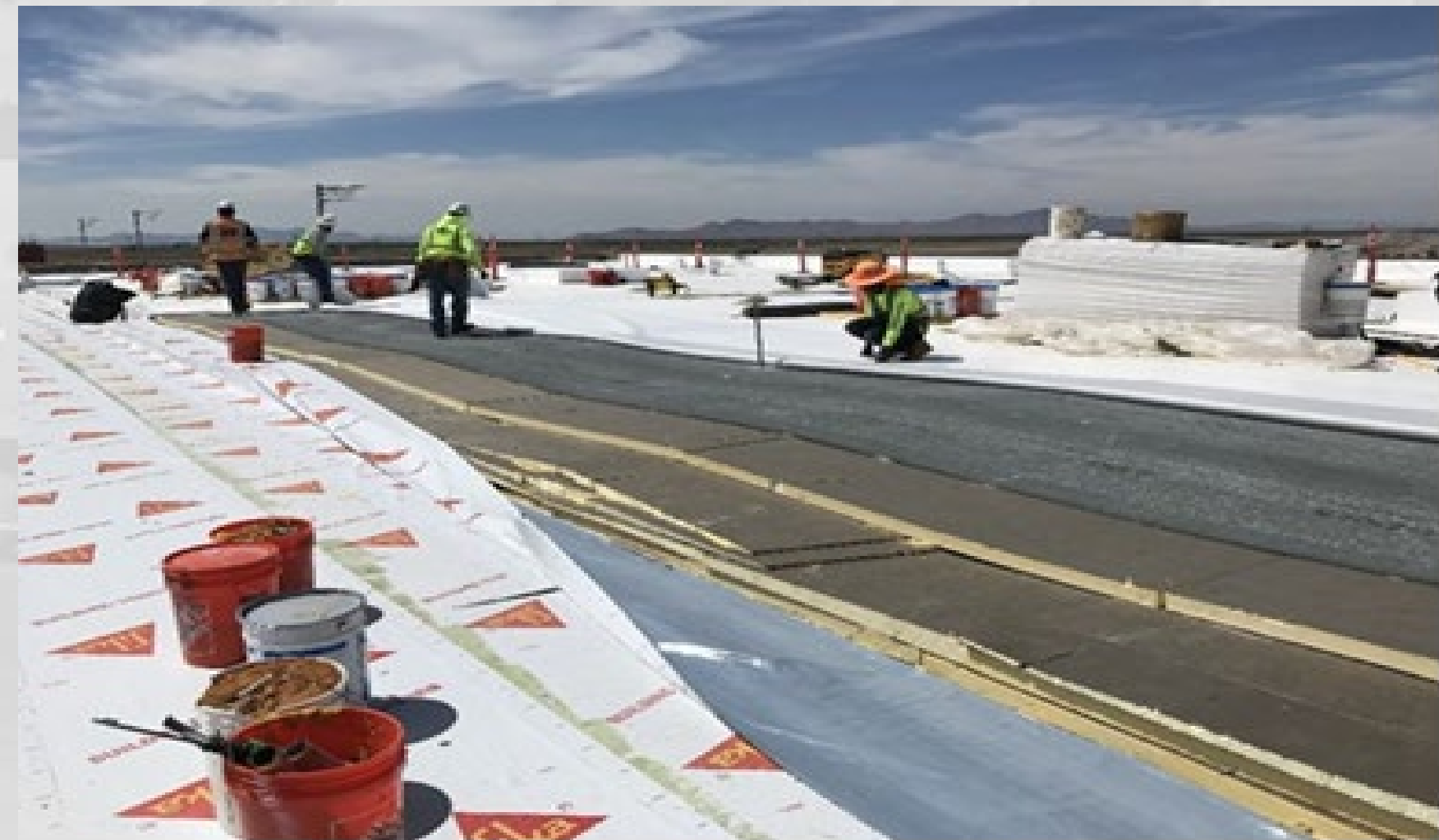
Area G Roofing
