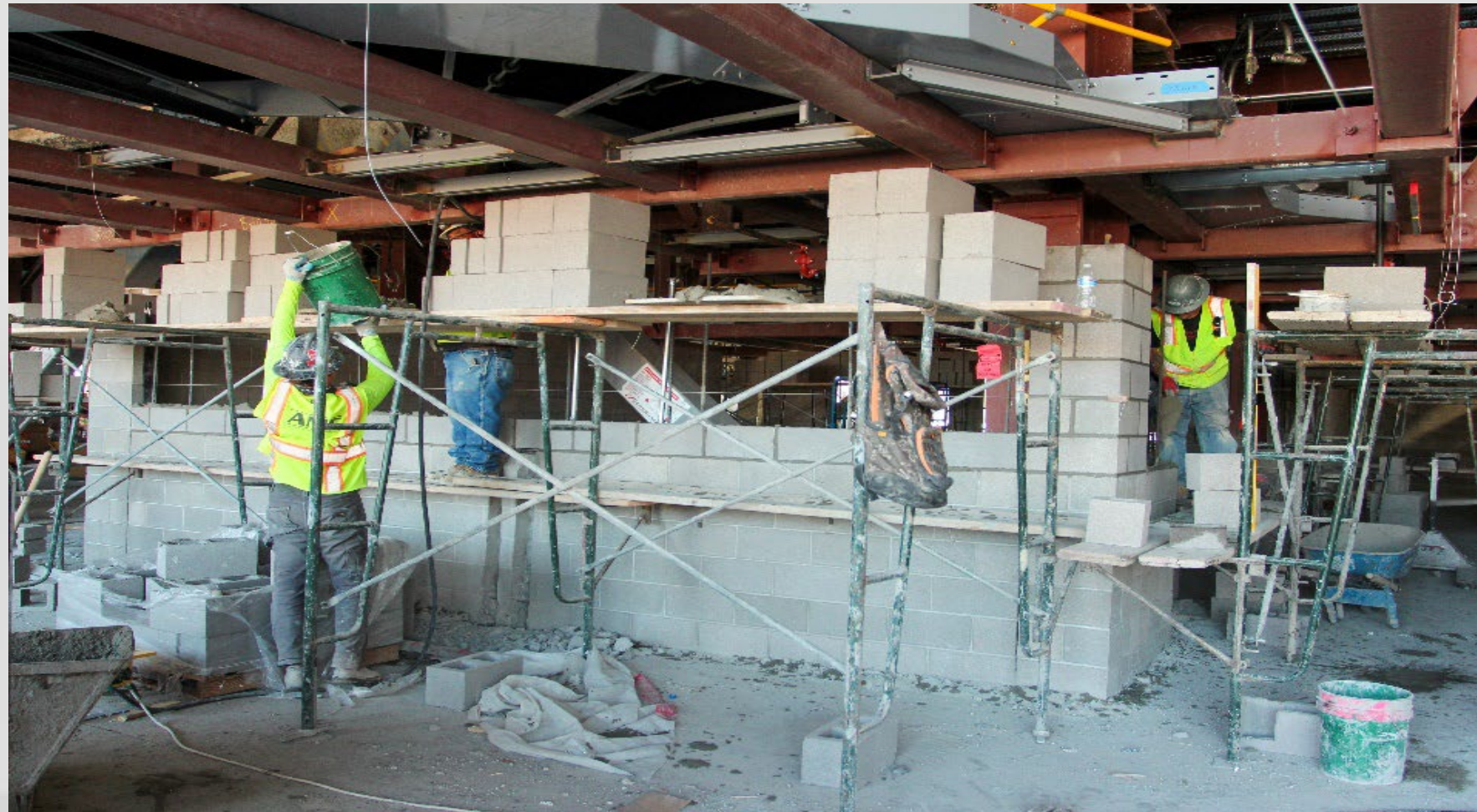
Level 1 Masonry Walls
