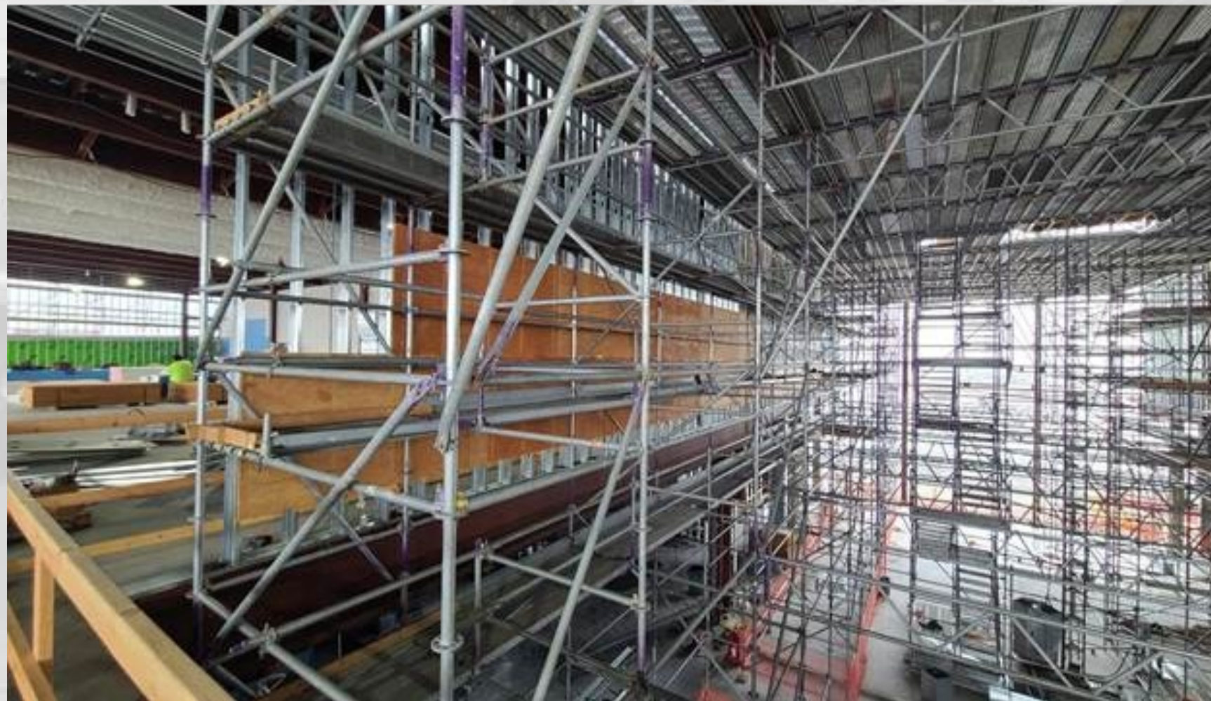
Canyon High Ceiling Scaffolding
