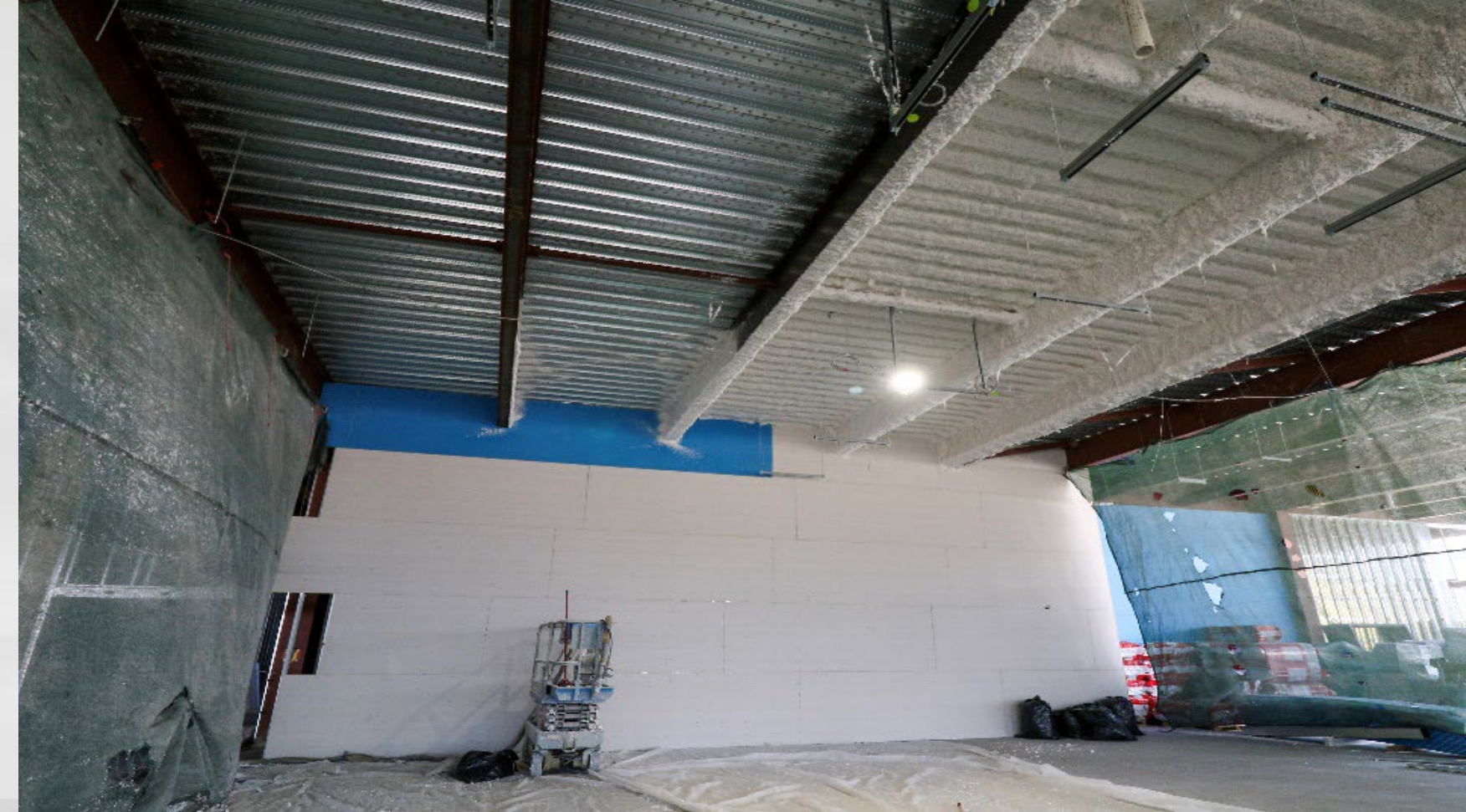
Level 3 Spray Fireproofing
