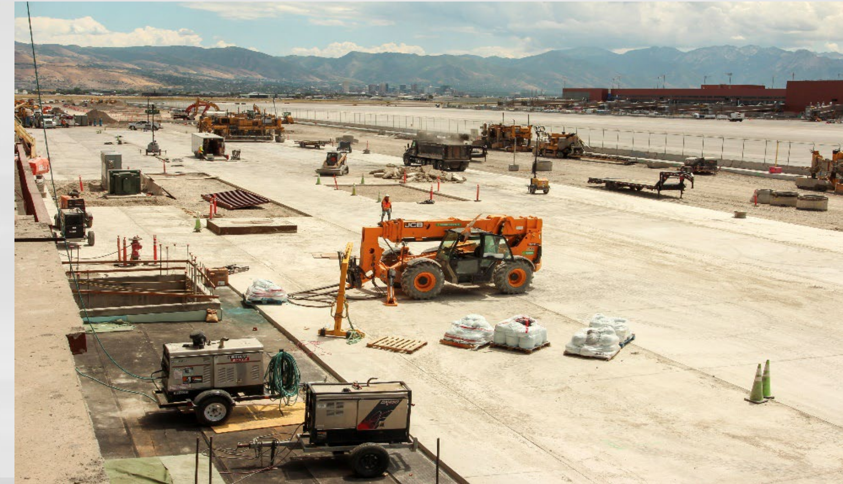
South Side Apron Paving
