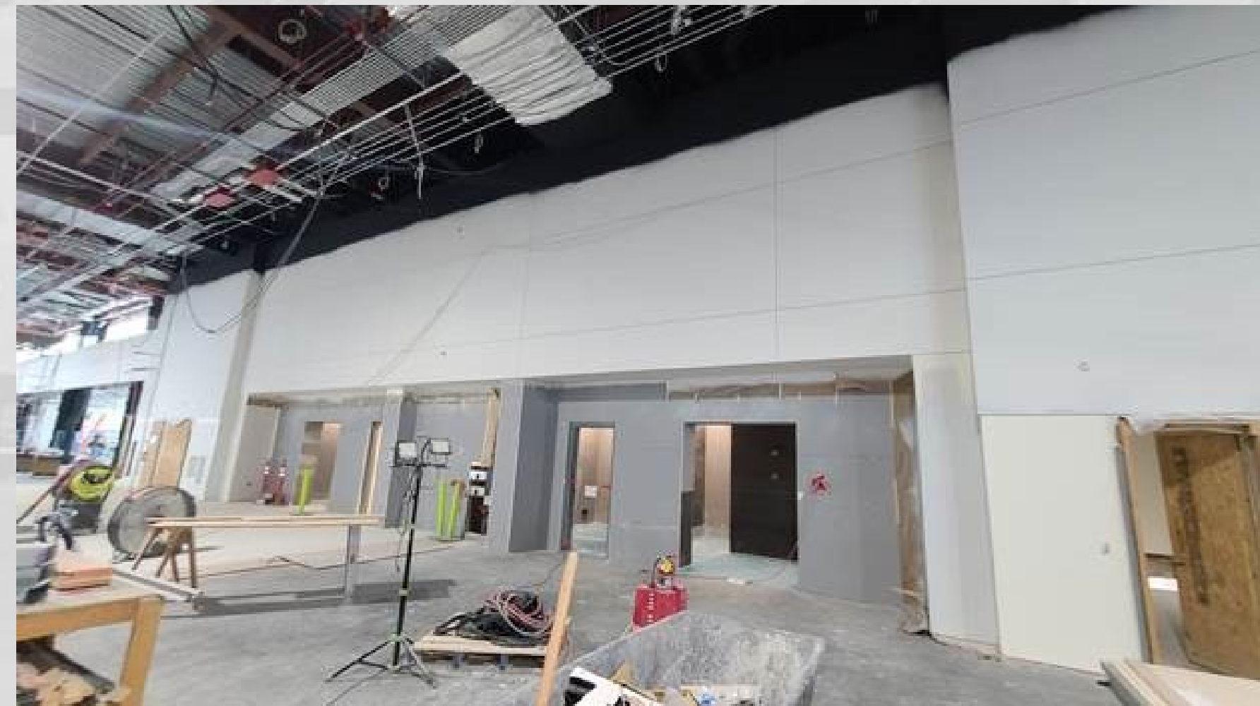
Level 2 Restroom Build-out
