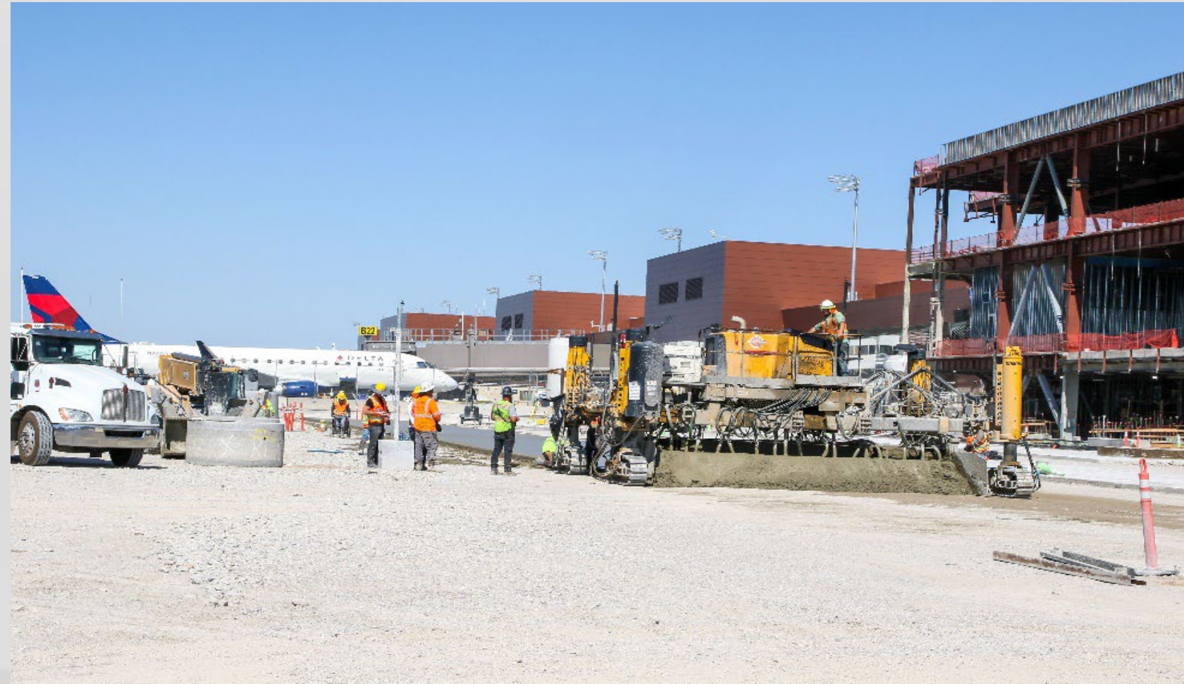
South Side Apron Paving
