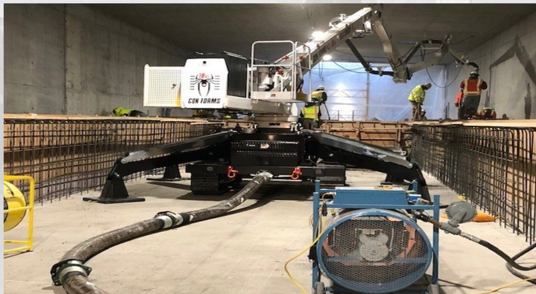
APM Platform Concrete Placement
