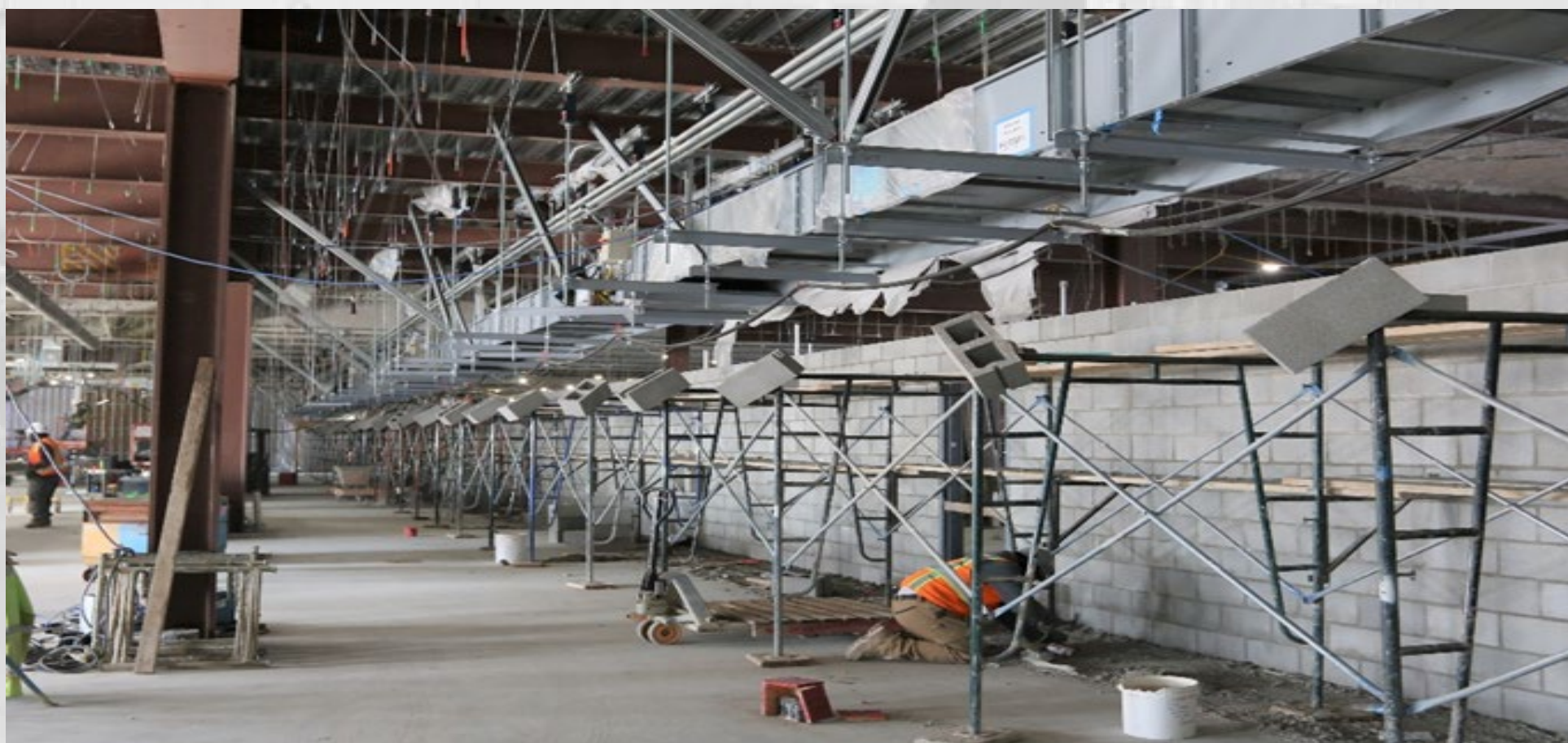
Level 1 Area C Interior Masonry
