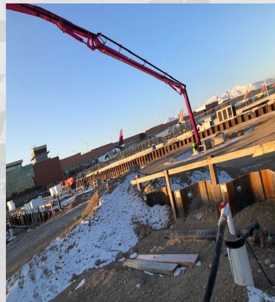
Concrete Hose from Truck into Tunnel to Spider
