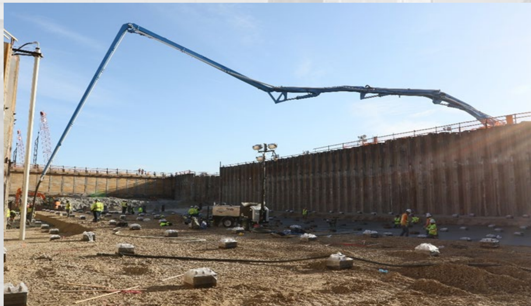
Mud Slab Concrete Placement
