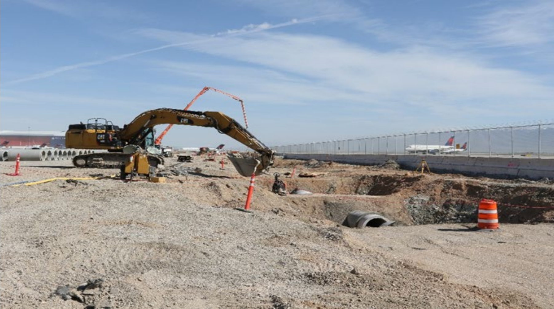
60" Storm Line Installation
