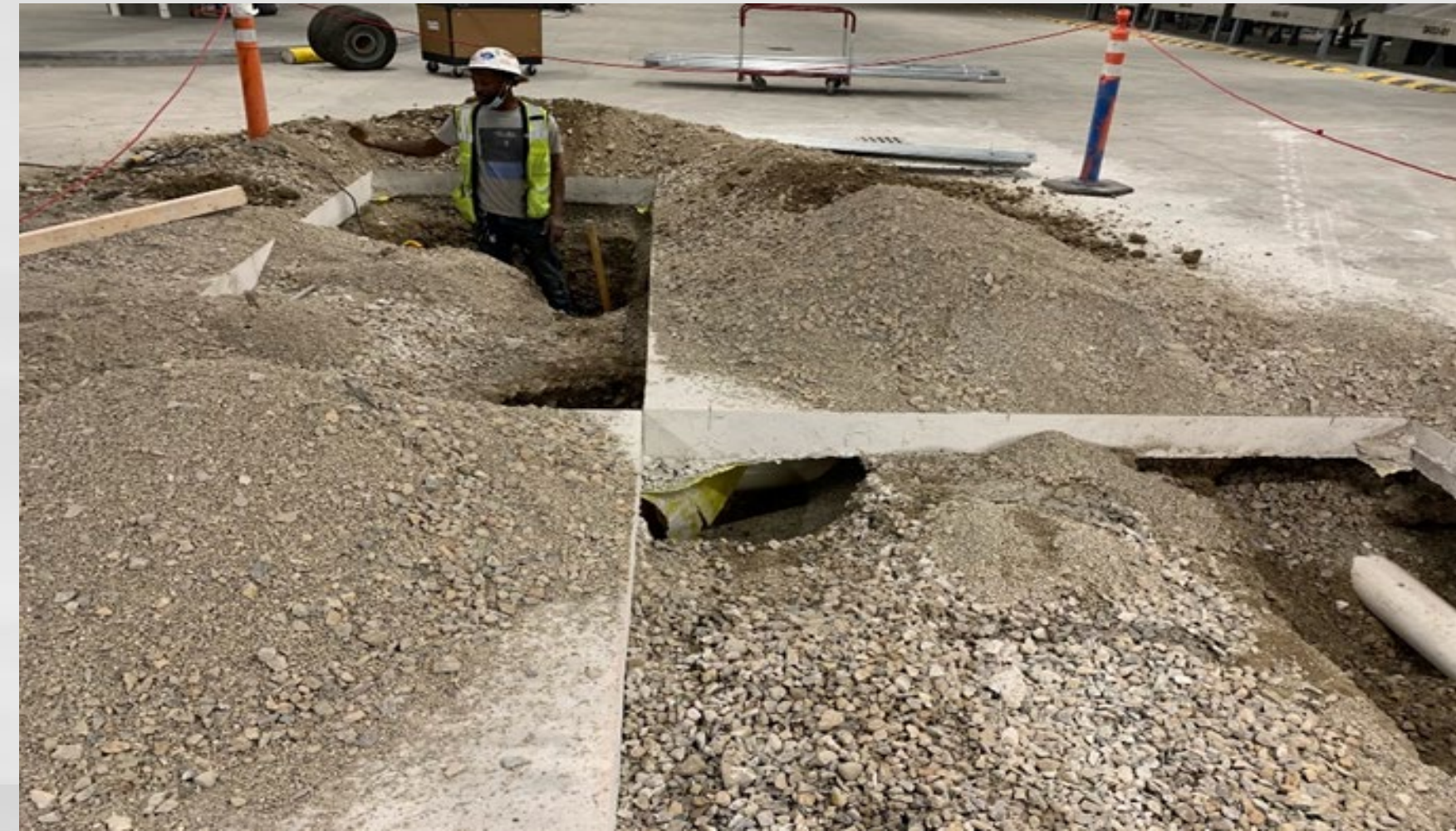
Restroom Underground Rough-in
