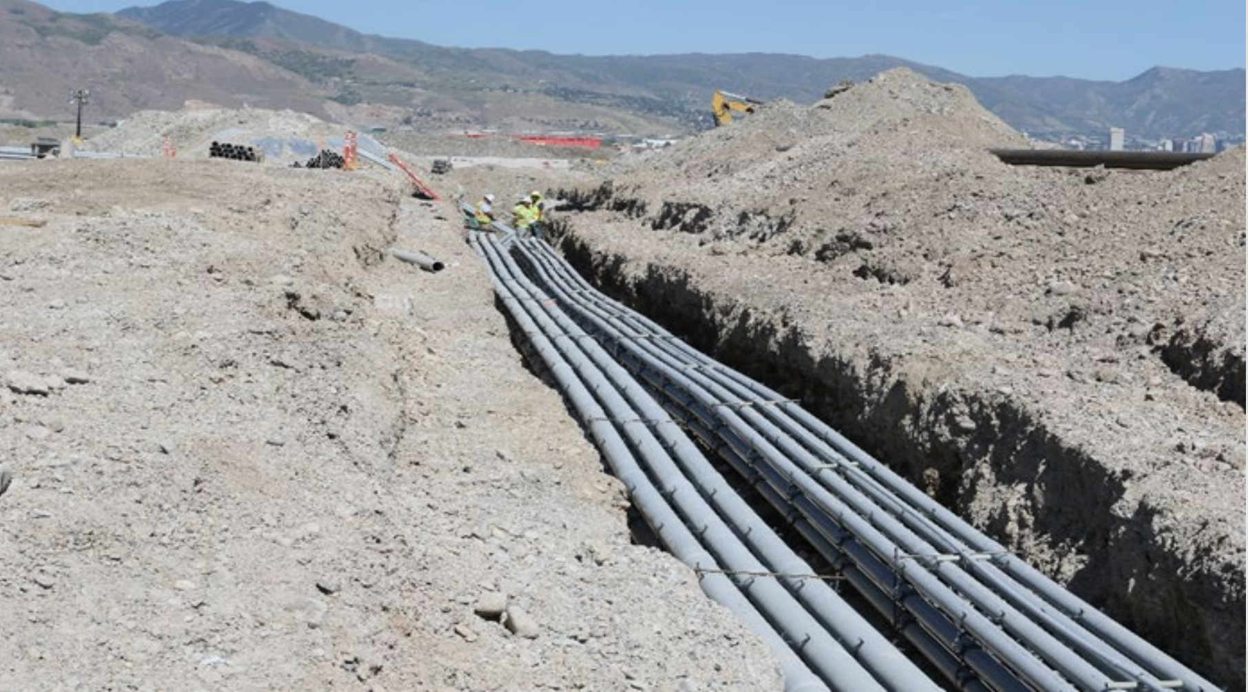
Ductbank Installation
