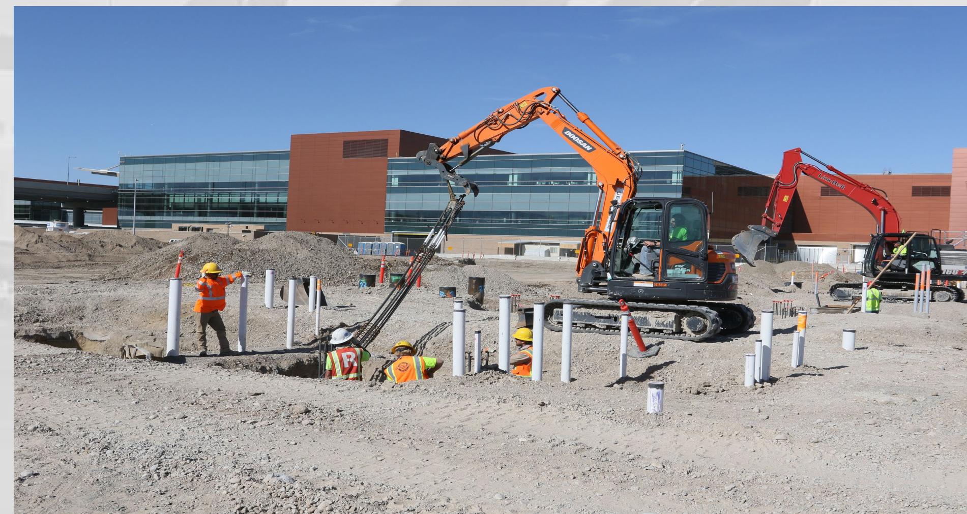
Underground Mechanical, Electrical, Plumbing
