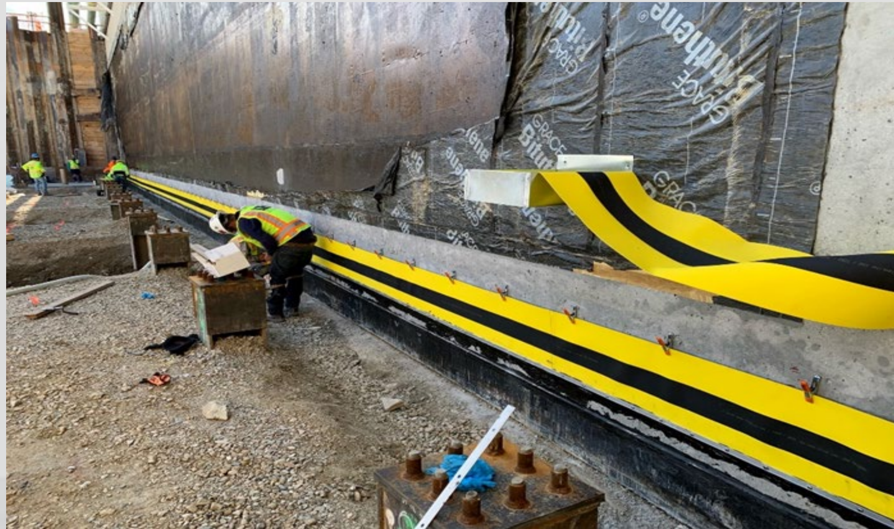
Central Tunnel/Terminal Joint/Waterproofing
