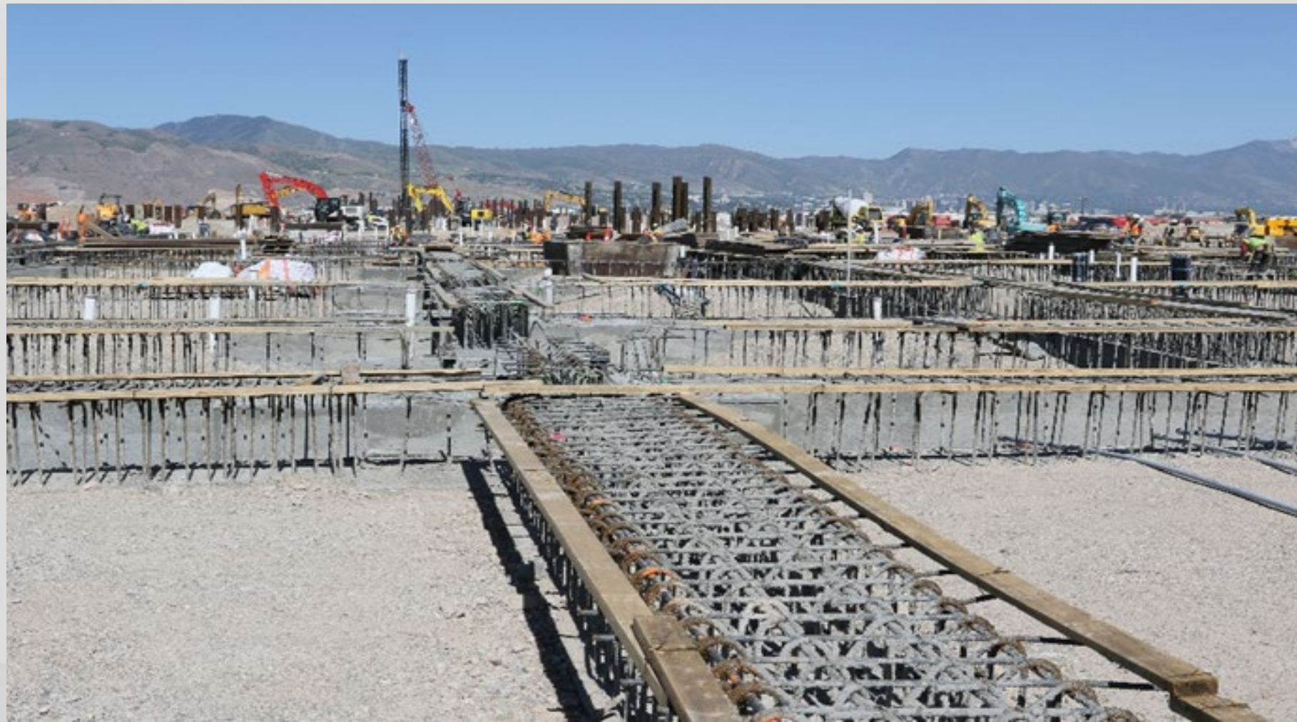
Grade Beam Reinforcing Steel
