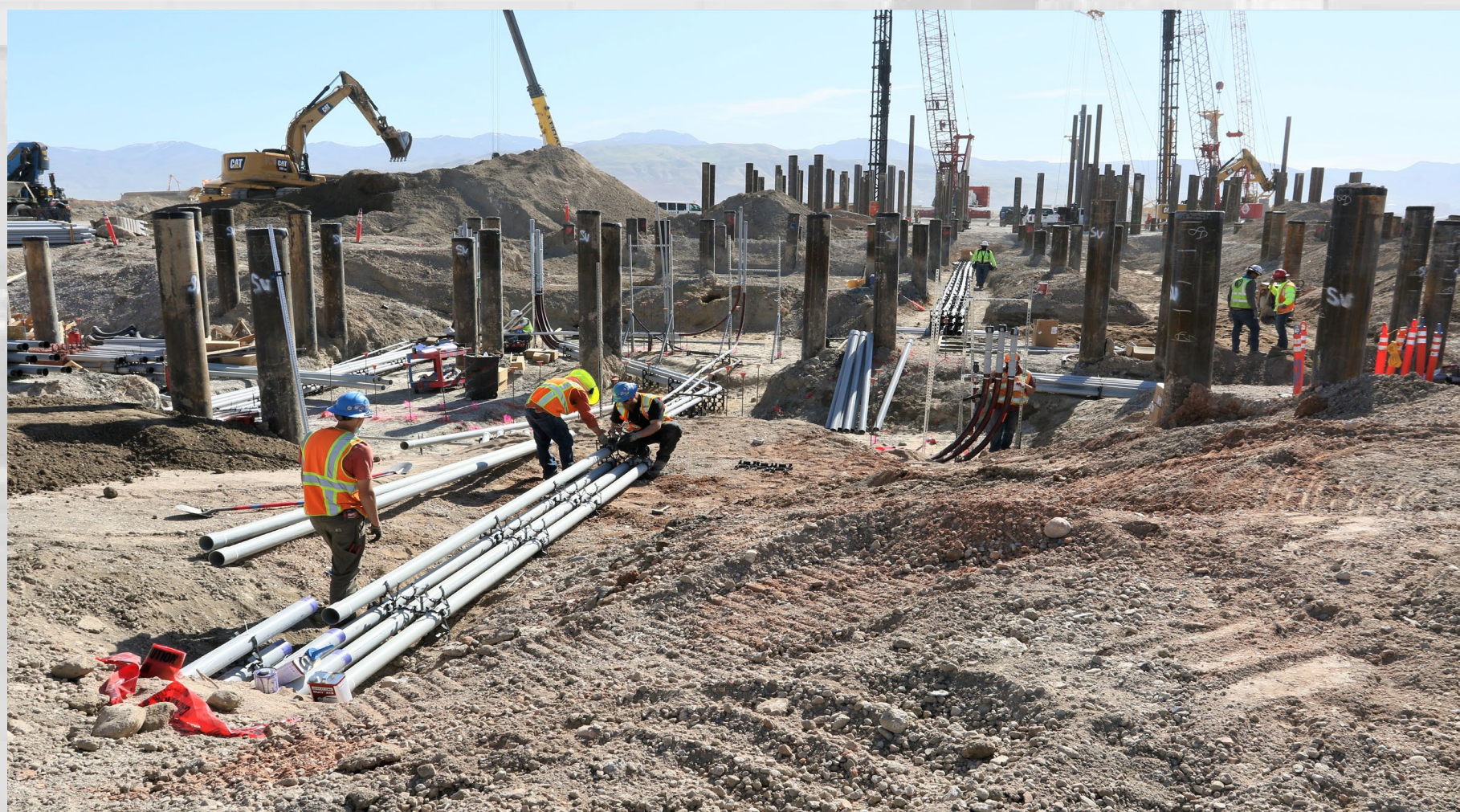
Underground Mechanical, Electrical, Plumbing
