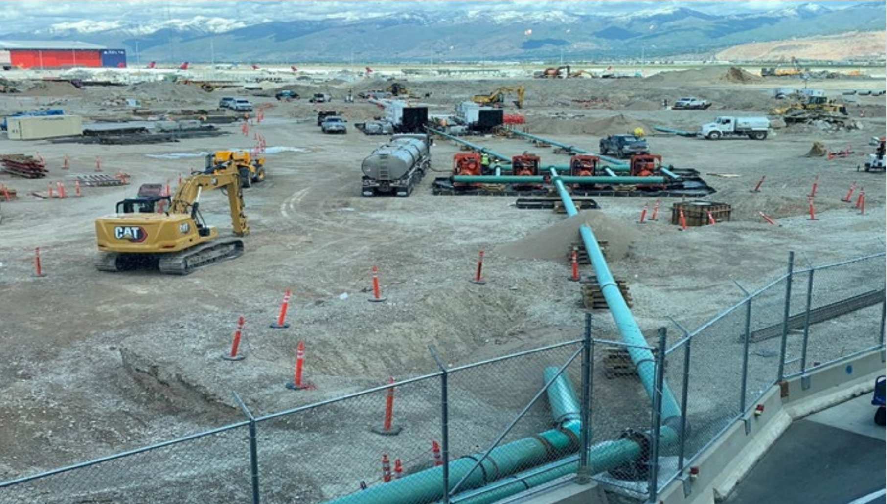
Fuel Line Flushing
