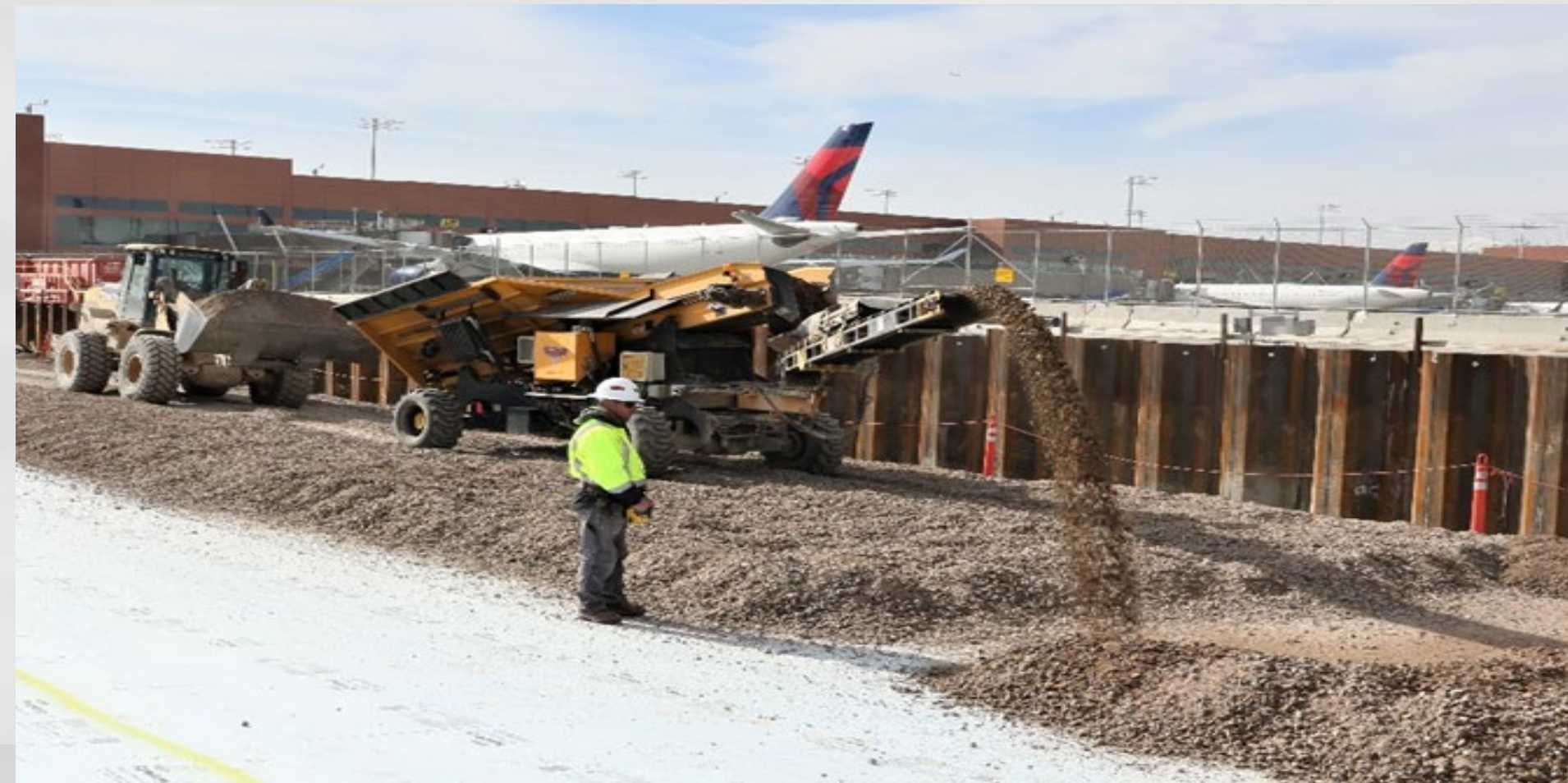
Area C Backfill
