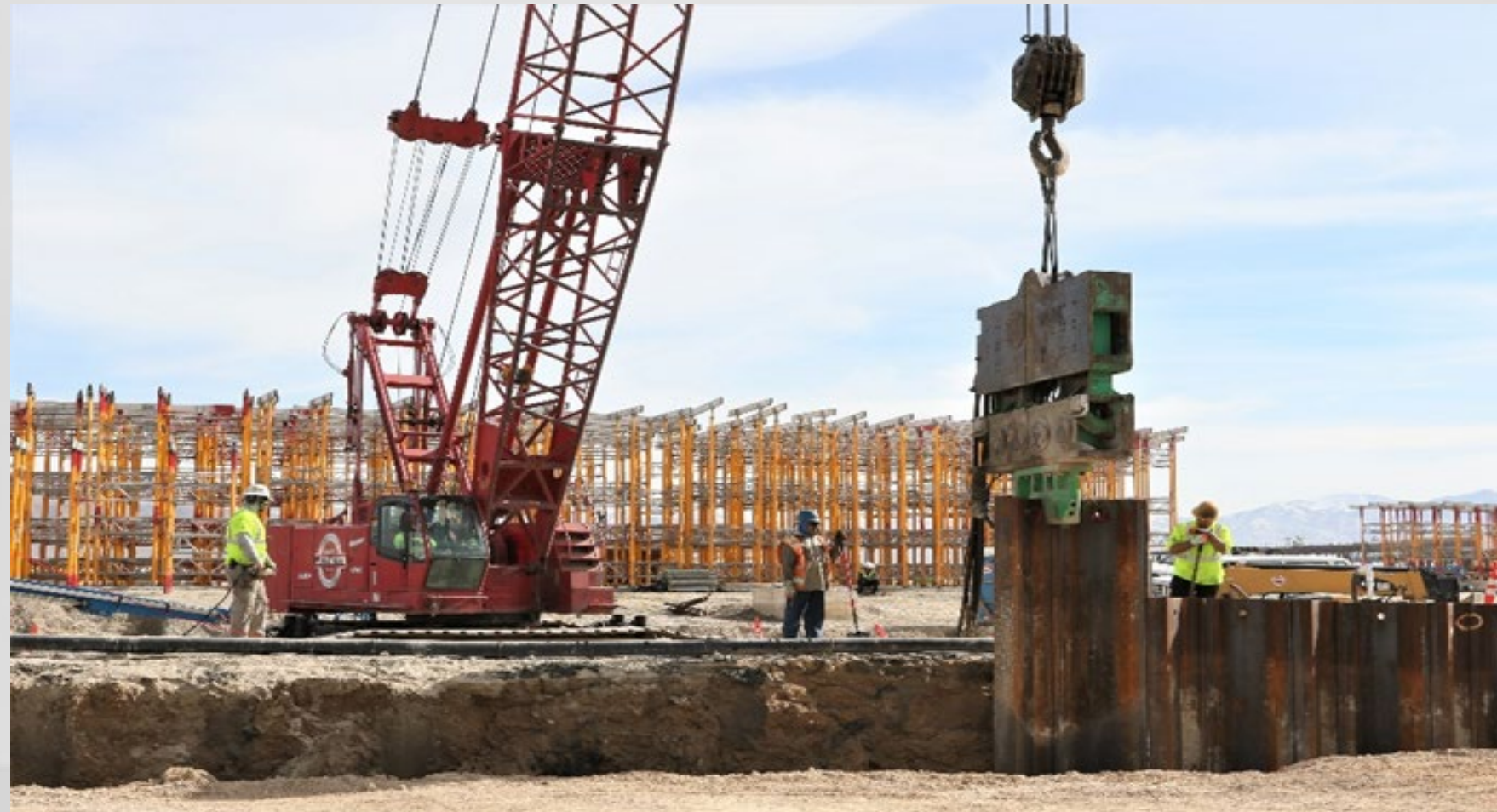
Area B Sheet Pile Removal
