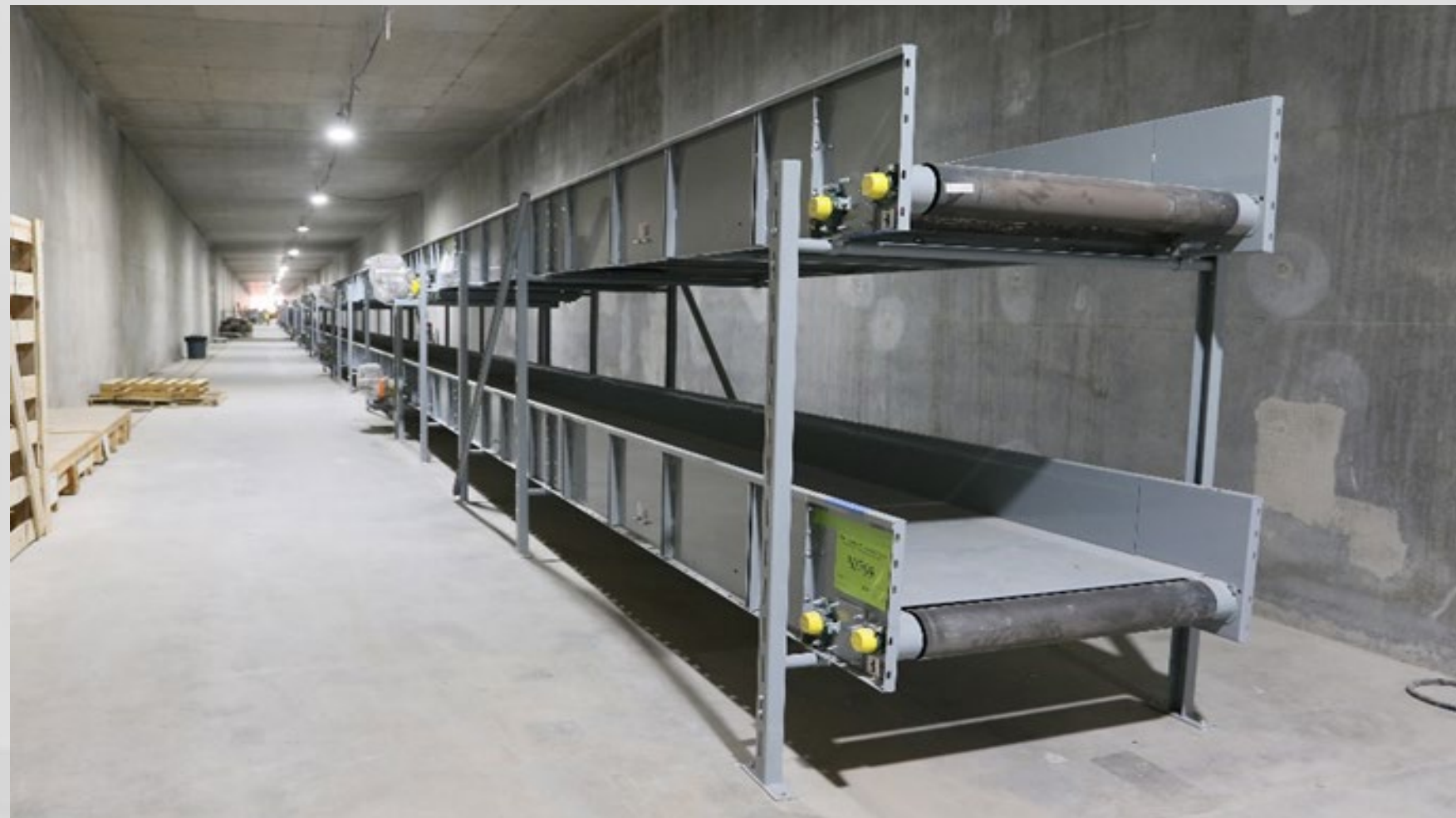
Baggage Conveyor Installation
