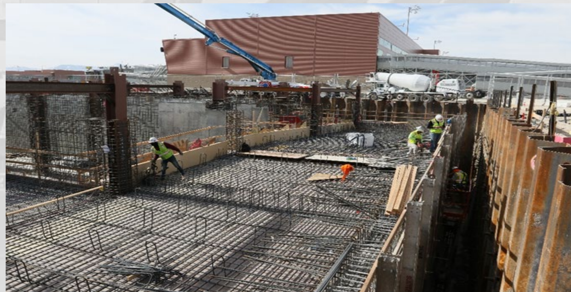
Area G (Concourse B Node) Lid Framing
