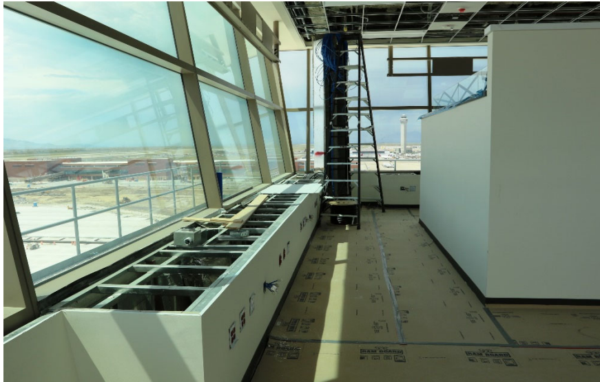
Ramp Control Tower
