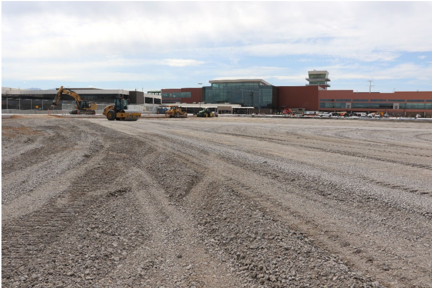
Site Grading near Concourse D
