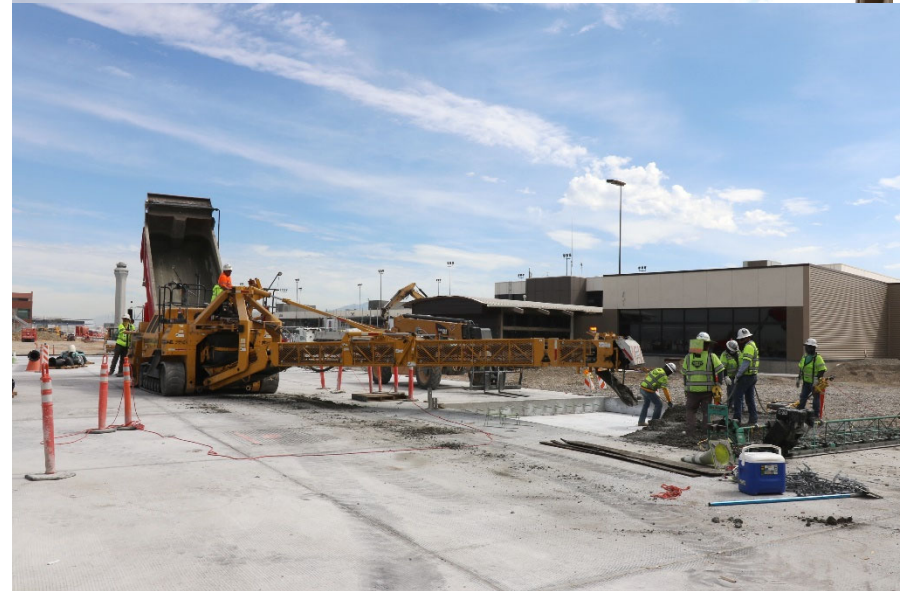
SCW North Apron Paving
