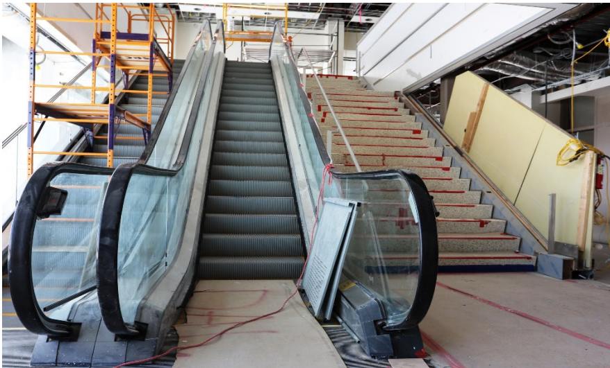
Sterile Corridor Level 2 to Level 3 Transition
