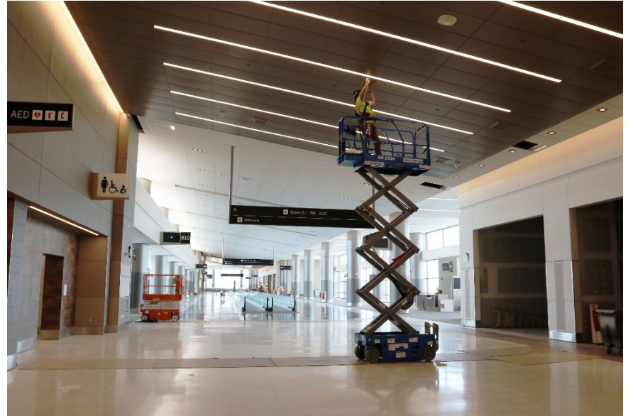
North Concourse Level 2 Passenger Node & west end
