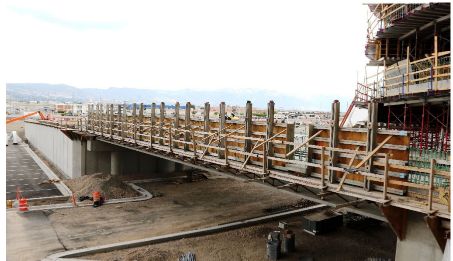
Garage East Entrance Barrier Wall
