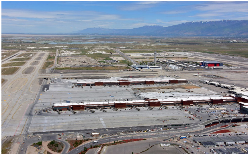
South & North Concourses looking north
