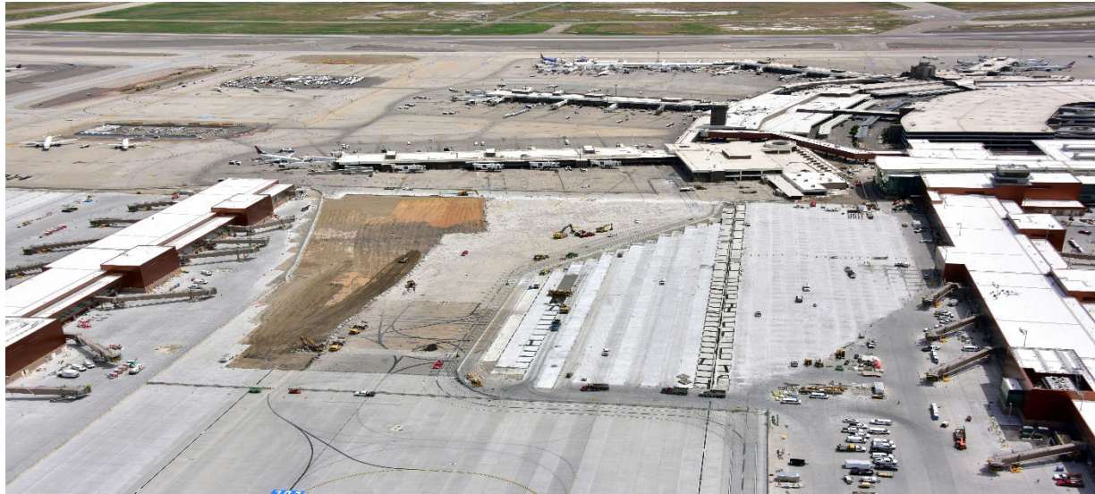
Future Taxilane 20 & 21 Paving looking east
