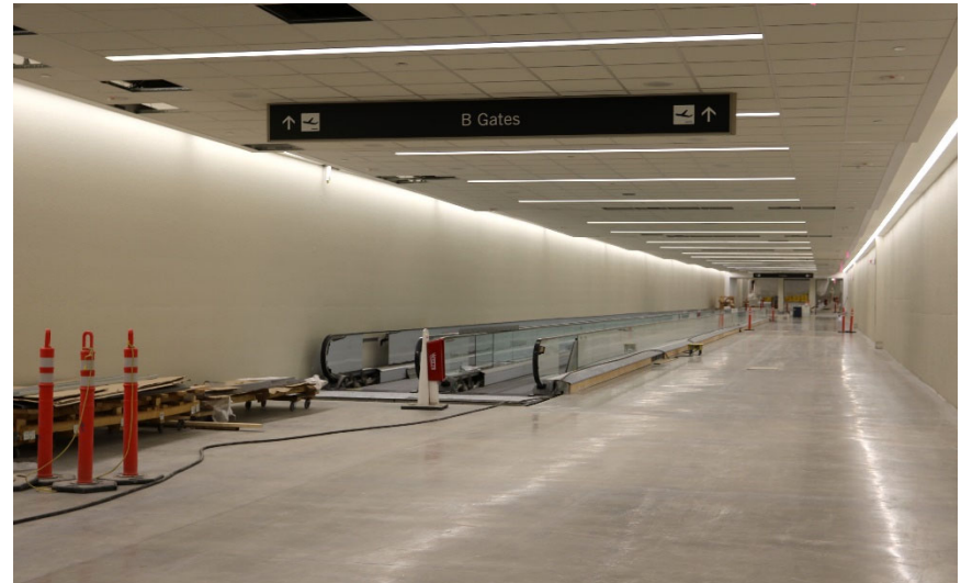
Mid-Concourse Tunnel Looking north
