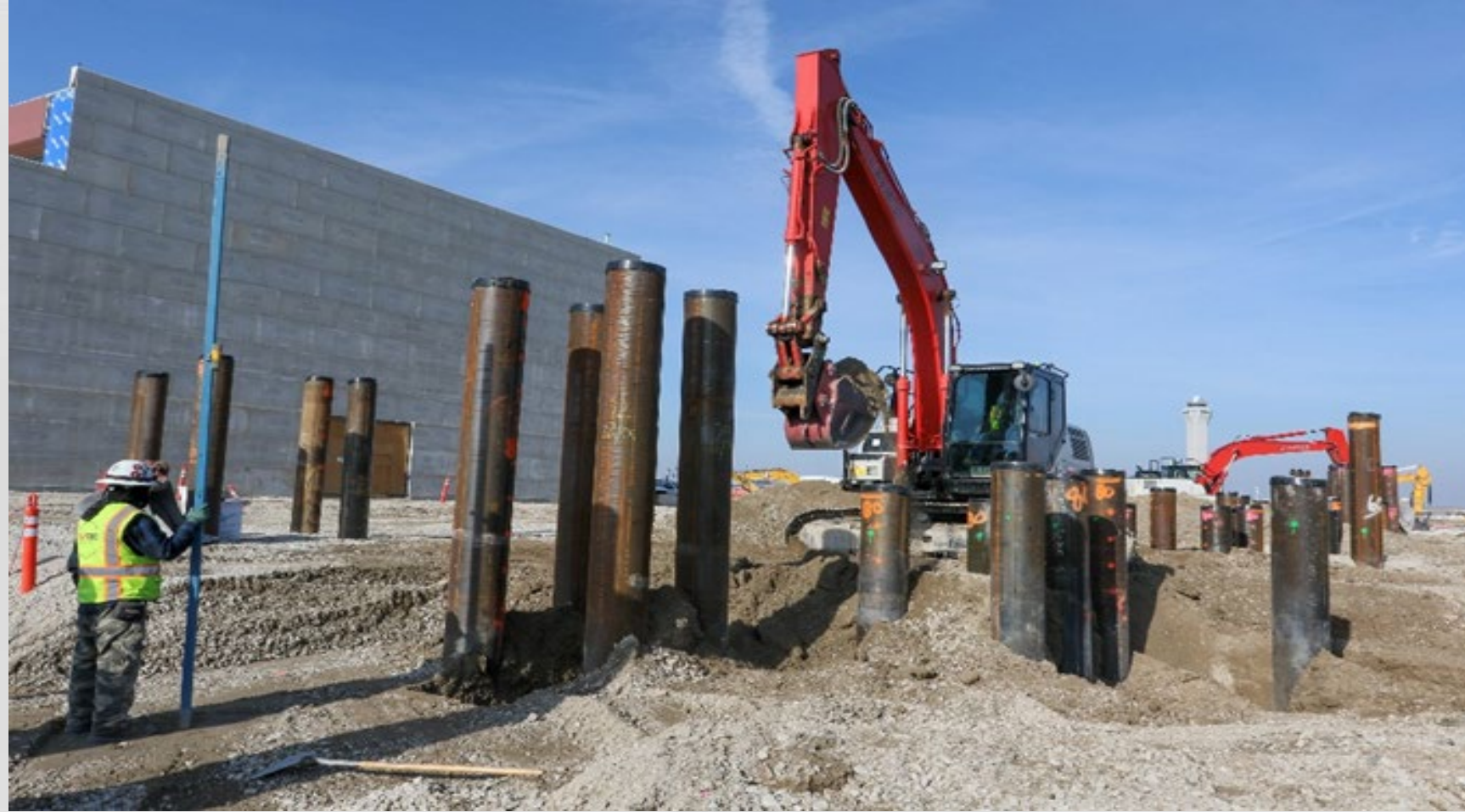
Pile Cap Excavation
