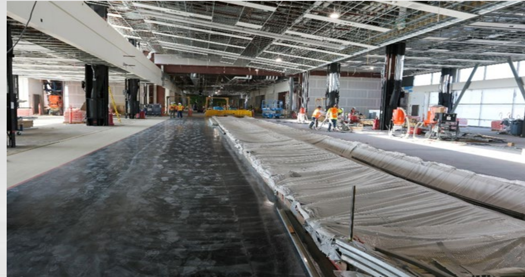
Level 2 Looking West
