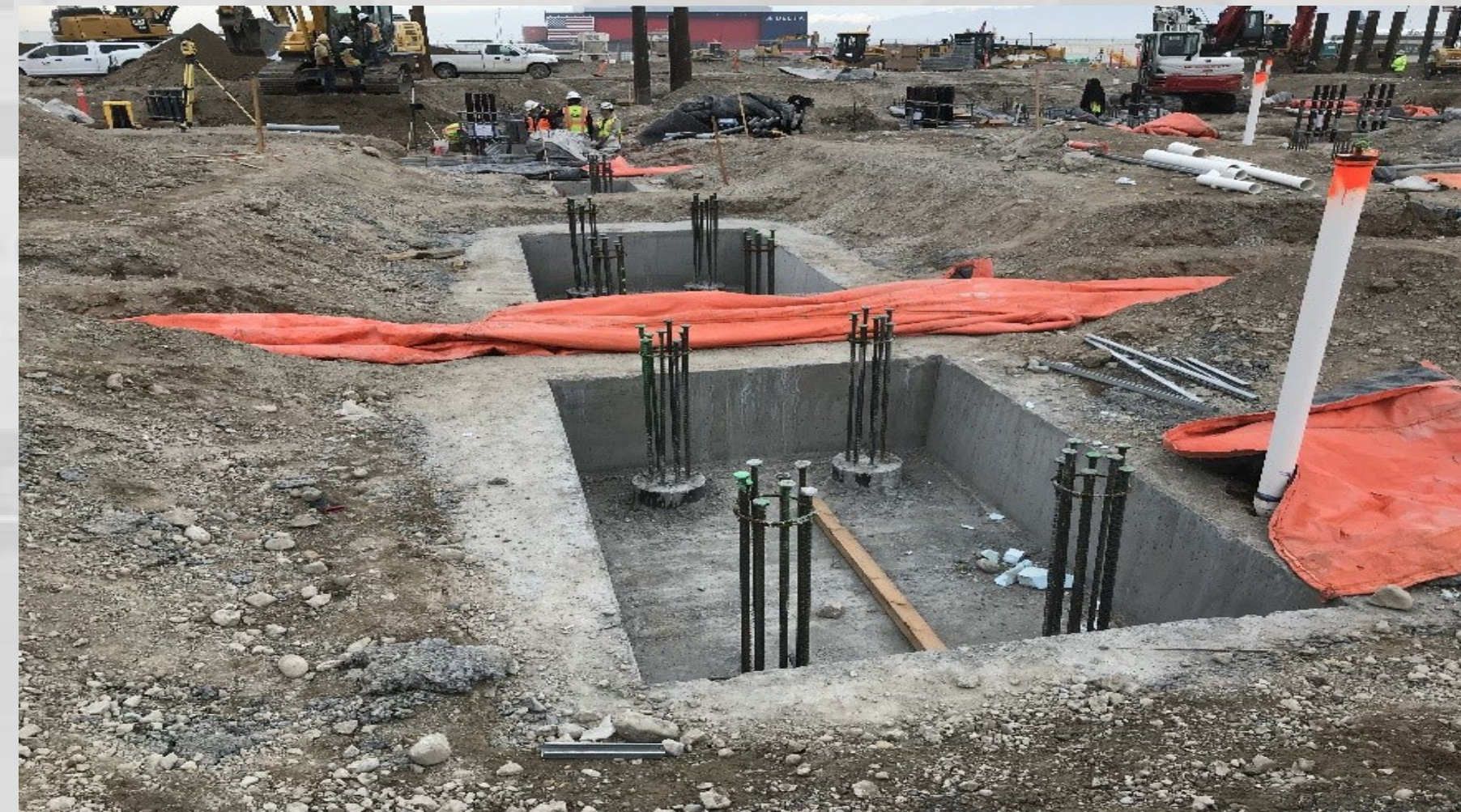
Start of Foundations
