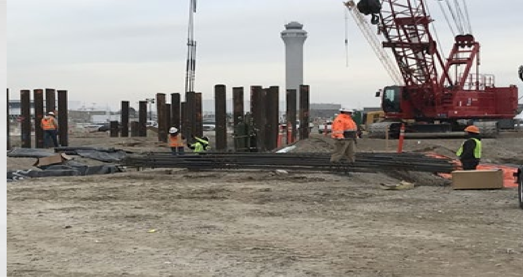
Pile Cut-off Underway
