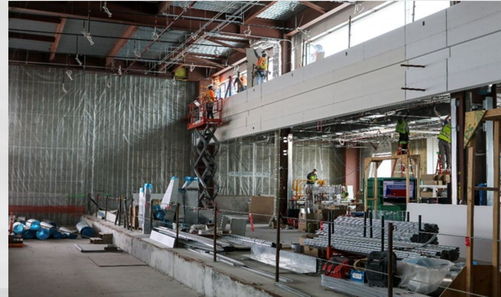
Level 2 Soffit Framing
