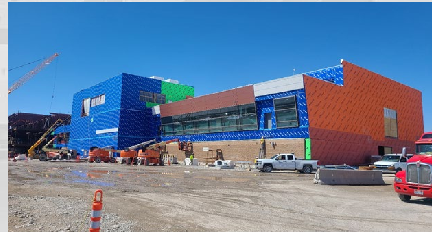
Exterior Metal Panel Installation
