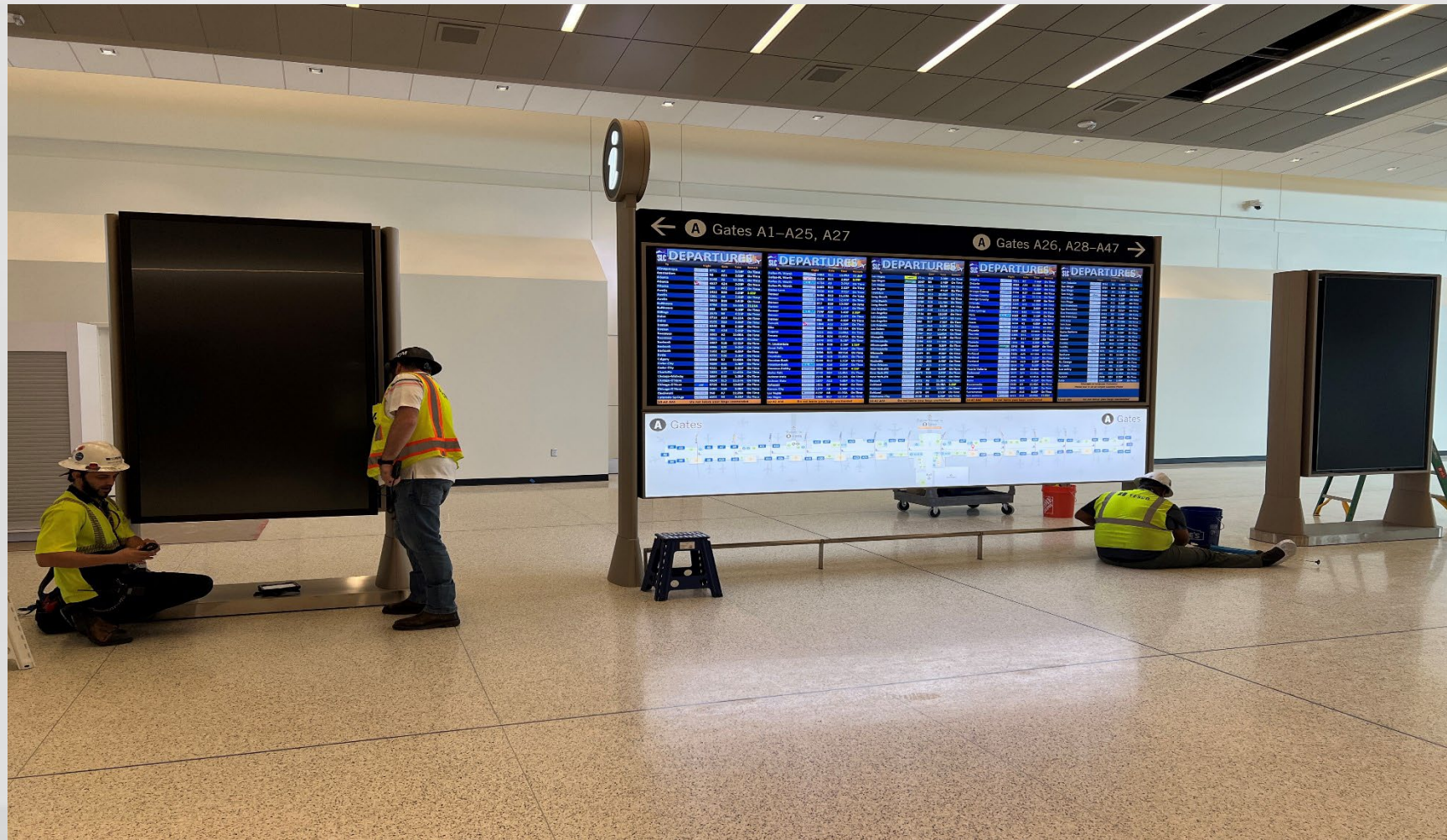
Info Hub Installation
