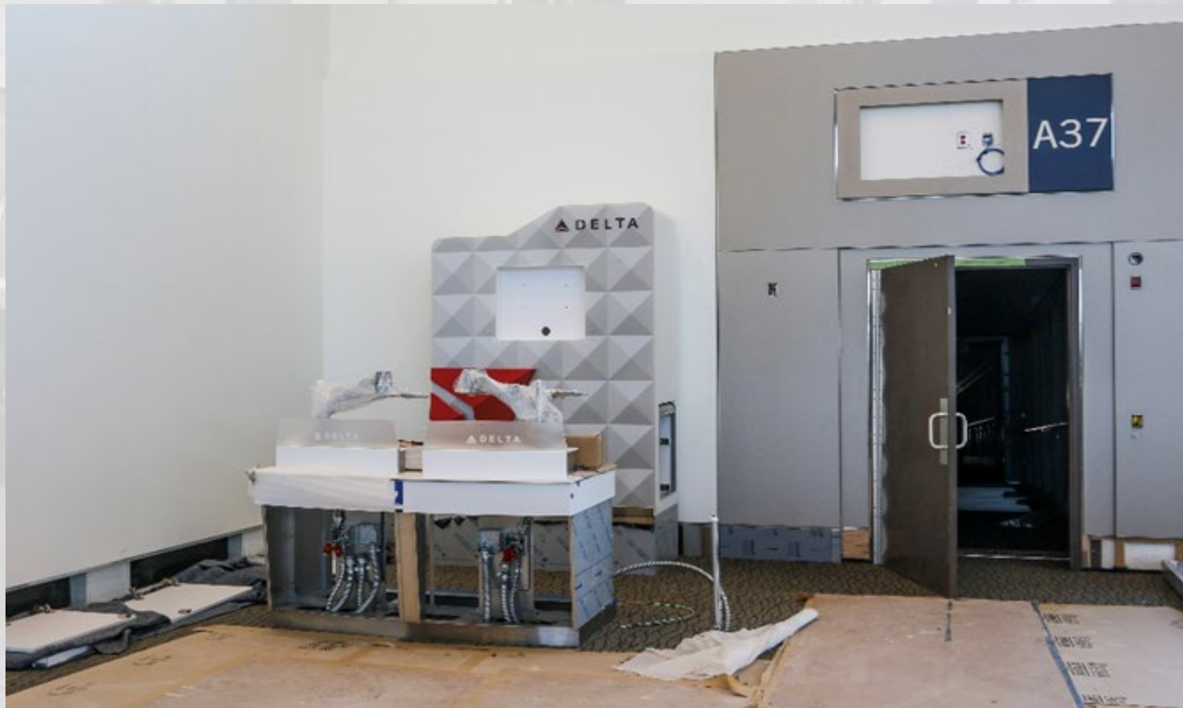
Area D Gate A37 Millwork Installation
