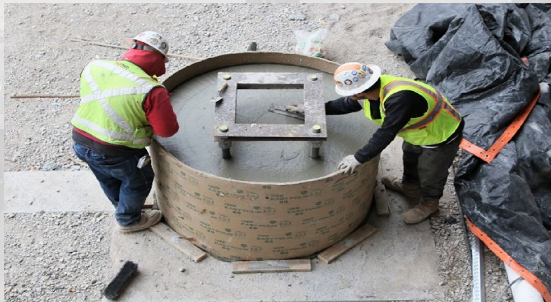
Passenger Boarding Bridge Foundation
