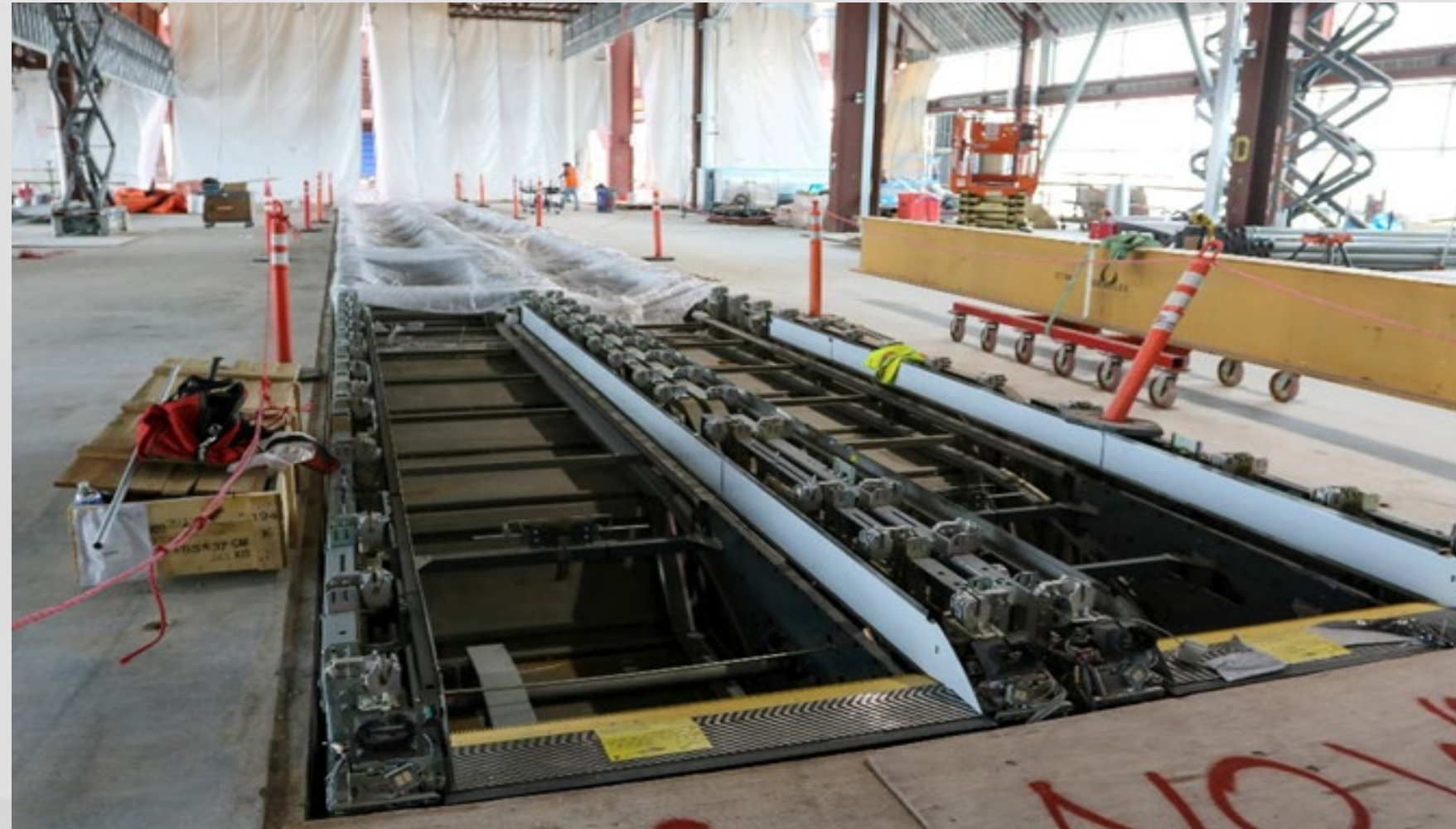
Level 2 Moving Walk Installation
