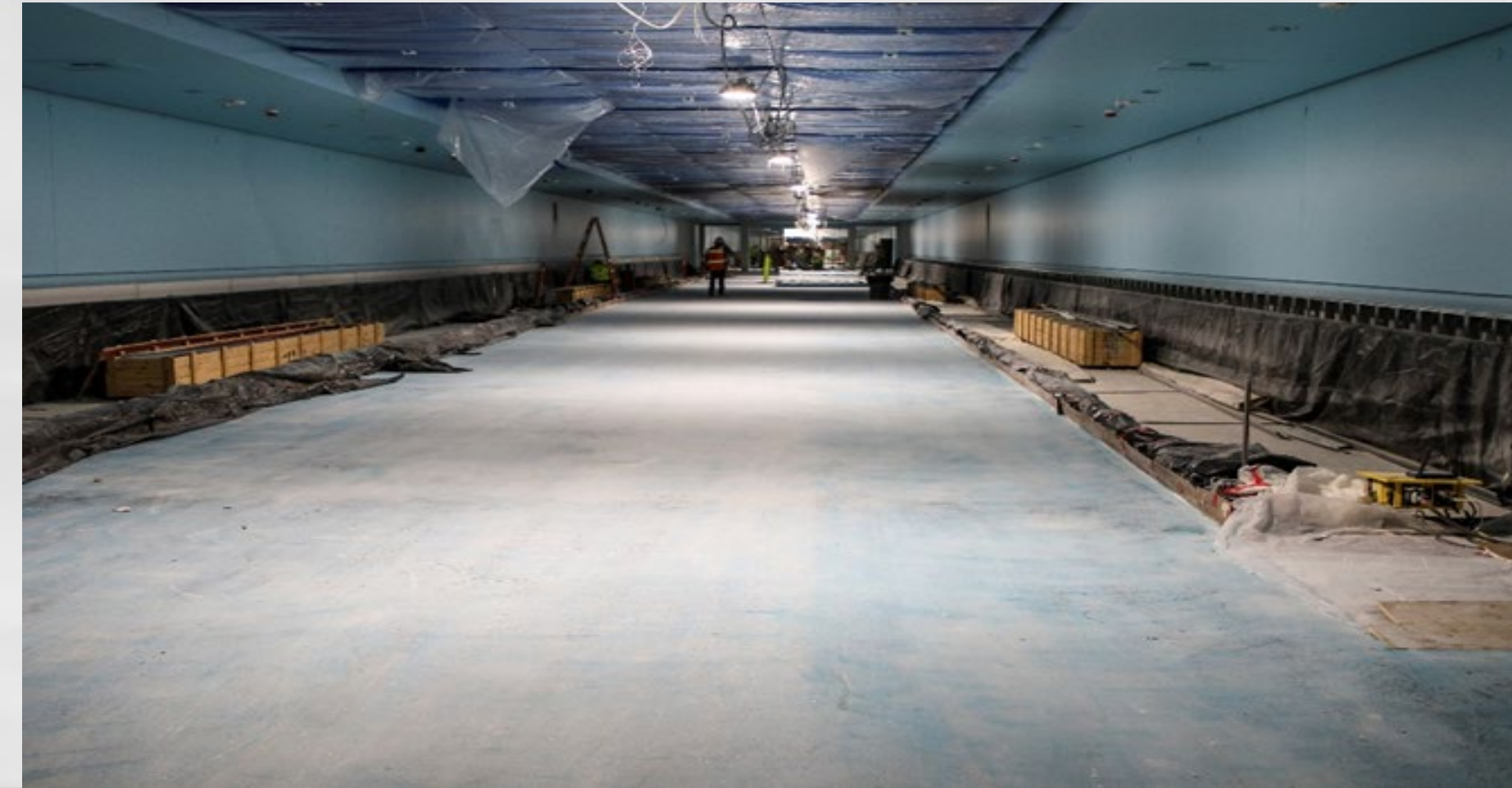
Terrazzo Rough Placement Complete
