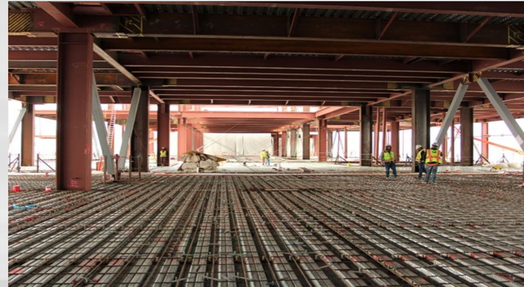
Central Node (Area G) Decking and Rebar
