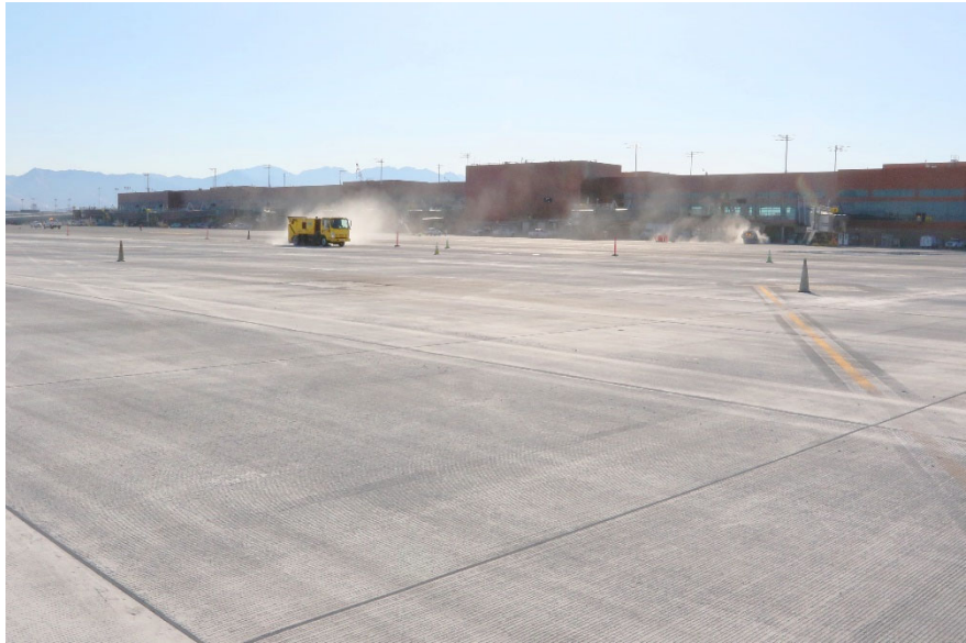
Final Sweeping of North Apron
