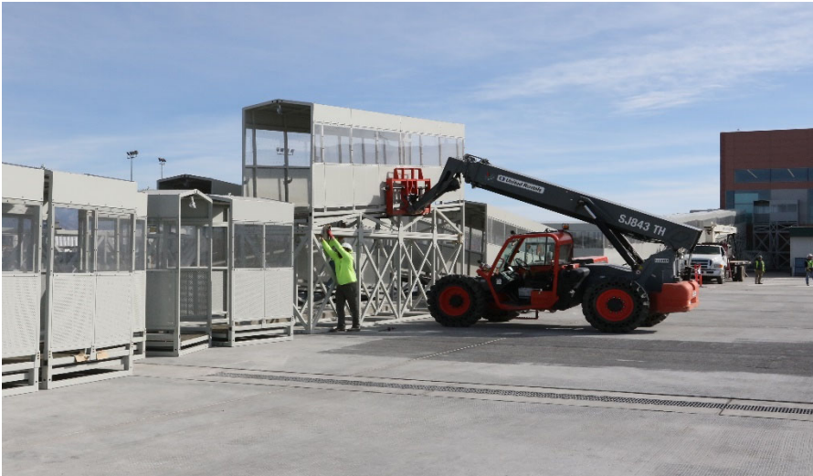
Bus Holdroom Passenger Ramp Installation
