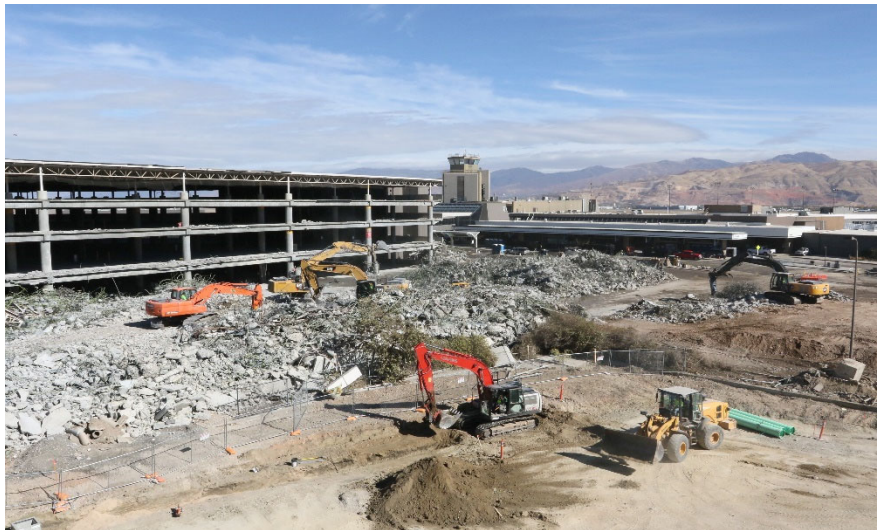
Parking Garage East Side Demolition
