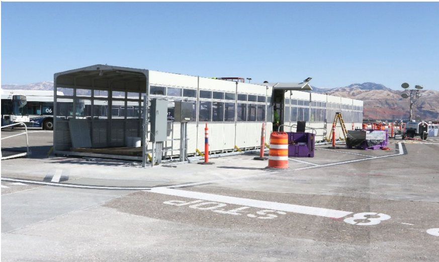
Hardstand Bus Shelters Installation
