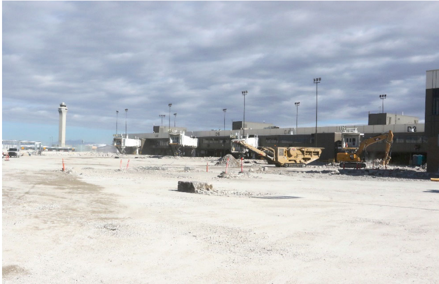
Concourse 'D' Jet Bridge & Pavement Demolition
