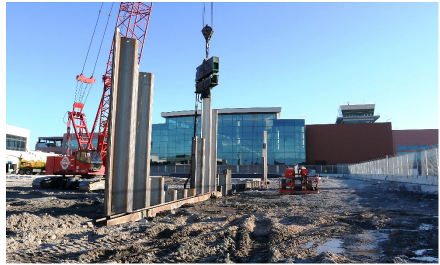
Central Tunnel Sheet Piles
