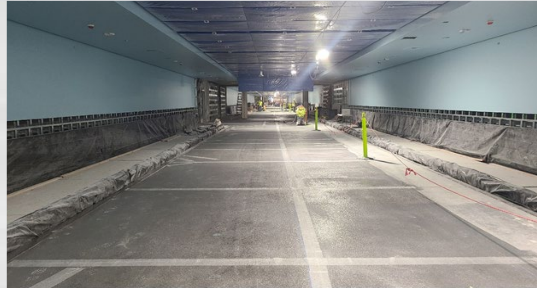
Terrazzo Floor Prep
