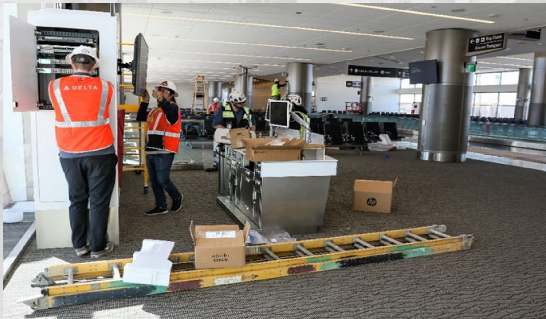
Delta IT Equipment Installation
