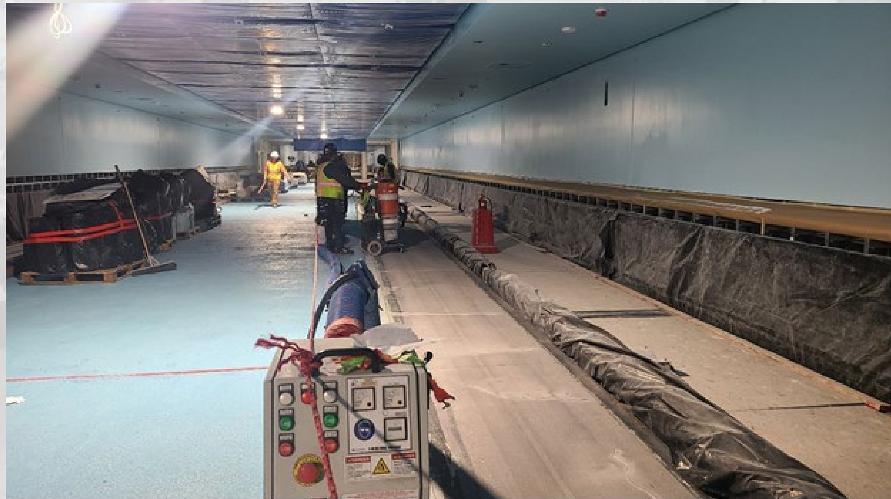
Central Tunnel Terrazzo Progress
