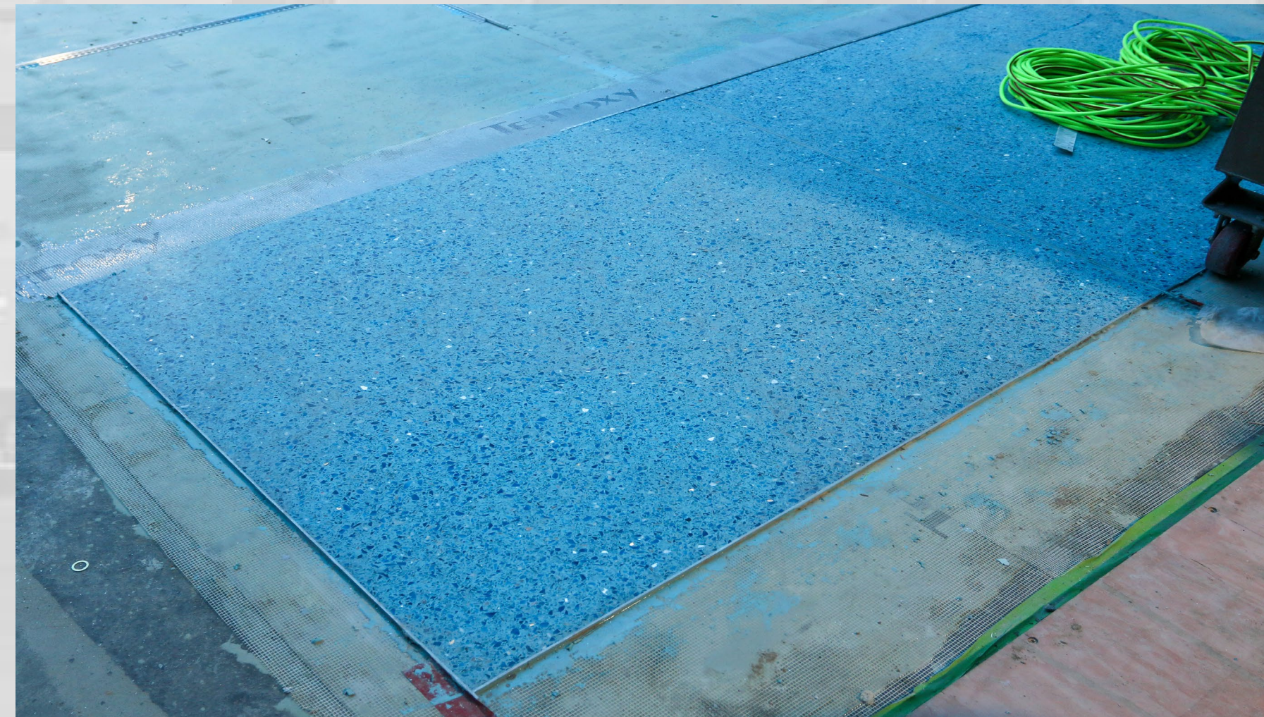
Terrazzo Floor Mock-up
