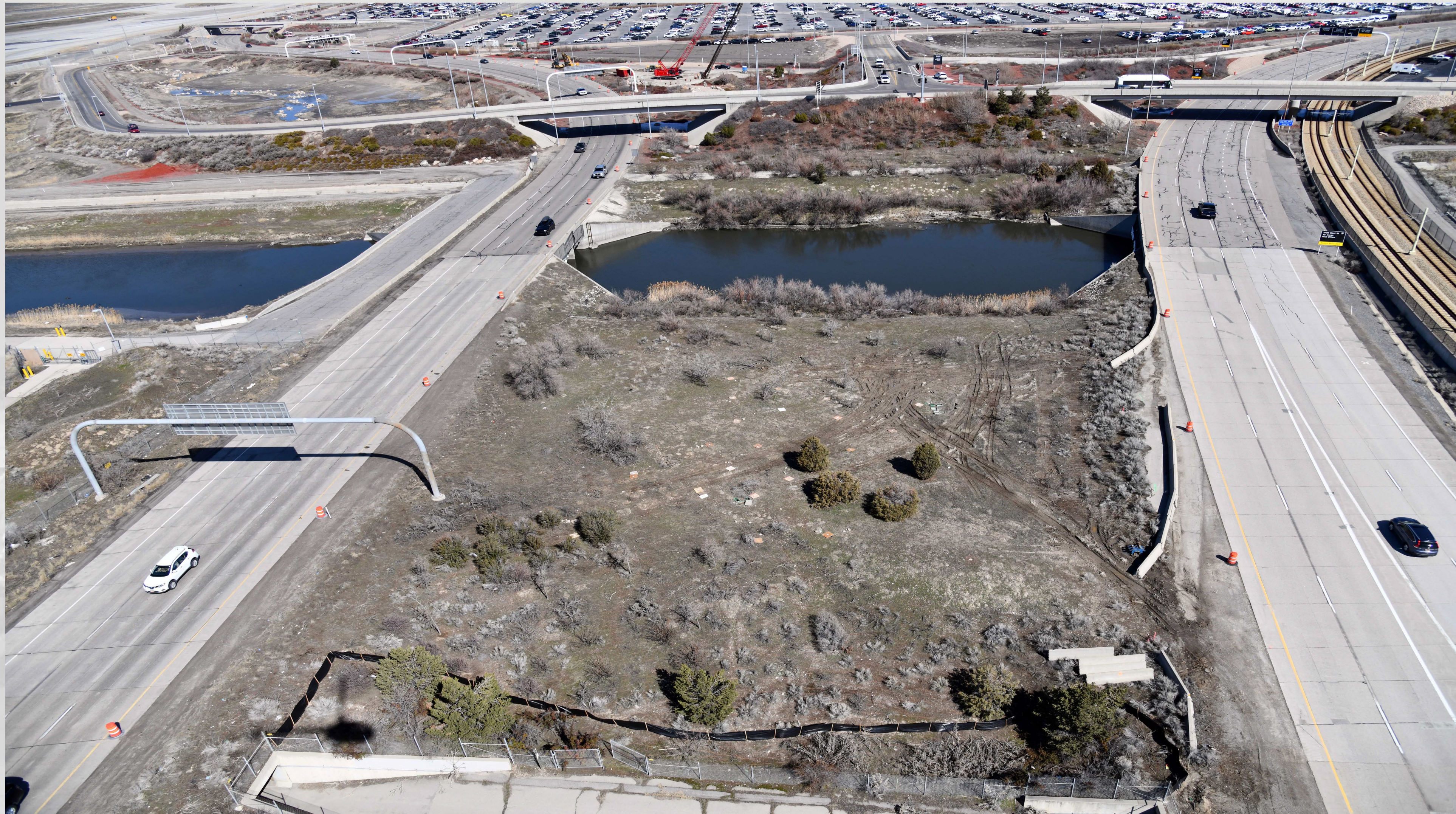
Entrance Installation Site
