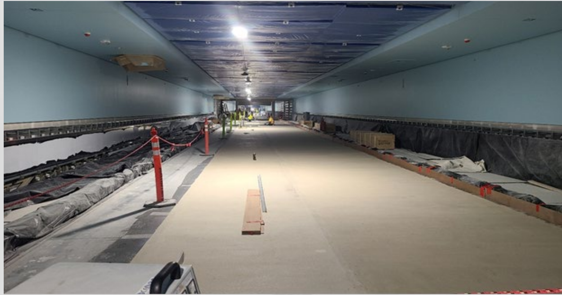
Central Tunnel Main Circulation Area
