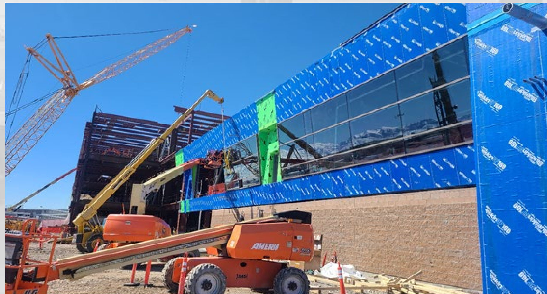
Passenger Boarding Door Framing
