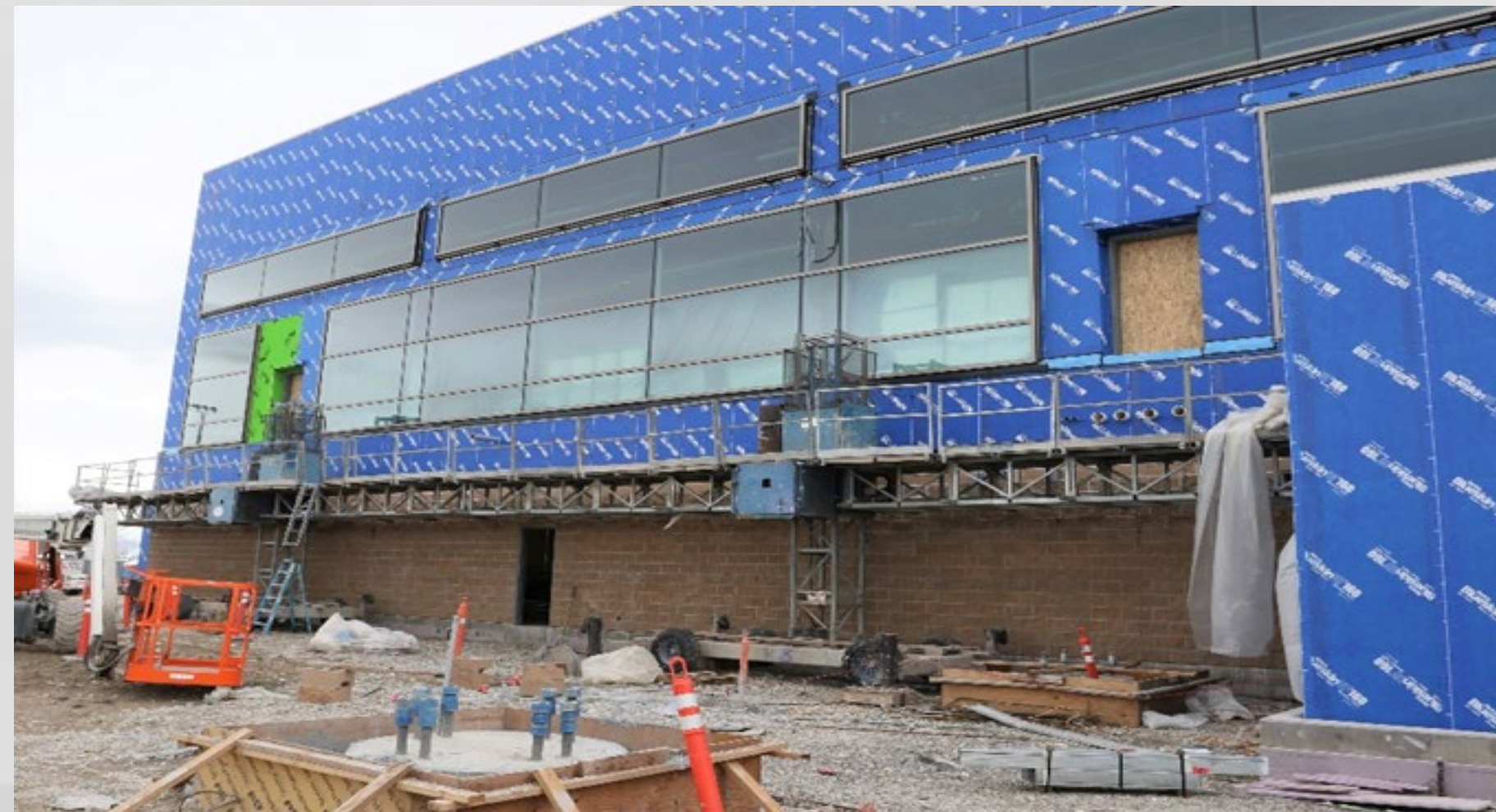
East End North Side Masonry and Glazing
