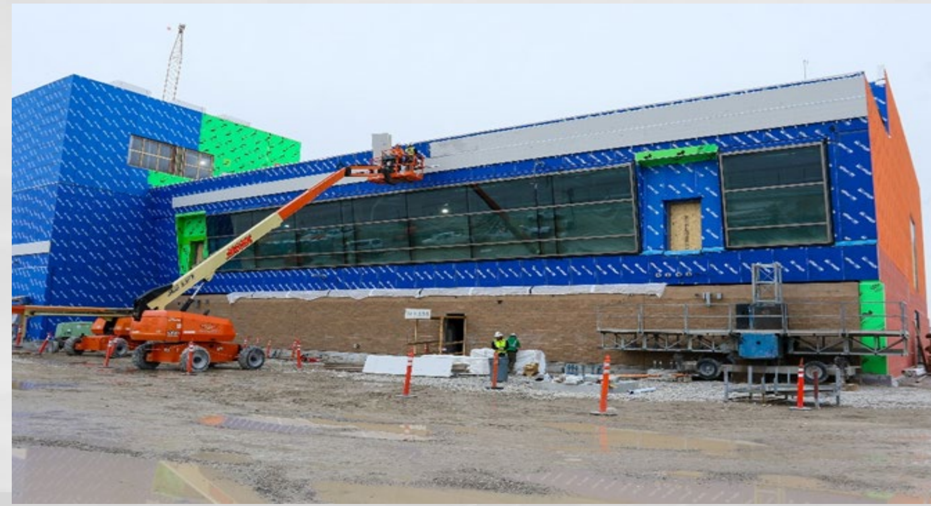
East End South Side Masonry and Glazing
