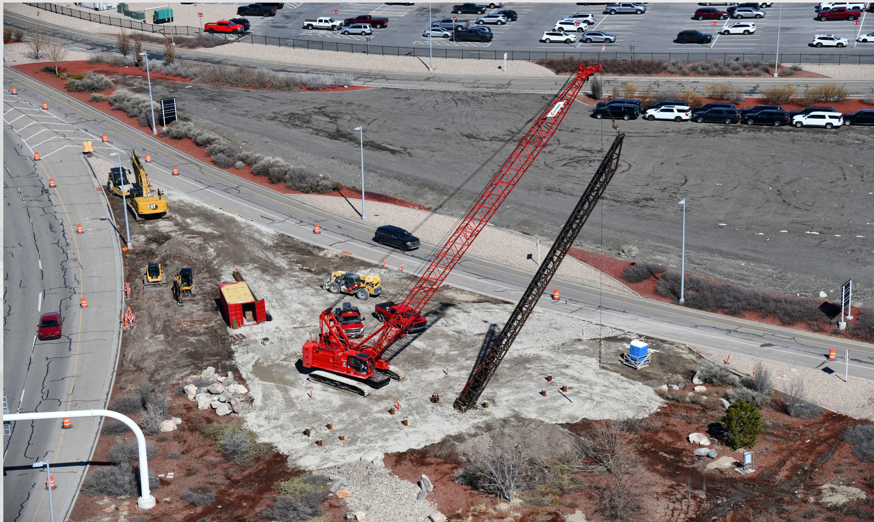
Exit Installation Pile Driving
