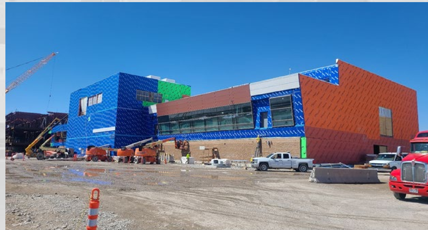
Start of Exterior Metal Panel Installation
