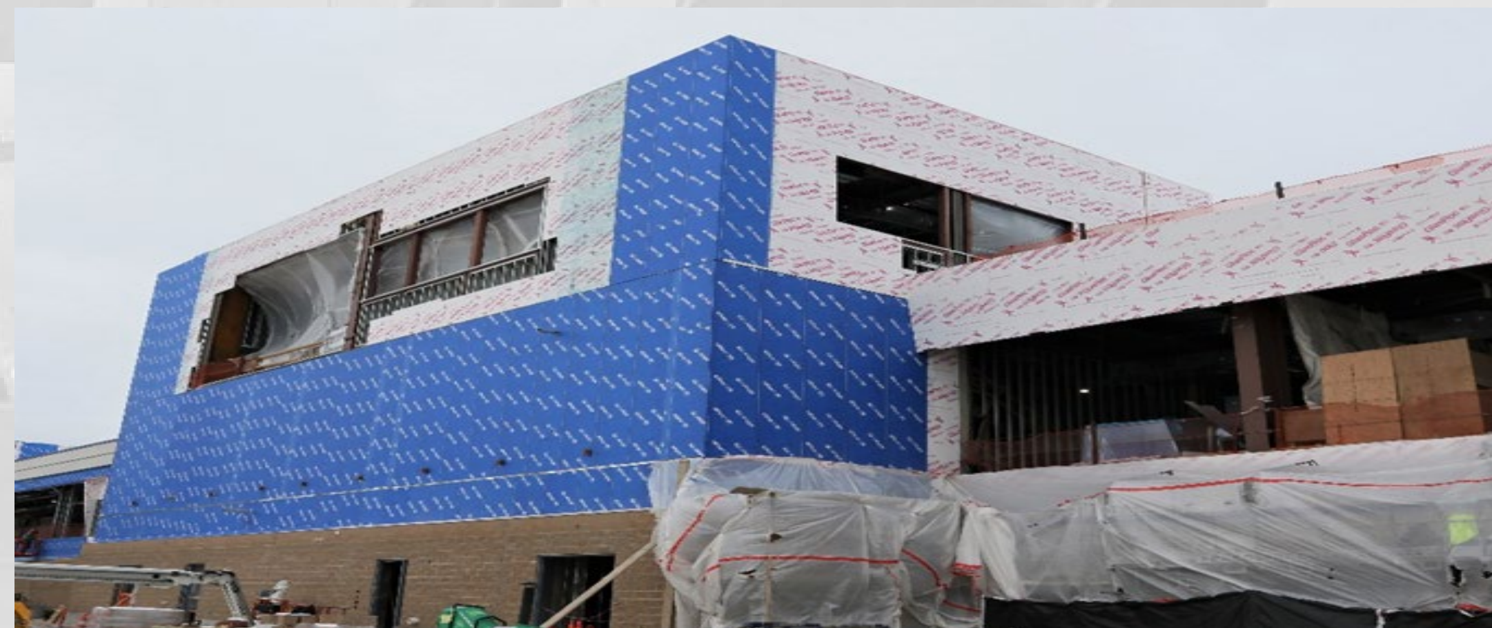
Area C Exterior Sheathing
