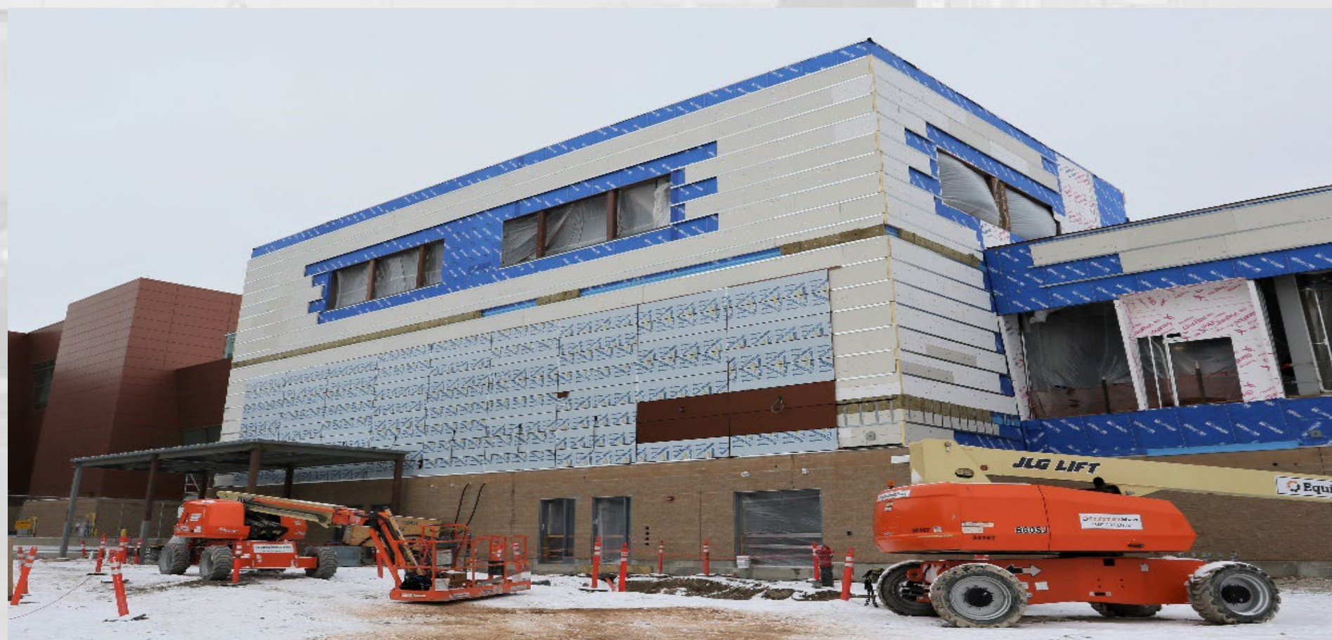
Area A Metal Panels South
