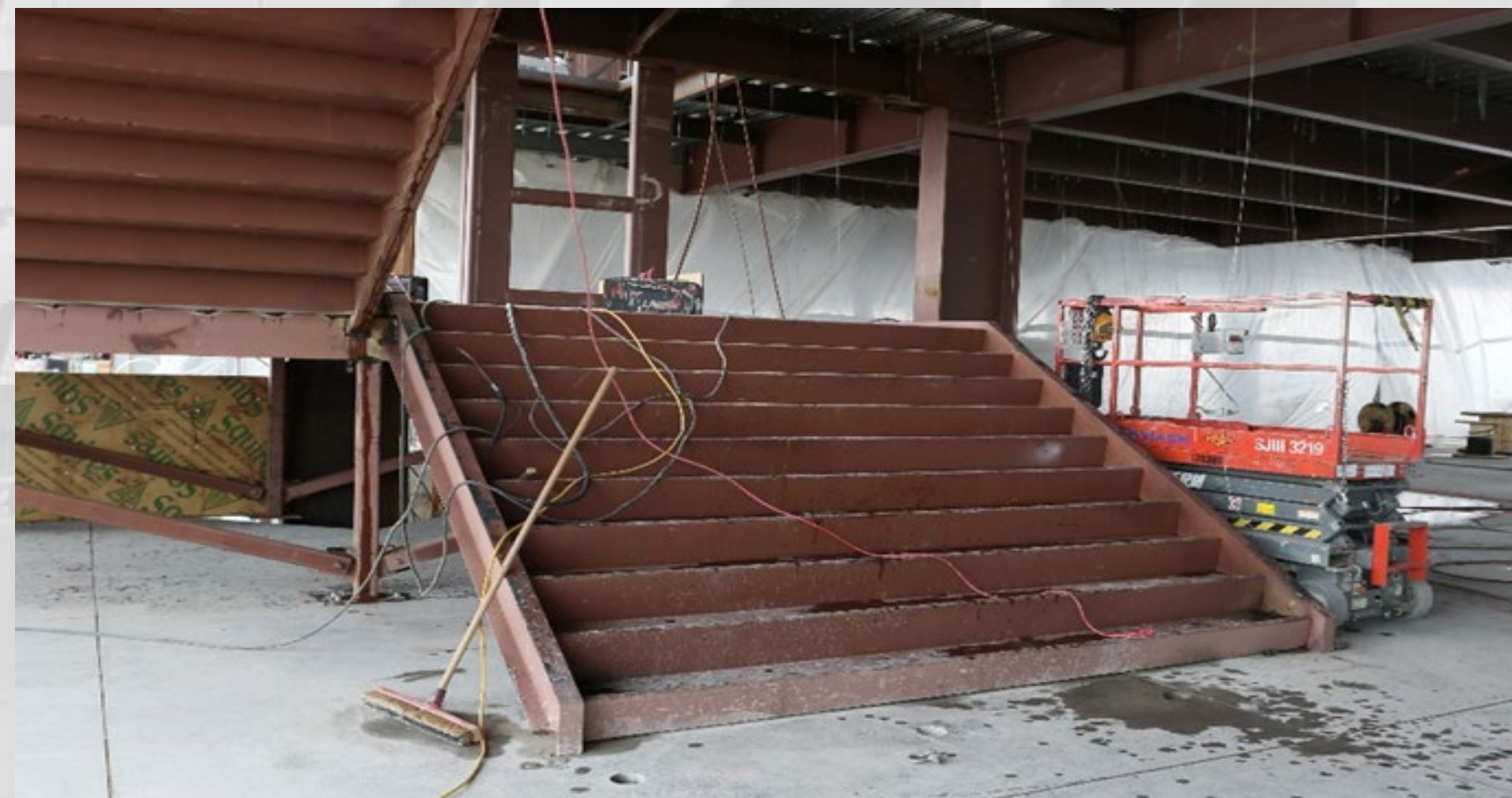
Area F (End of Building) Egress Stair
