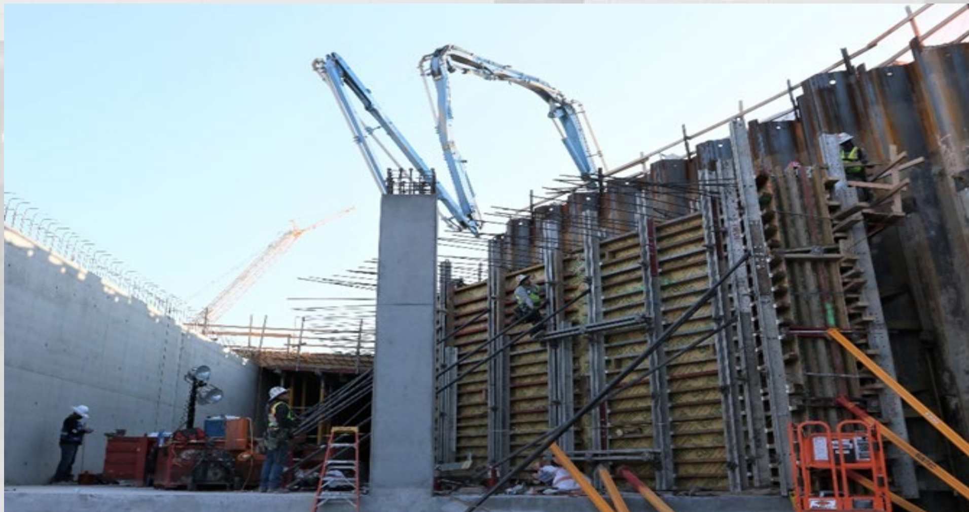
Wall Formwork
