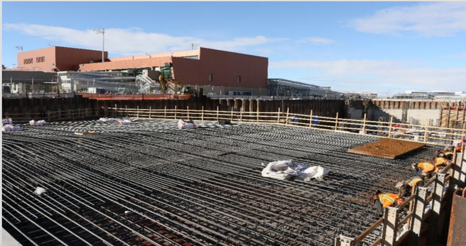
Lid Rebar and Formwork
