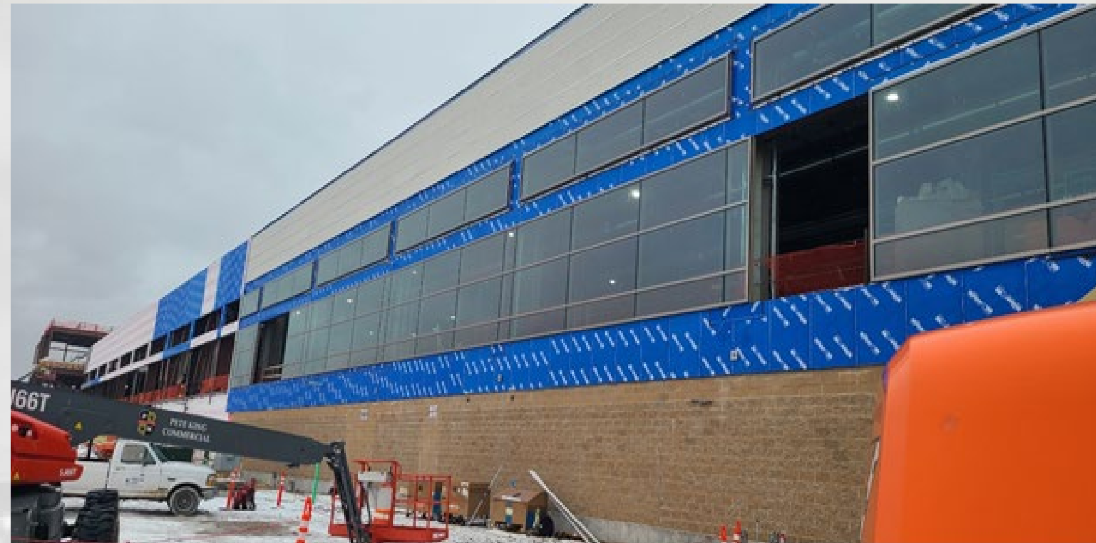
Area B Glazing north
