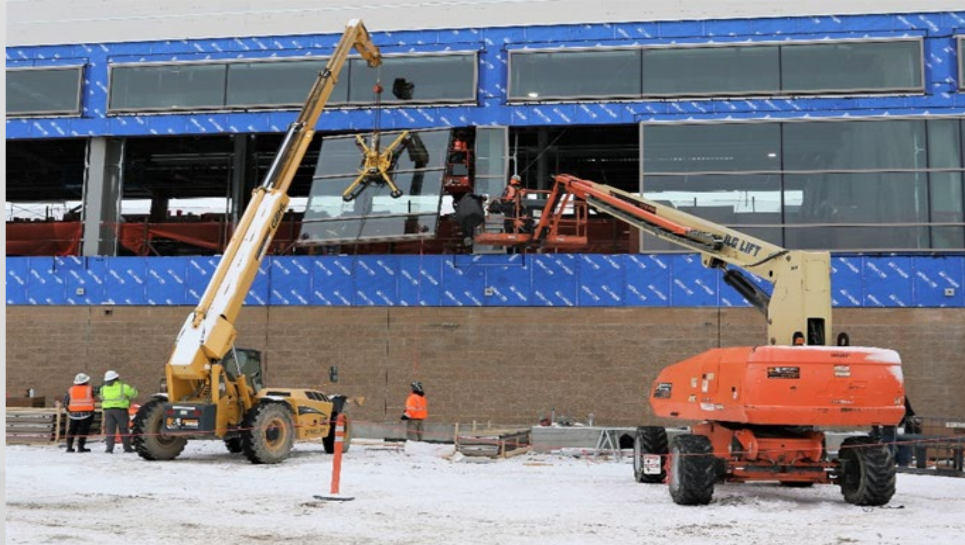
Area B Glazing north
