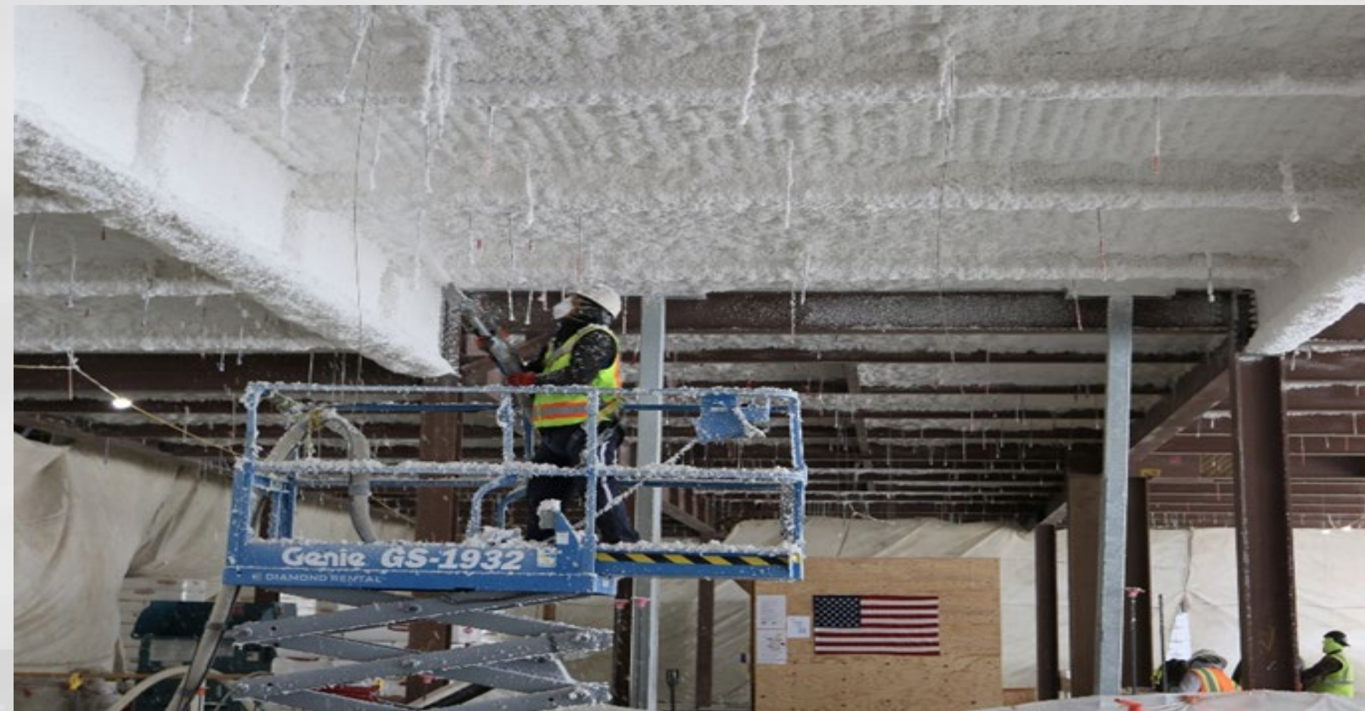
Area D Level 1 Spray Insulation
