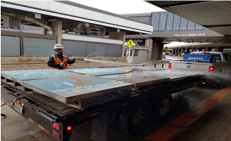
Loading Sections & Prep for Storage
