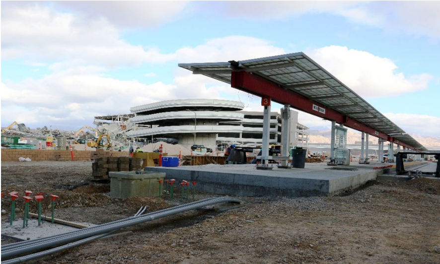
TRAX Station Looking East
