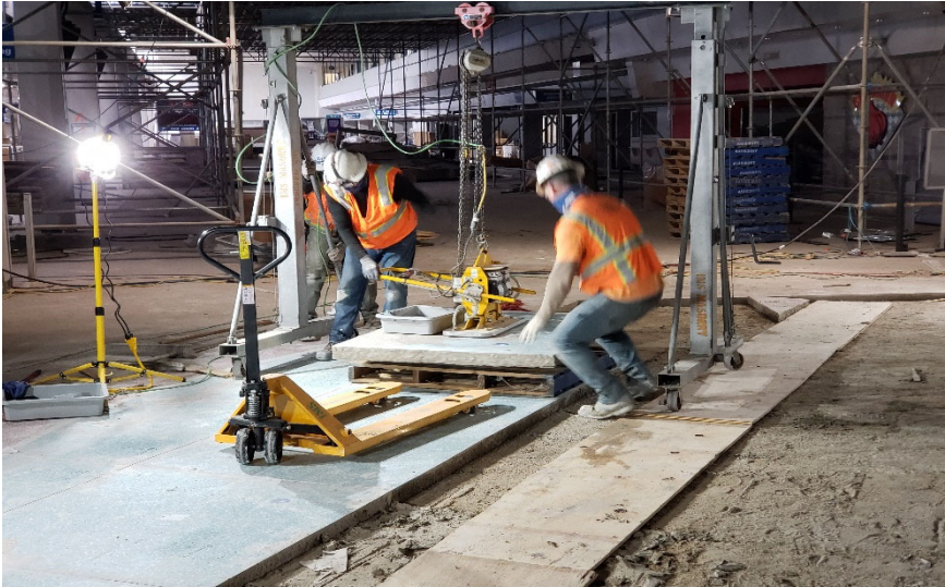
Hoisting out Sections
