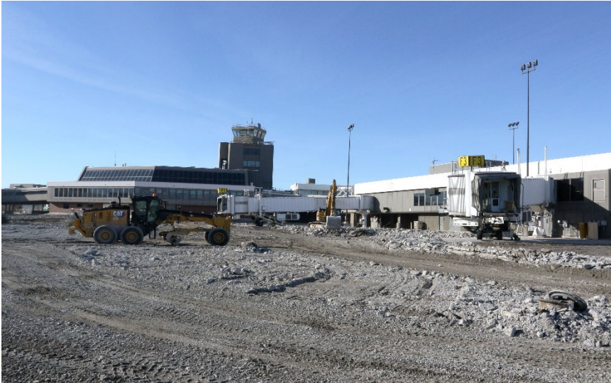
Concourse G Pavement Demolition
