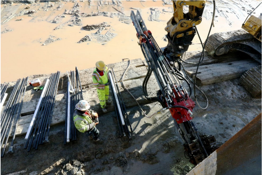
Installation of Central Tunnel Tie-backs
