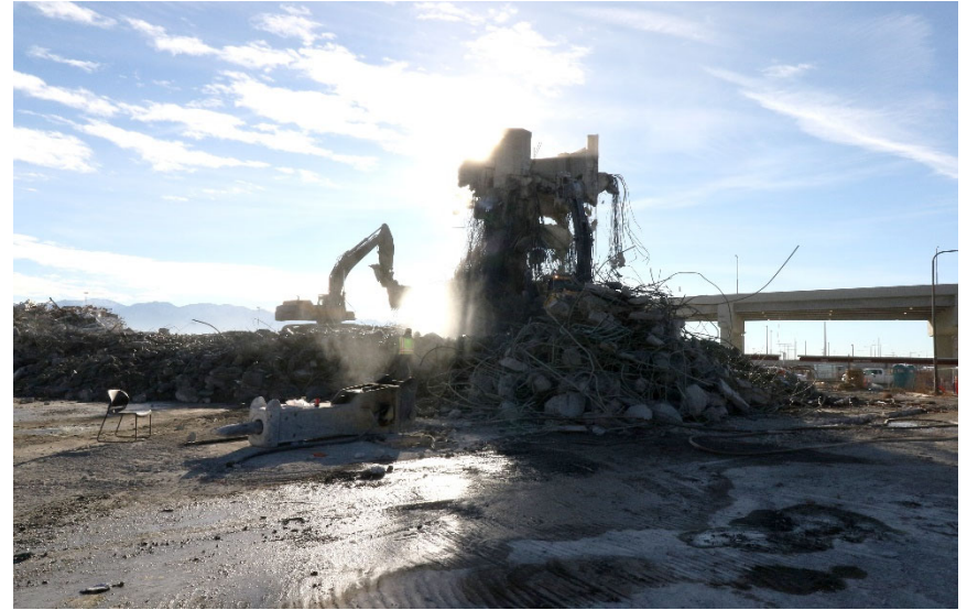
East Helix Demolition
