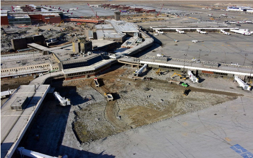
Concourse F & G Pavement Demolition
