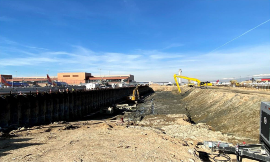
Tunnel Excavation Looking North
