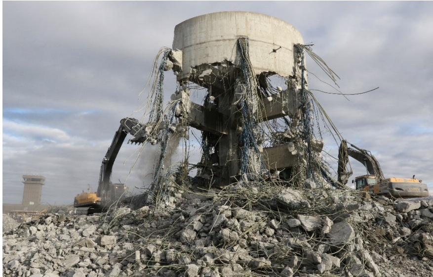
East Helix Demolition
