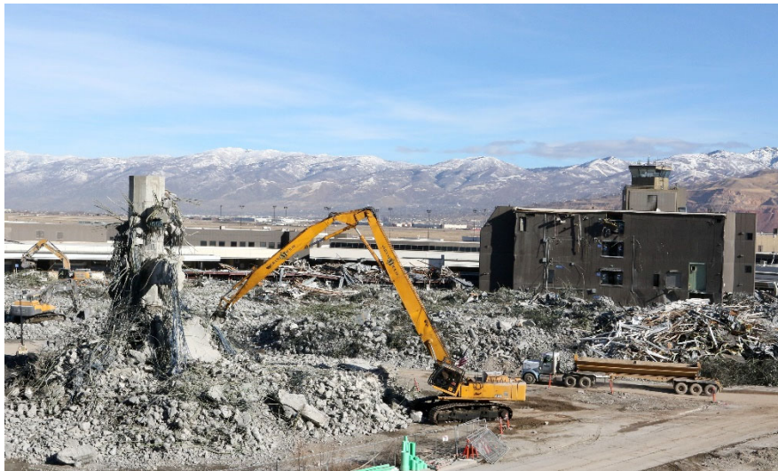
Parking Garage Demolition Looking Northeast
