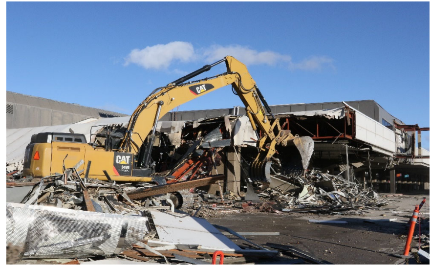
Start of T2 Demolition
