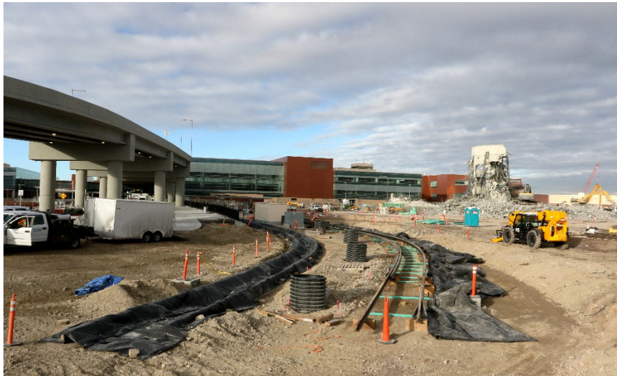
TRAX Track Installation
