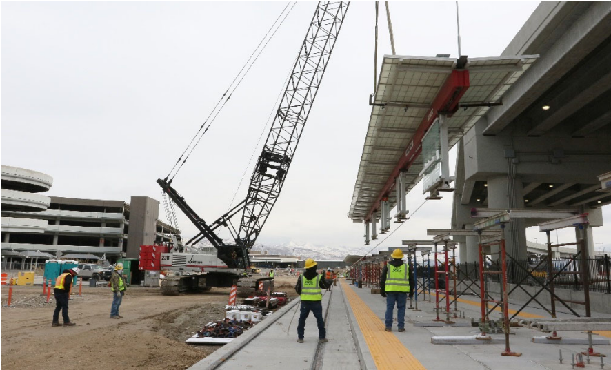
Moving Old TRAX Platform Canopy into New Station
