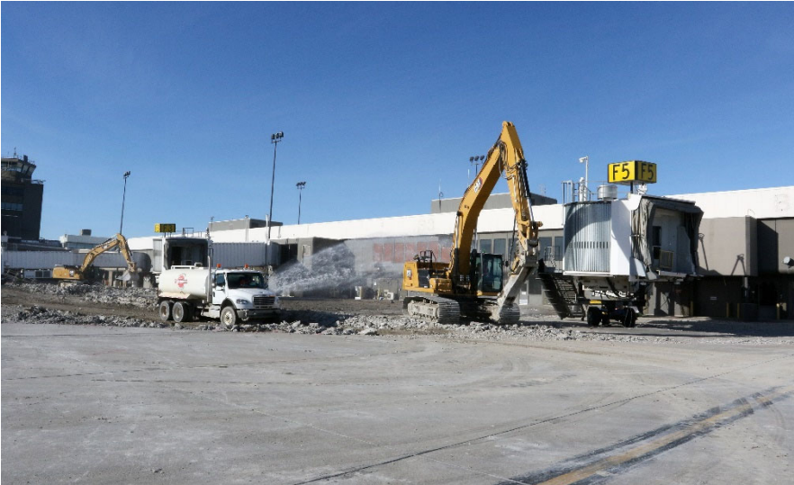
Concourse G Pavement Demolition
