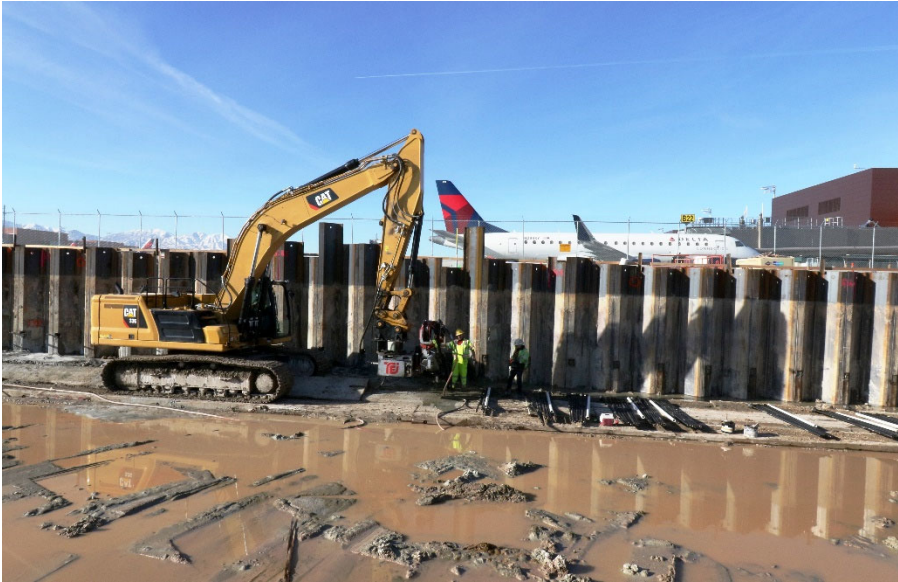
Central Tunnel Excavation Looking West
