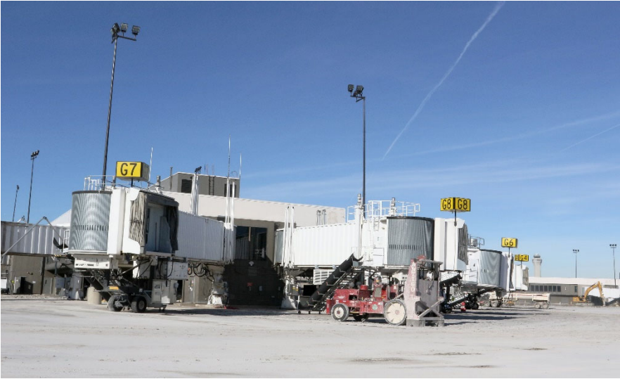
Concourse G Ready for Demolition
