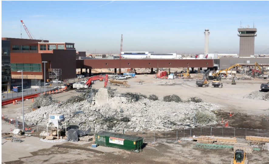
Garage Demolition Rubble
