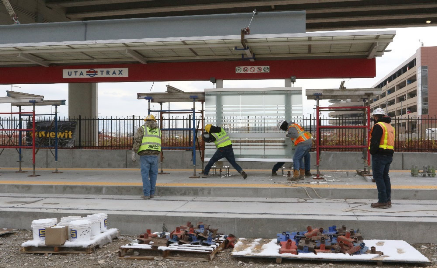
TRAX Platform Canopy Installation
