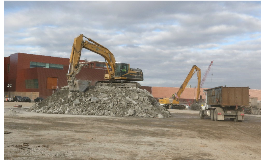
Demolition Rubble Haul-off
