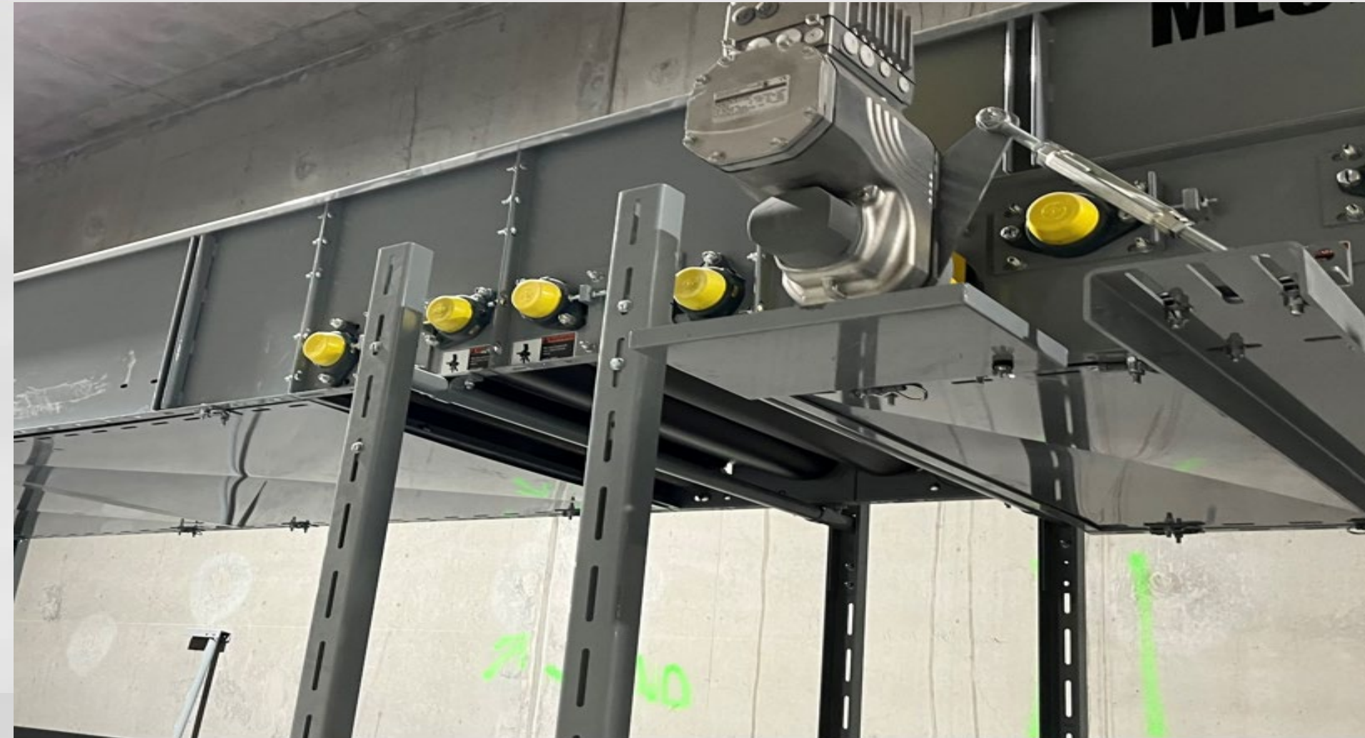
Baggage Conveyor Motor Installation
