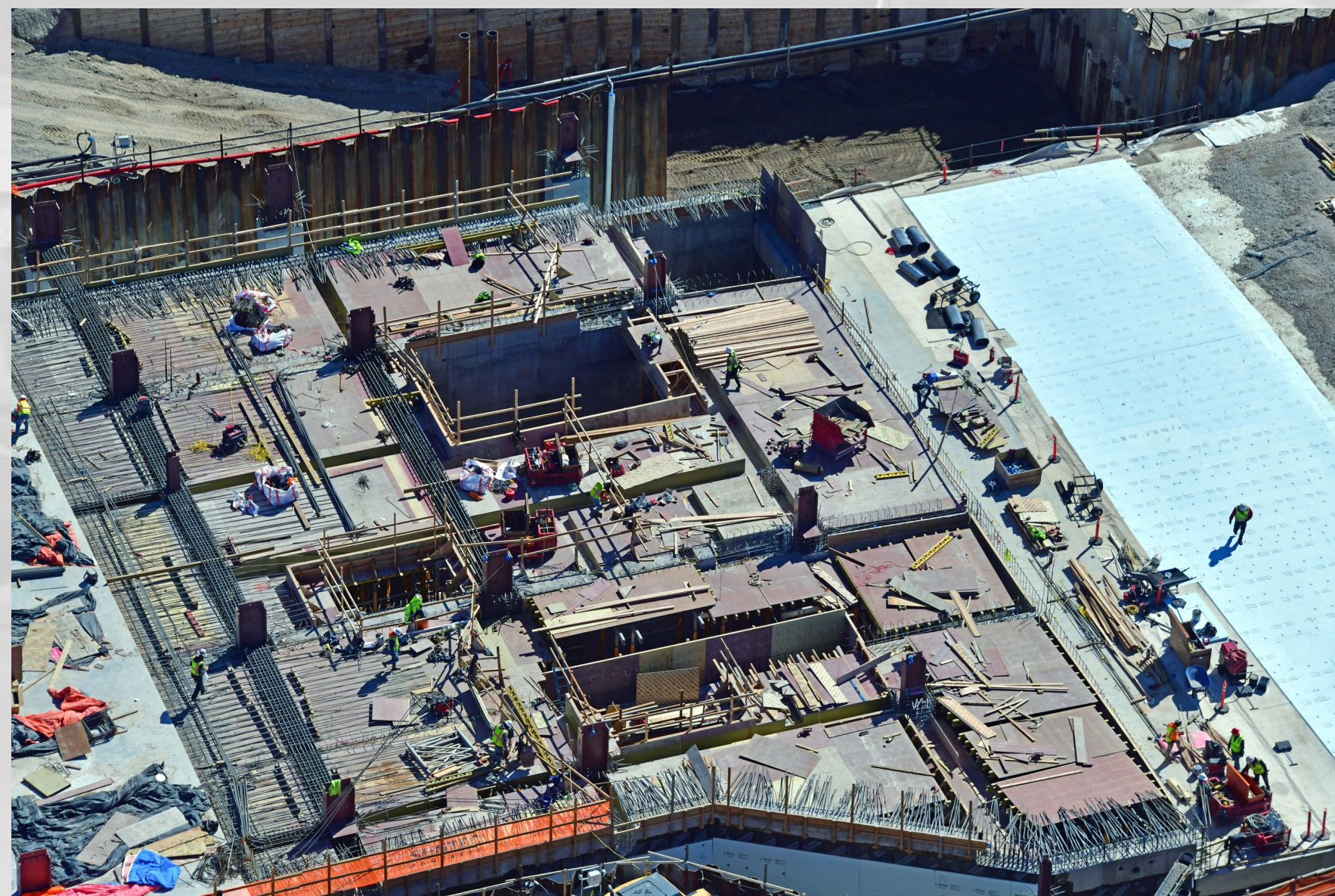
Area G Node - Tunnel and Basement
