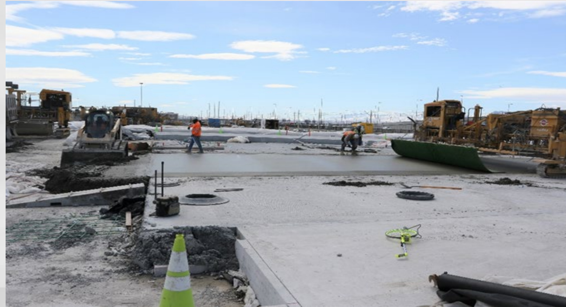
Airfield P-501 Paving
