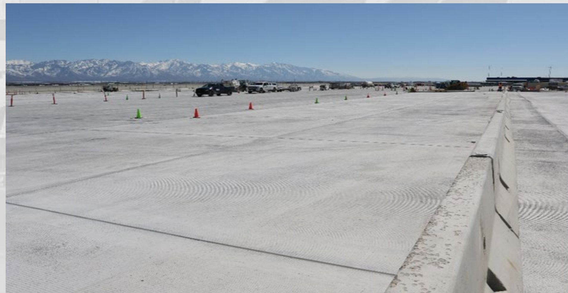
Taxiway 'Y' Paving Looking South
