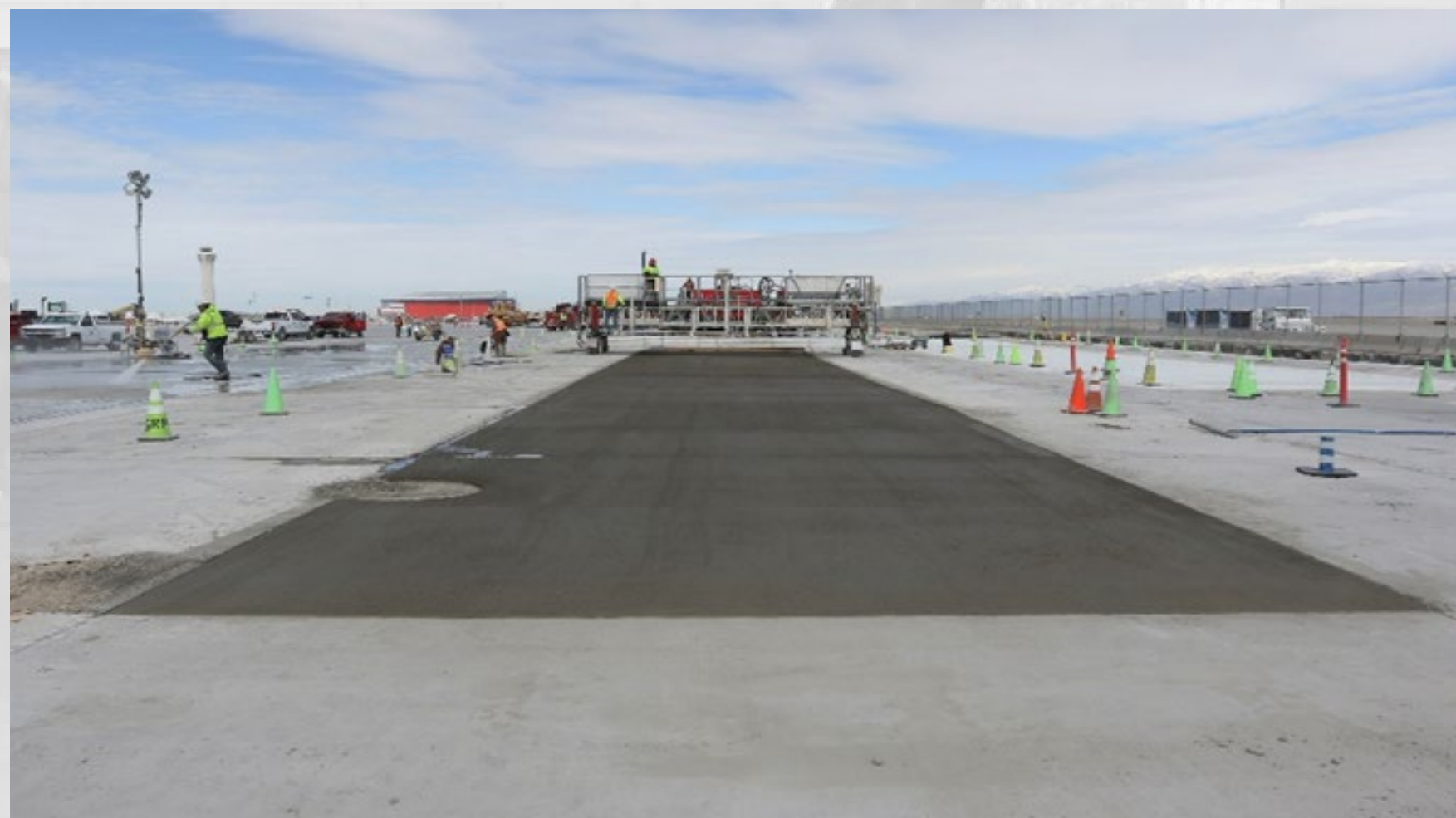
Taxiway 'Y' Paving Looking North
