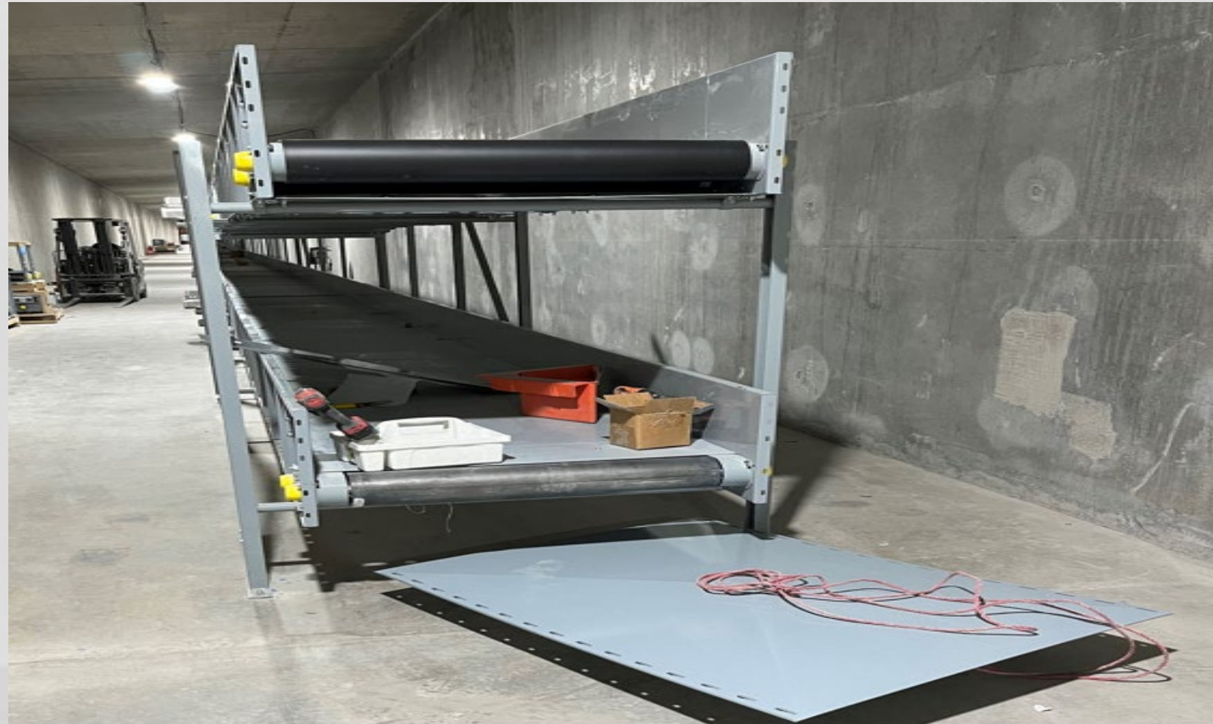
Baggage Conveyor Belt Installation
