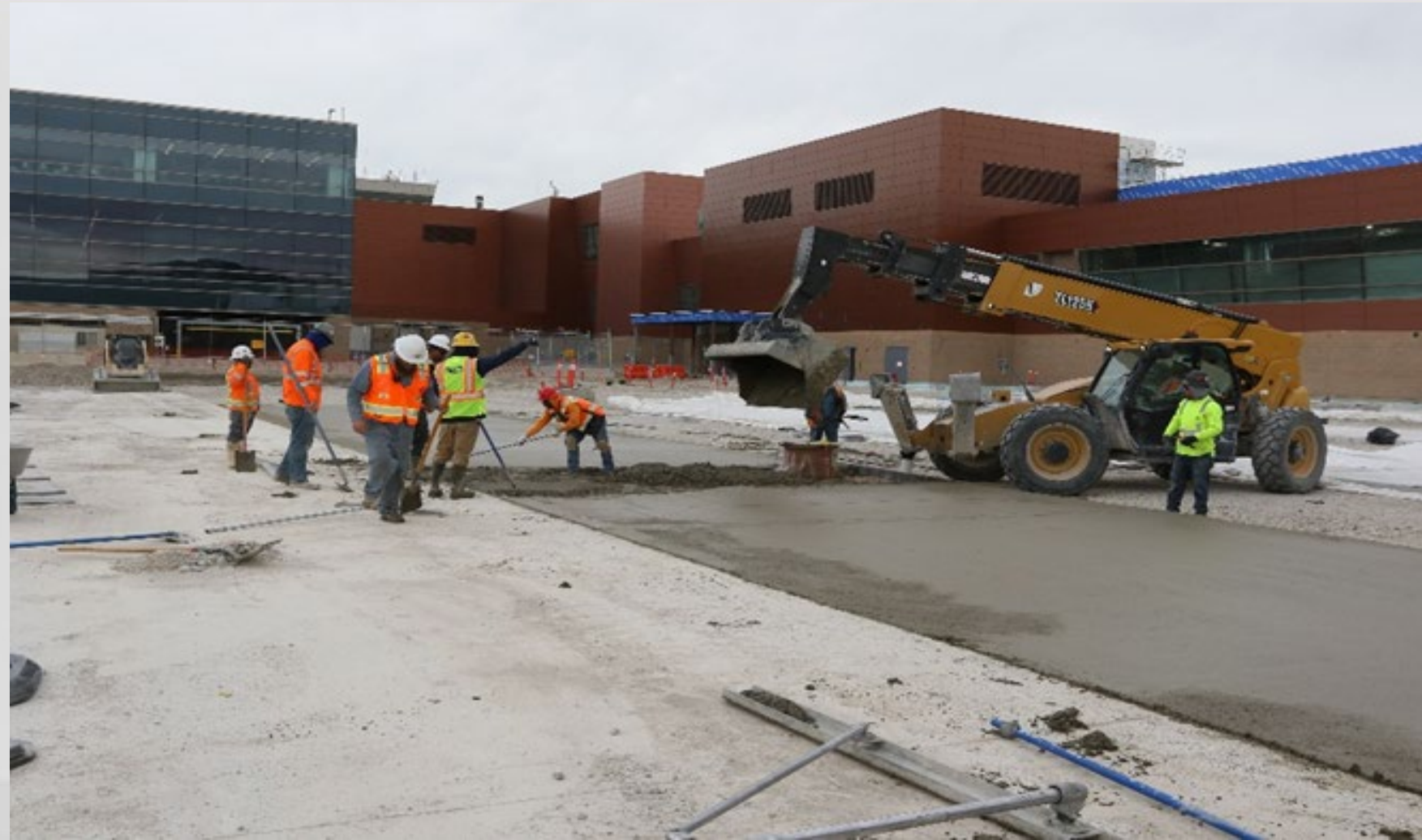
Lean Concrete South Side of Concourse 'A'
