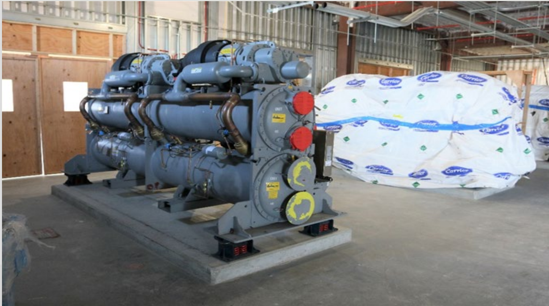
Level 1 Area C PCAir Chiller Installation
