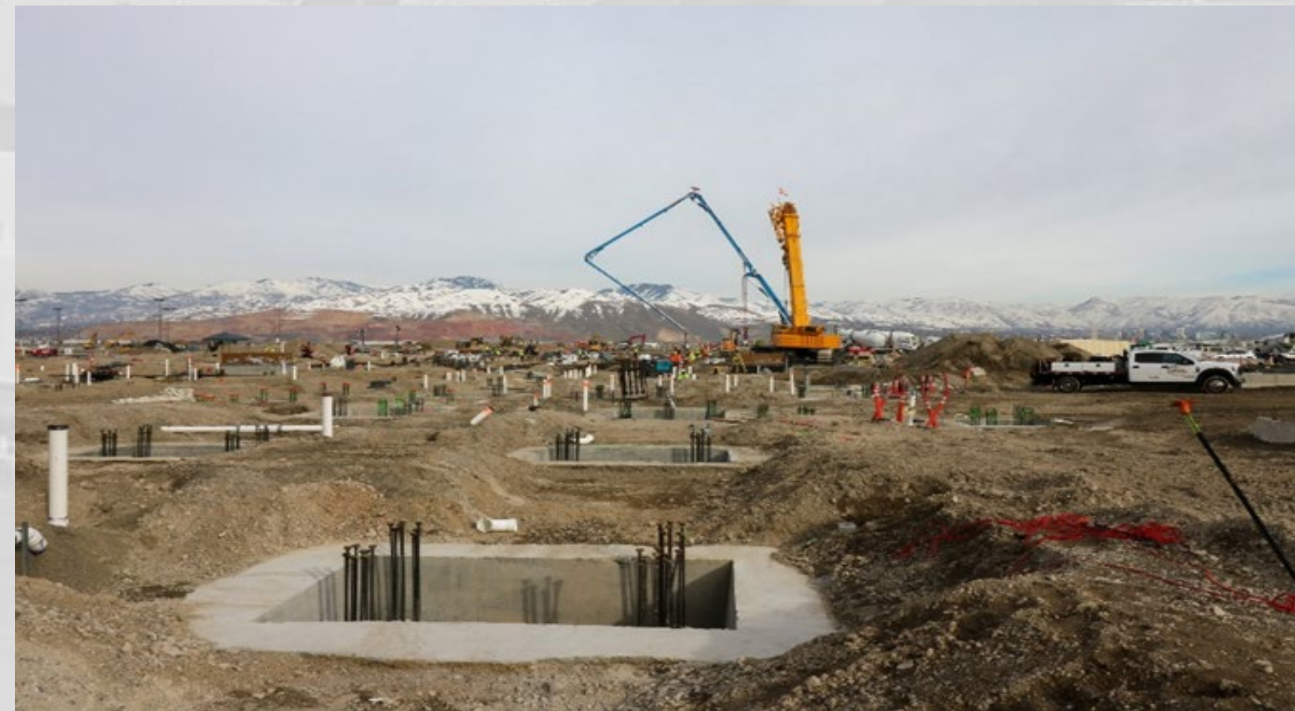
Building Pad Backfill
