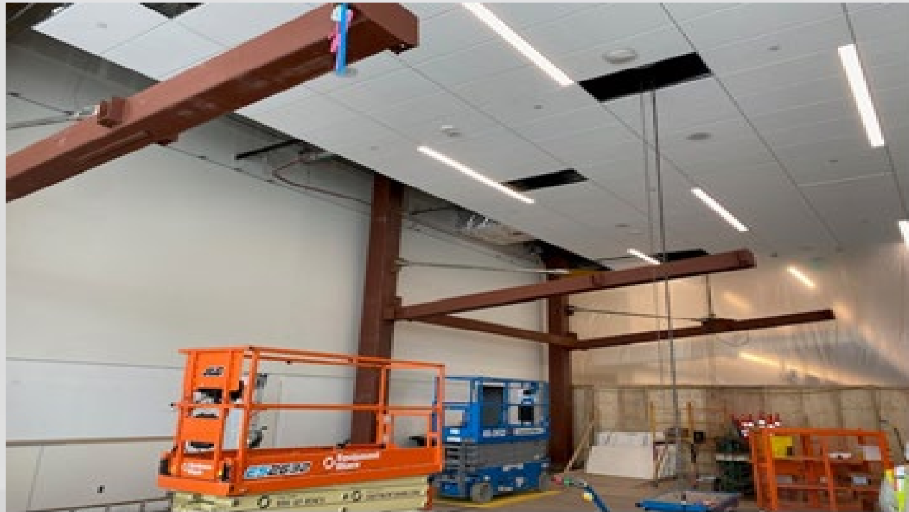
Ticket Counter Expansion Steel
