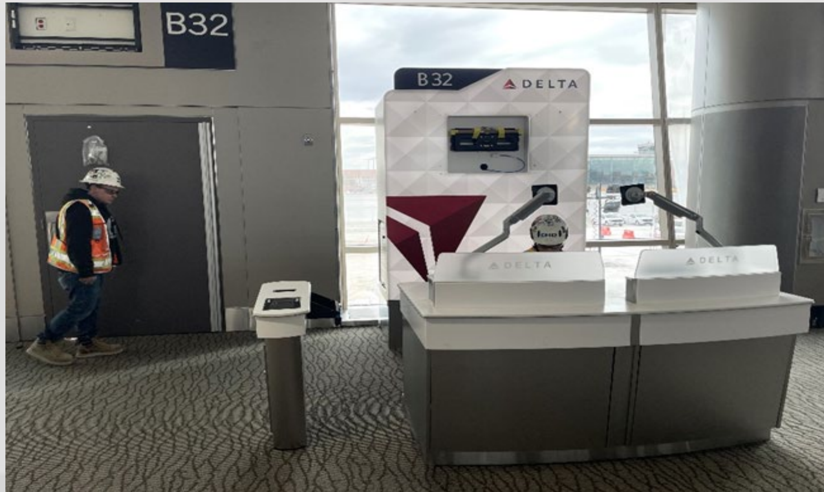
B32 Holdroom Millwork First Install
