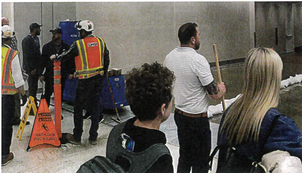
A ground water leak did not impact flights after it flooded a tunnel connecting gates at the Salt Lake City International Airport on March 11, 2024. (Photo: Courtesy of Justin Christensen)
