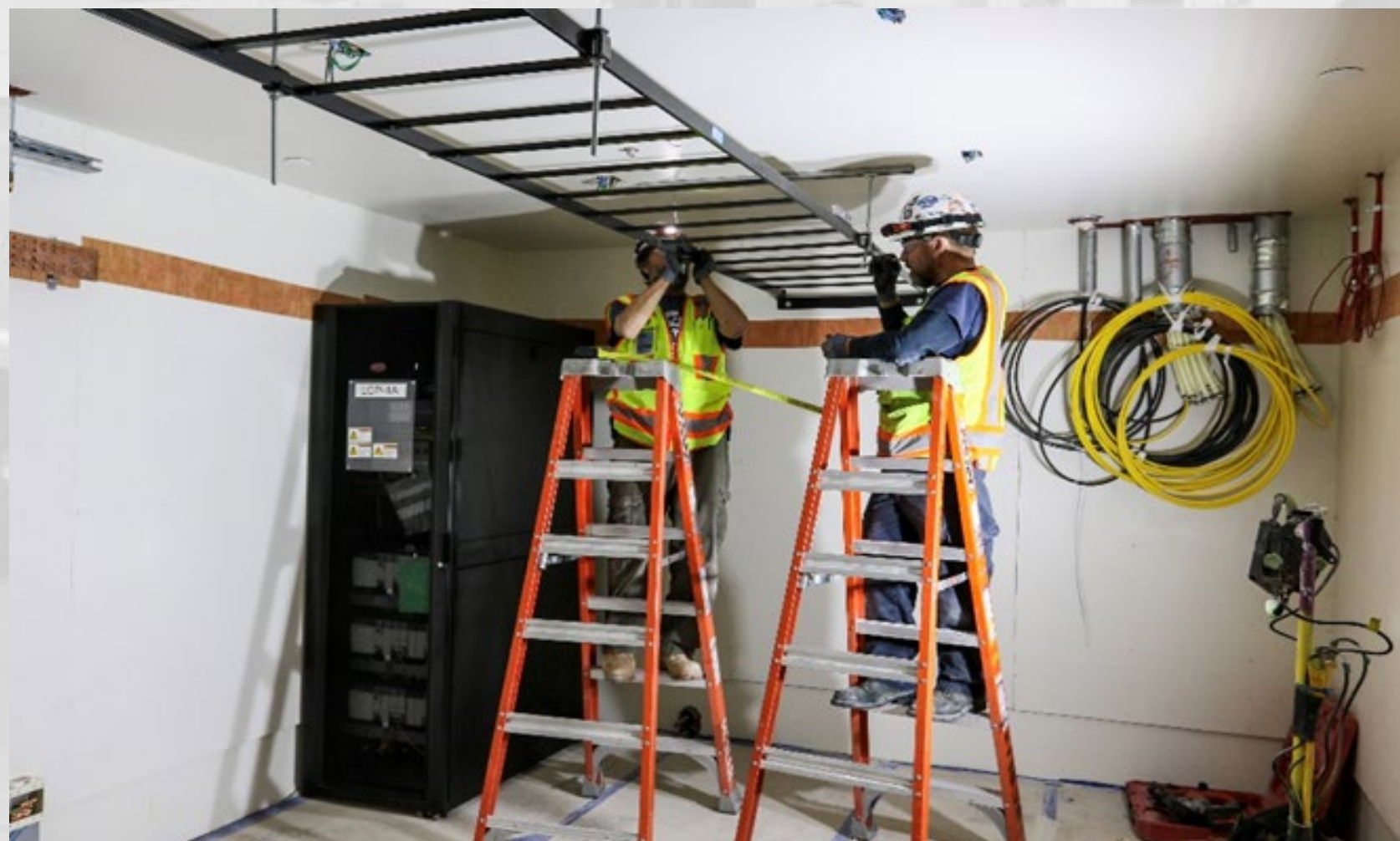
Comm Room Progress
