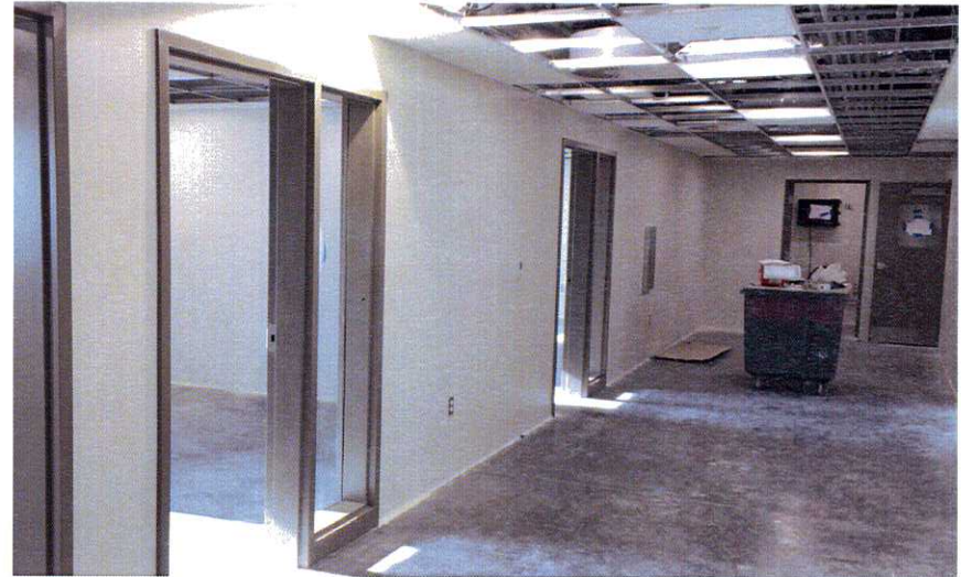
Interior Progress in RSS 'A' Admin Area.
