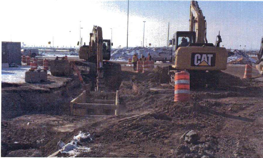
QTA West Area Temporary Storm Line.
