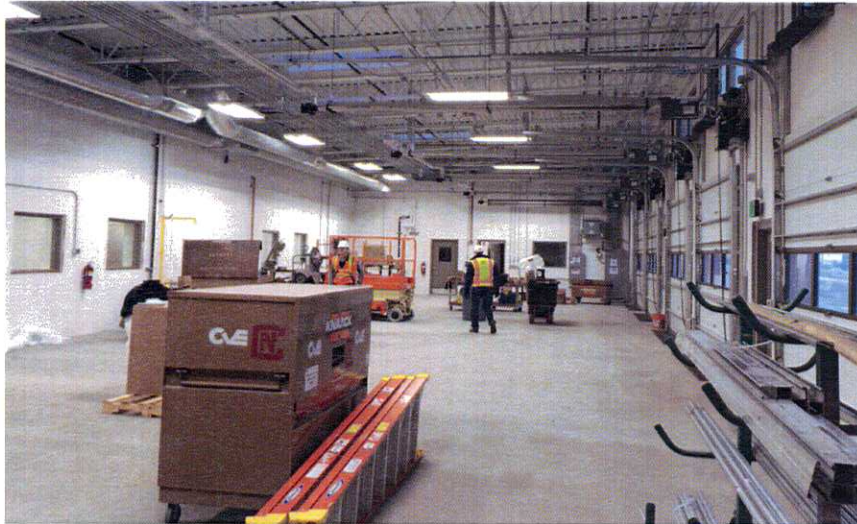
RSS 'C' Work Bay progress.
