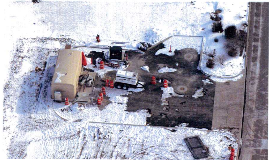
South Lift Station during interior wet well epoxy coating process.
