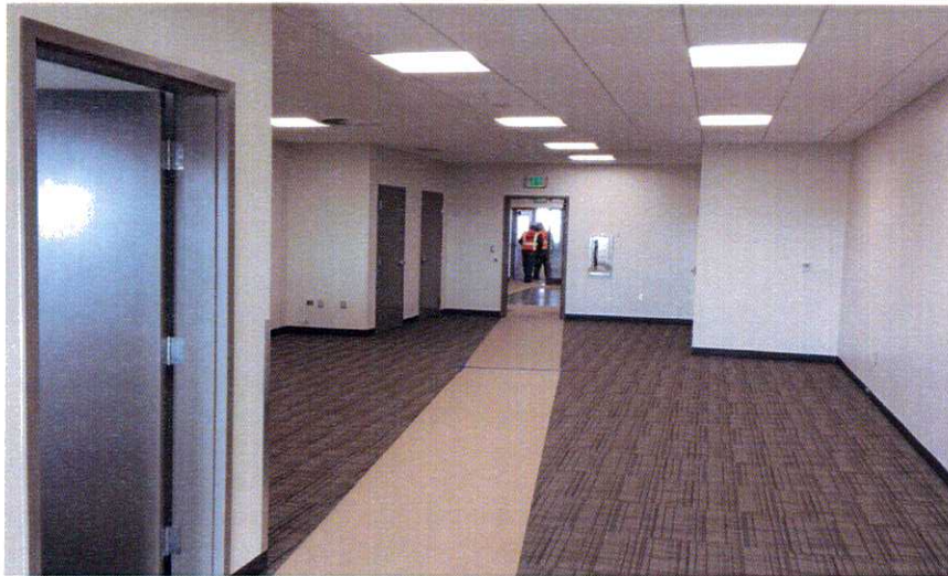
QTA Admin Build-out, Ceiling Tile, Carpet, Lighting, Final Paint.
