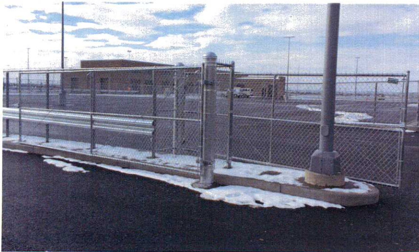
Typical RSS security fencing, guard rail, and gate.
