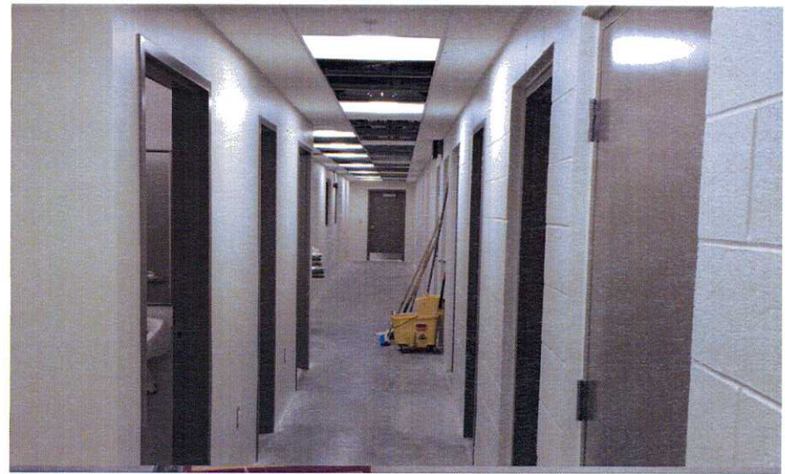
Admin Area Progress in RSS 'C'.
