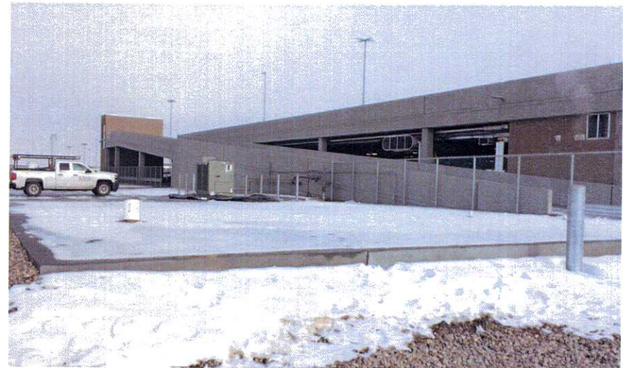
QTA trash compactor slab.
