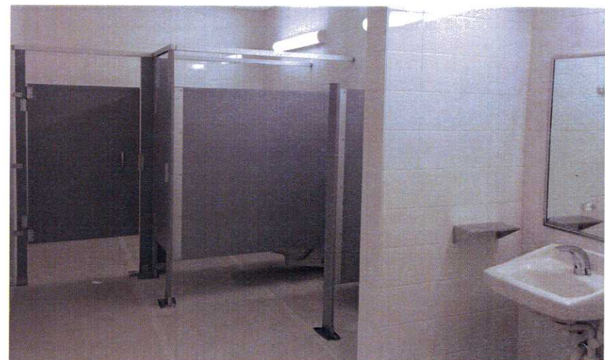
QTA Restroom build-out, Toilet Partitions and Fixtures.
