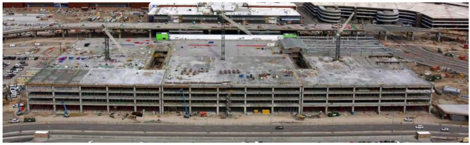
Parking Garage looking north – Roof Steel Erection underway
