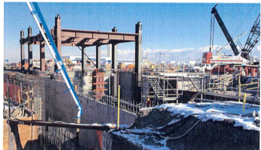
North Tunnel Basement wall construction
