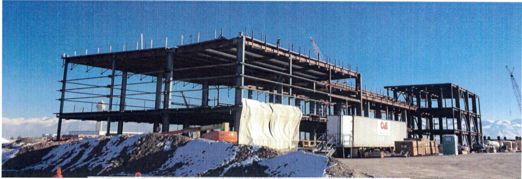
North Concourse Steel erection looking northeast, Sectors 'A' and 'BN'
