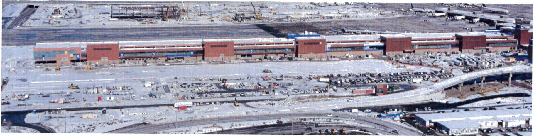
SCW Building Exterior – Areas 'A' through 'H', looking north
