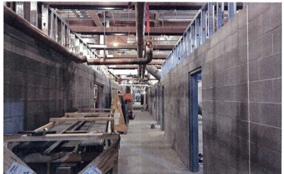
Terminal Service Corridor Level 1
