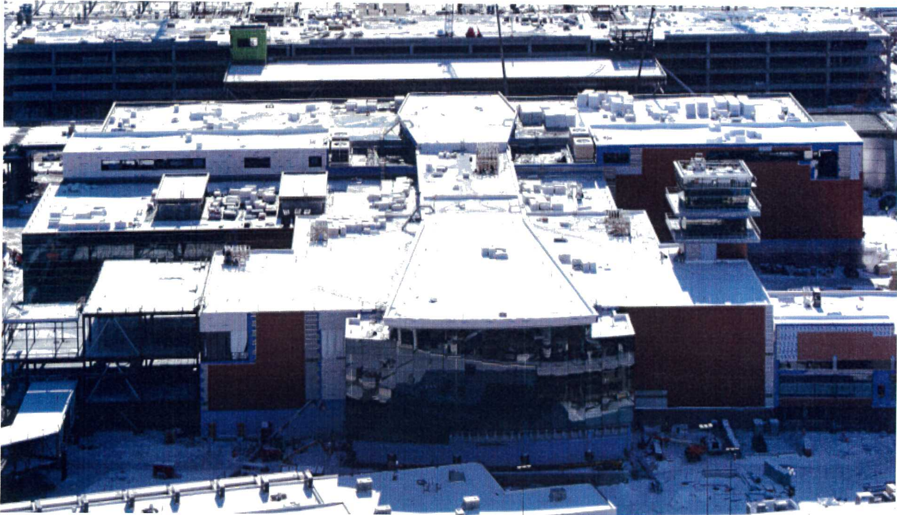
Terminal looking south
