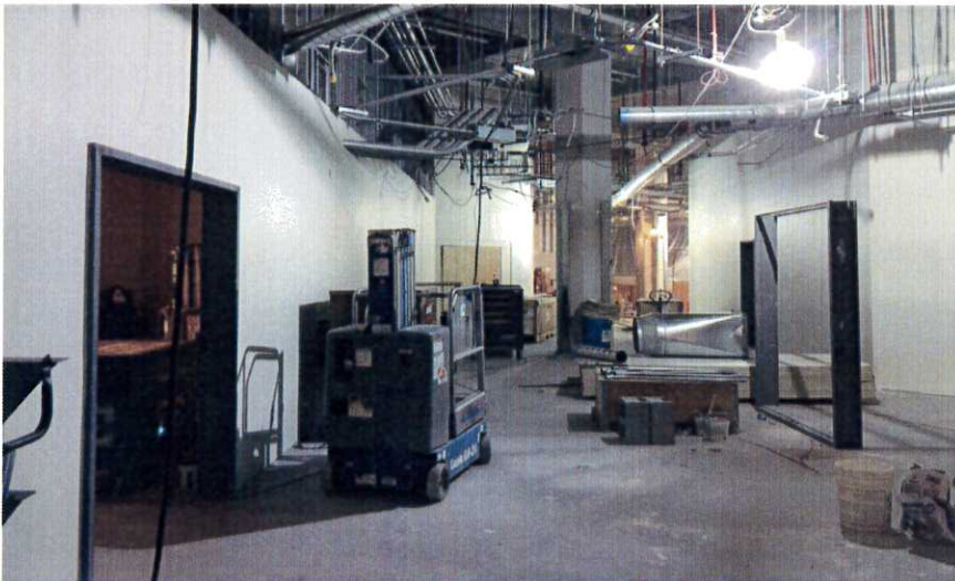
Terminal Basement Level 0 progress
