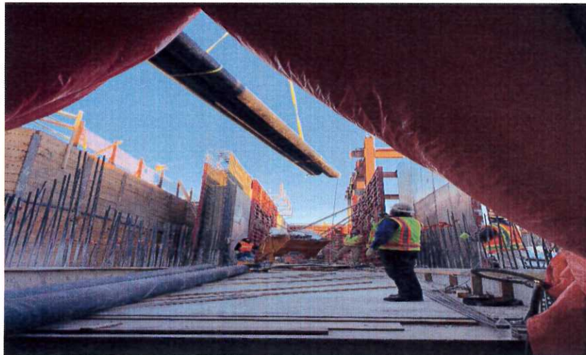
North Concourse Basement End of Mid-Concourse Tunnel
