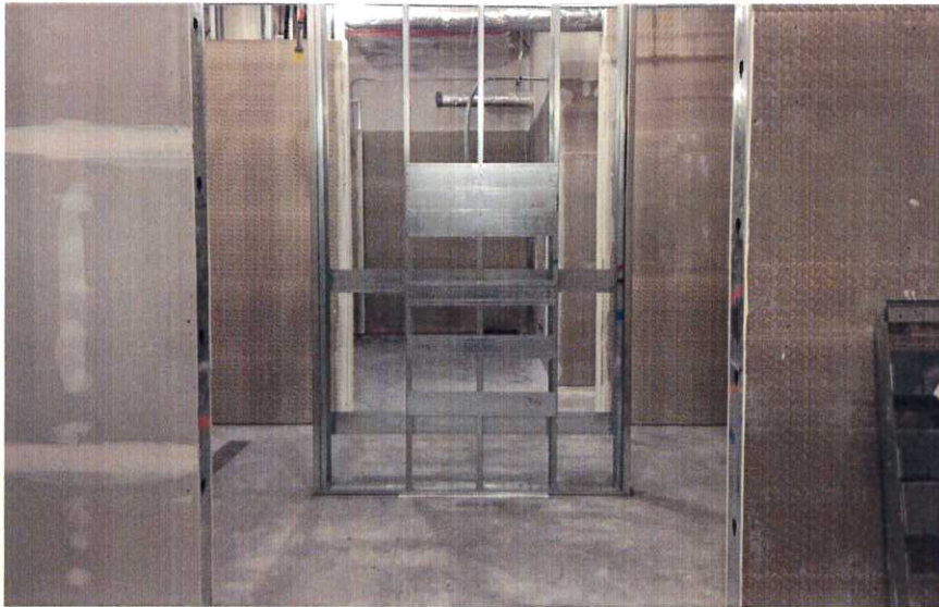
Terminal Restroom Level 2
