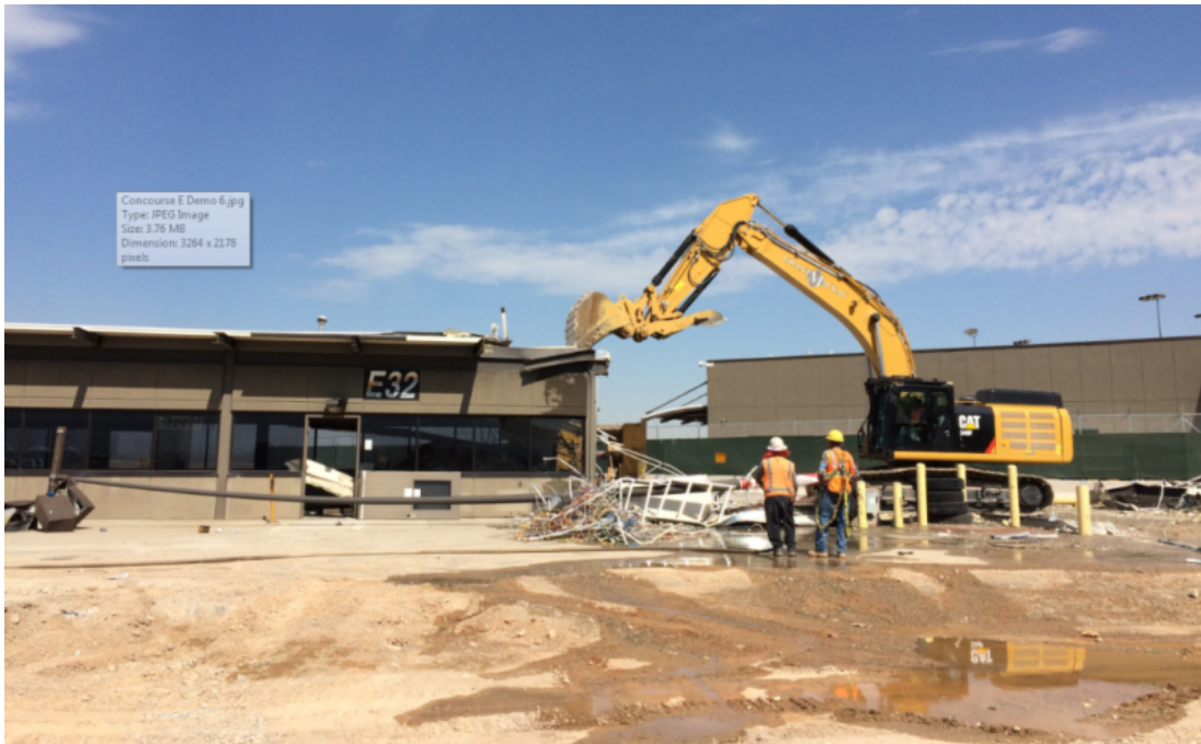
Construction crew members oversee demolition of Concourse E-south wing
