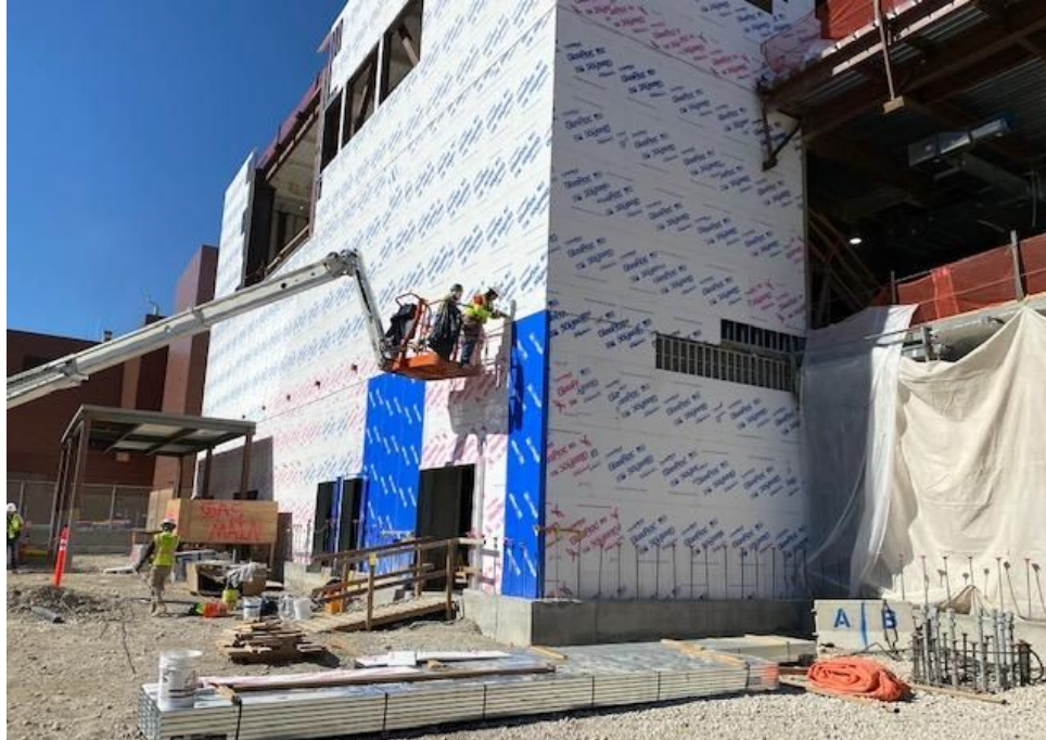
Concourse A-east exterior sheathing installation.
