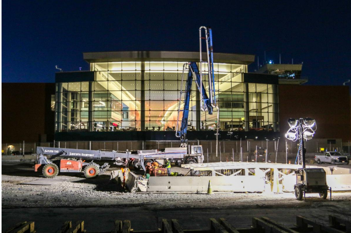
Sealing the final lid opening of the Central Tunnel
