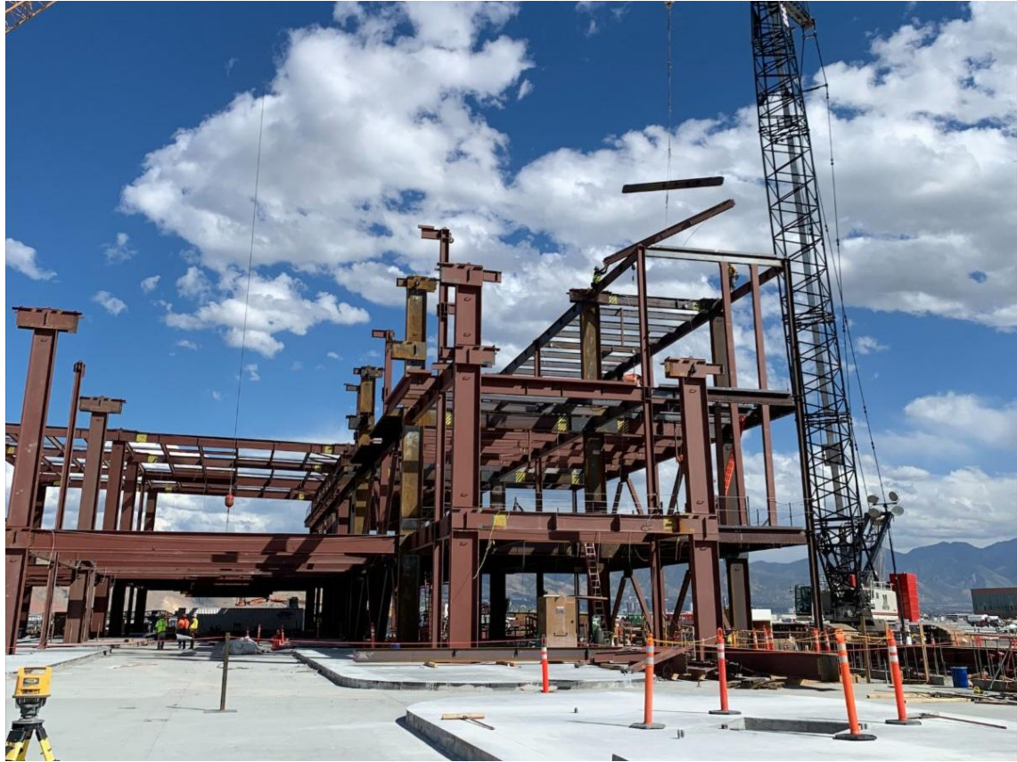
Erecting steel for Concourse B-east
