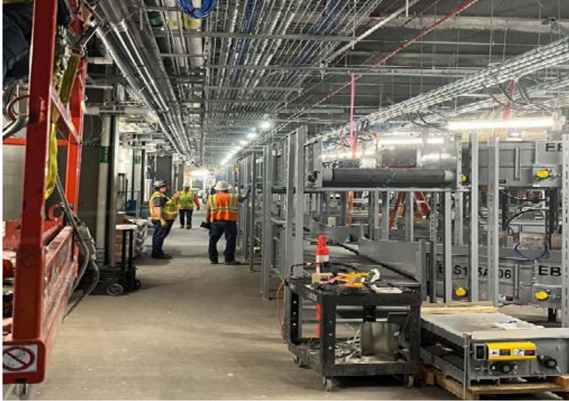
Installing the early bag storage system
