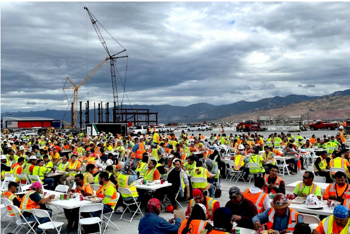
Airport Redevelopment Program workers enjoy a BBQ lunch to celebrate reaching 12 million craft hours on the project, as Concourse B-east takes shape in the distance.
