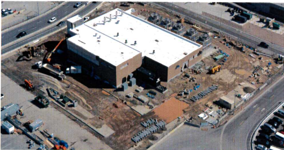
Central Utility Plant looking northeast
