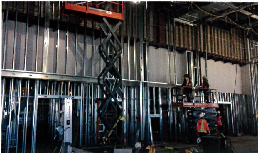
Drywall and metal stud installation in SCW
