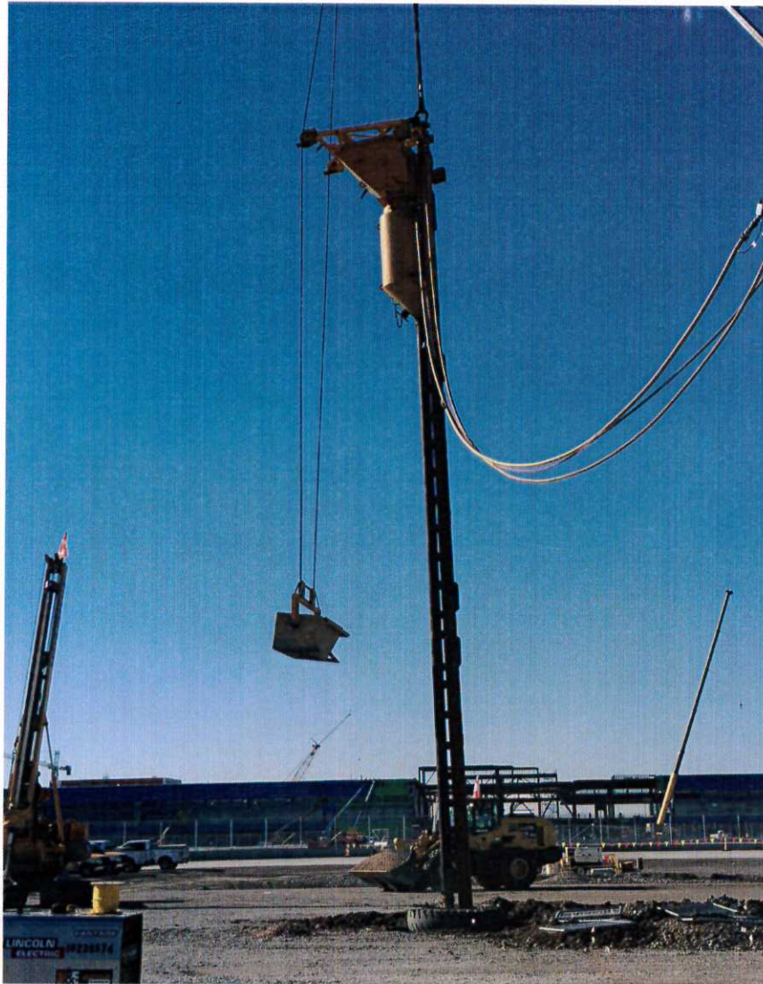
Start of Stone Column Installation
