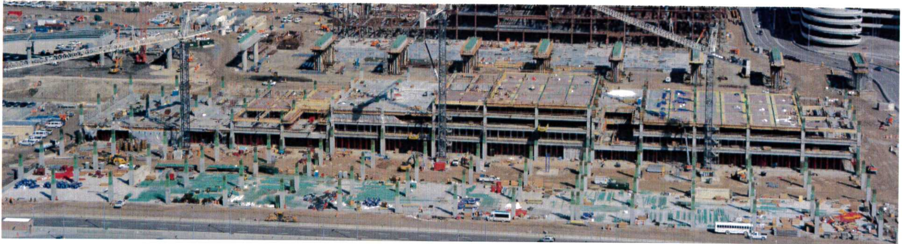
Parking Garage looking north
