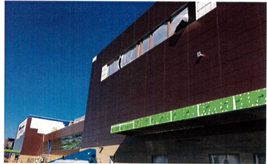
Metal panel installation at the SCW nodes
