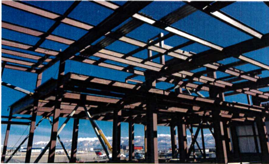
Mid-Concourse Tunnel area steel erection
