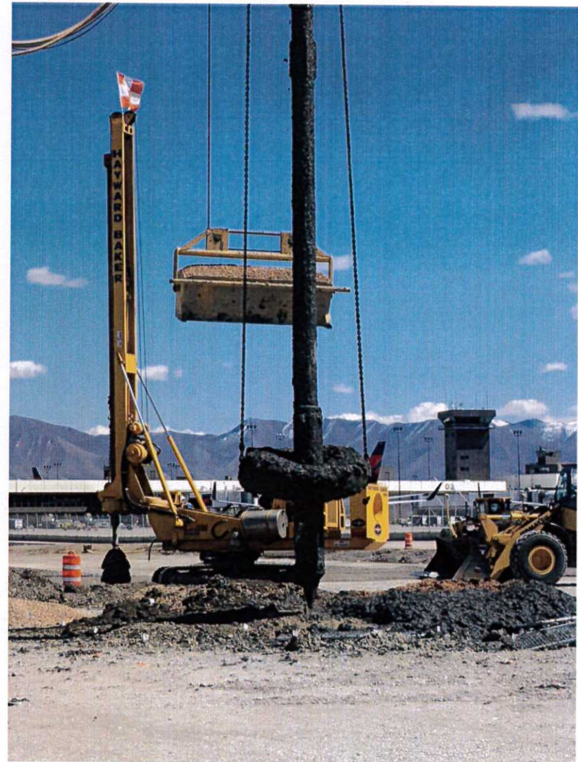
Stone Columns Underway
