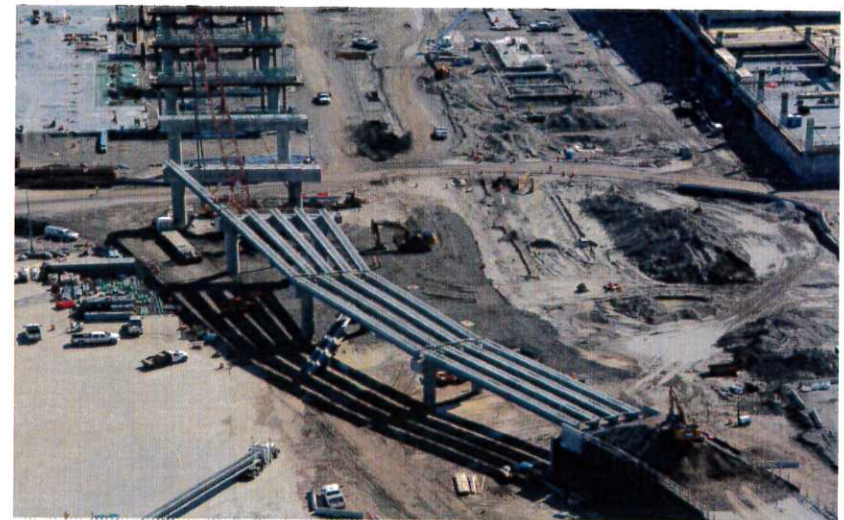
Elevated Roadway Bridge Girders looking east
