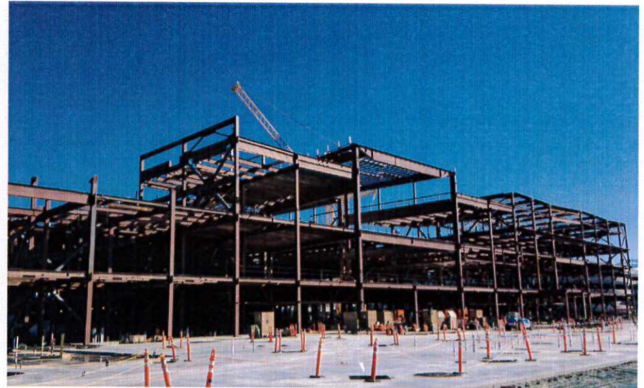
Terminal Building steel, including Area G
