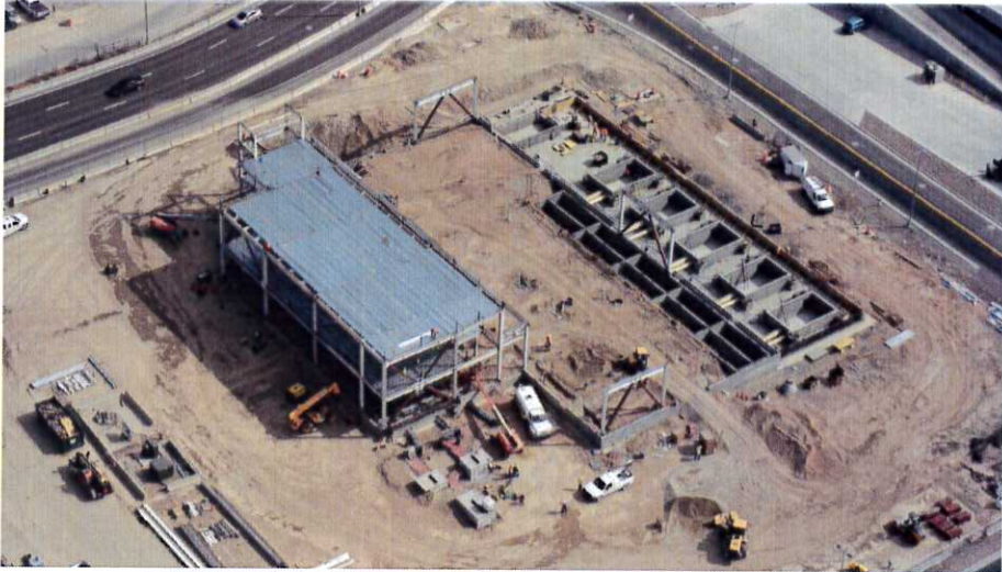
Central Utility Plant (CUP) structural steel erection
