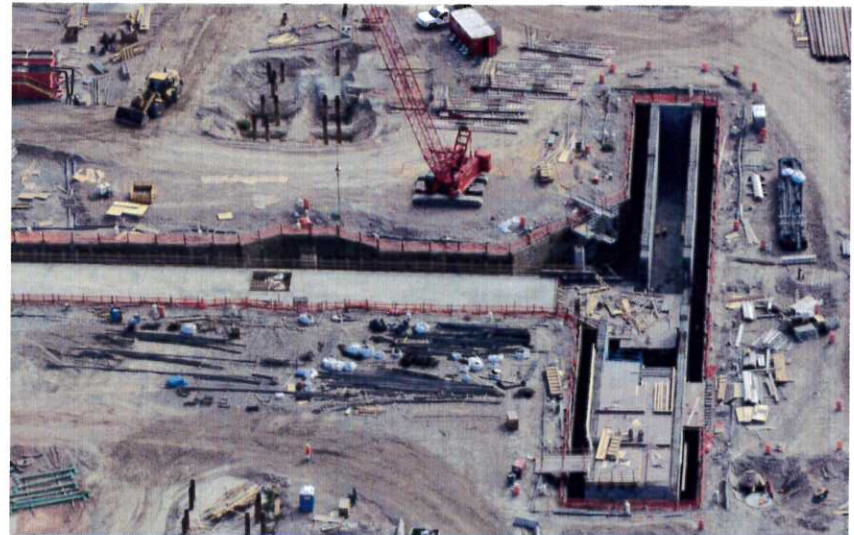
Progress at the south end of the Terminal/Gateway Tunnel
