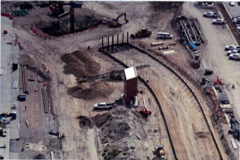
Elevated Roadway exit ramp construction
