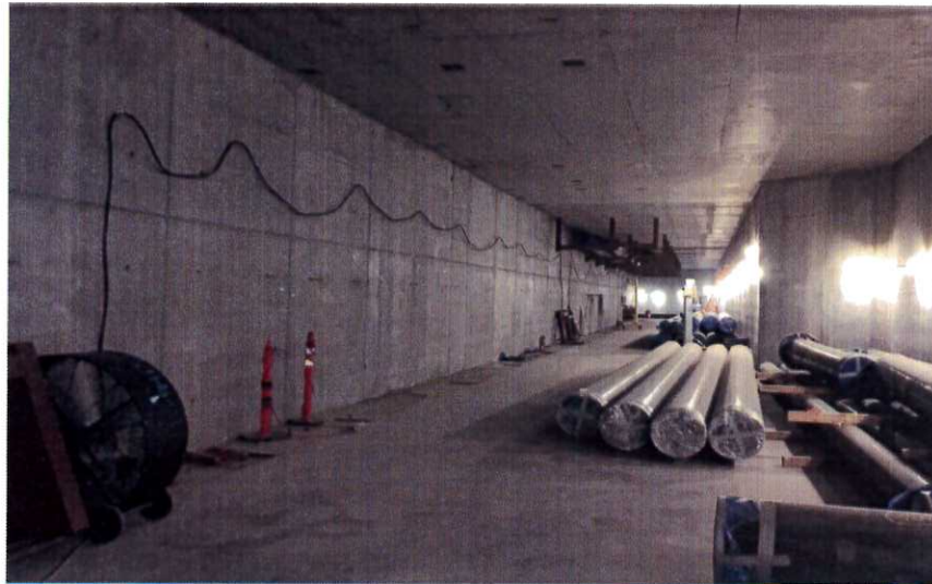
Terminal Tunnel installation of hydronic piping
