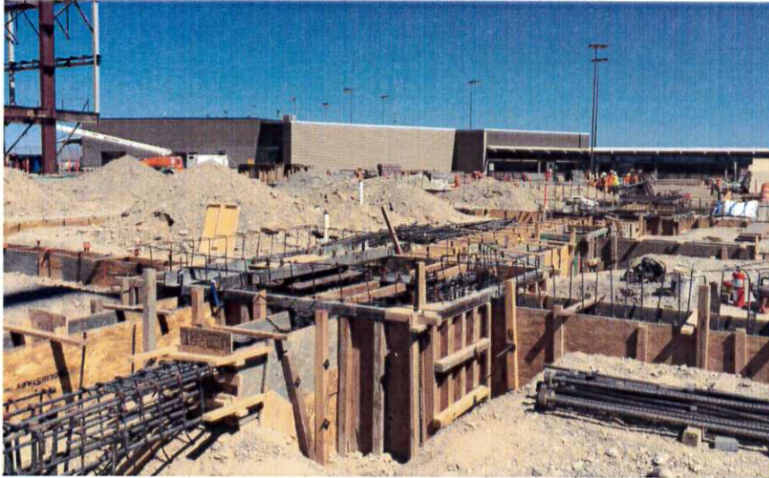
Pile caps and grade beam foundations for Level 1 slab
