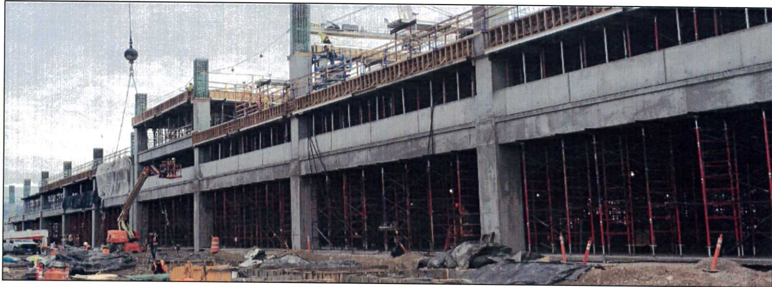
Formwork for Parking Garage Level 4
