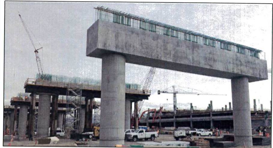
Completion of first Elevated Roadway bent
