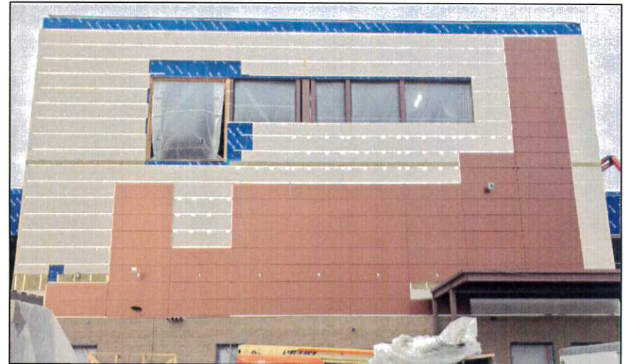
Metal panel installation at the SCW nodes
