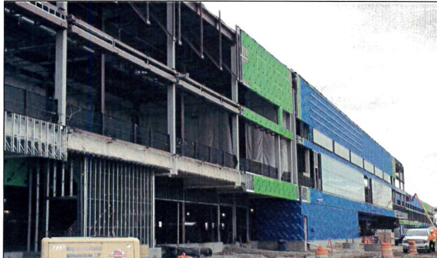
North Façade window wall installation on SCW
