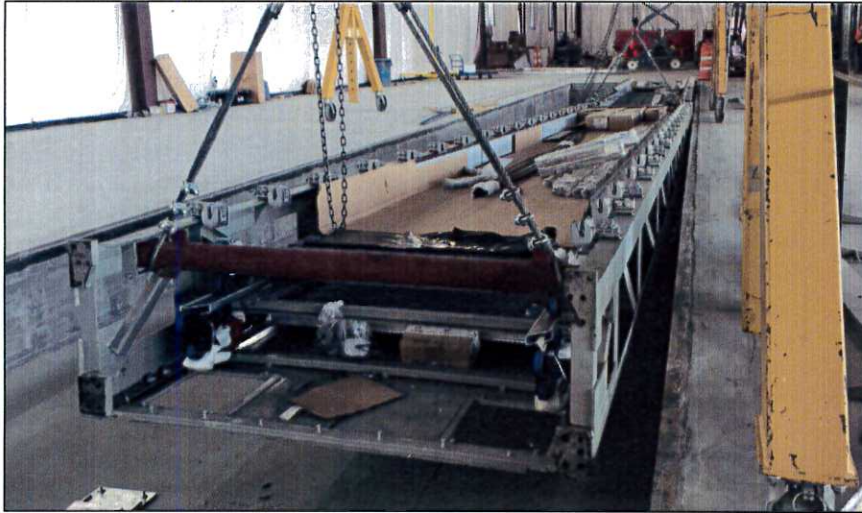
First moving walkway hoisted into place in SCW
