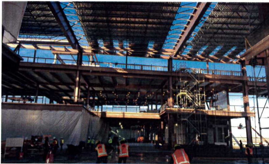
Upper Floors of the Terminal Building
