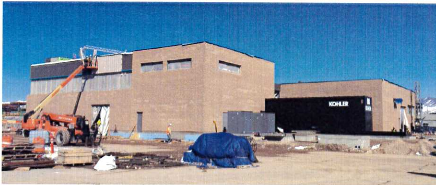
Central Utility Plant progress
