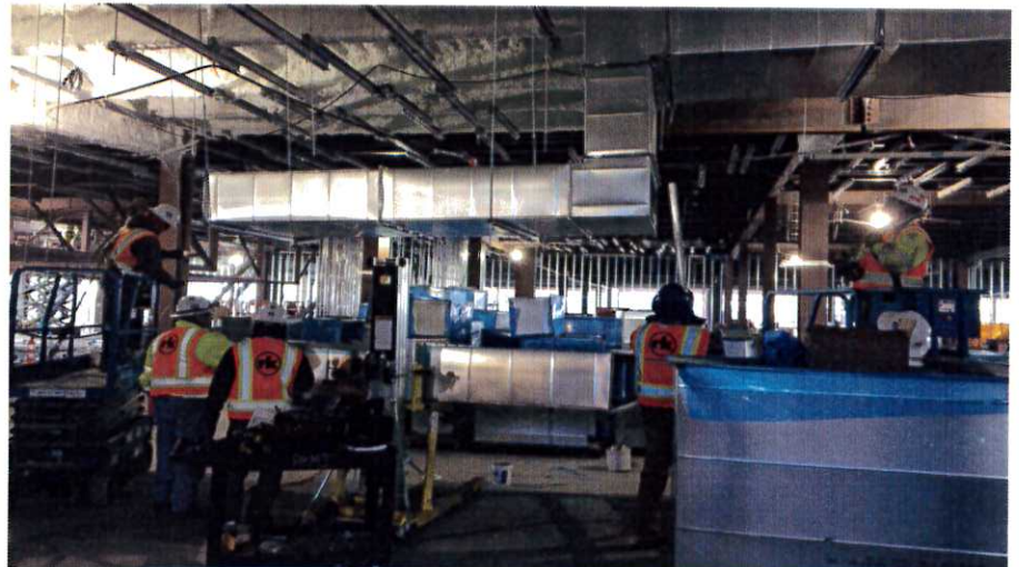
In addition to the ductwork, BHS header steel and interior wall studs are visible.
