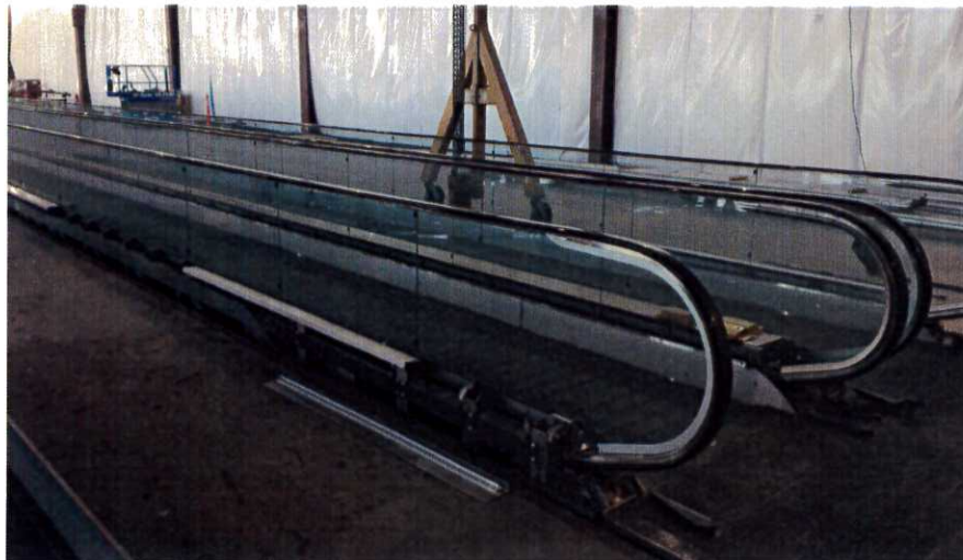
Escalator Installation at SCW
