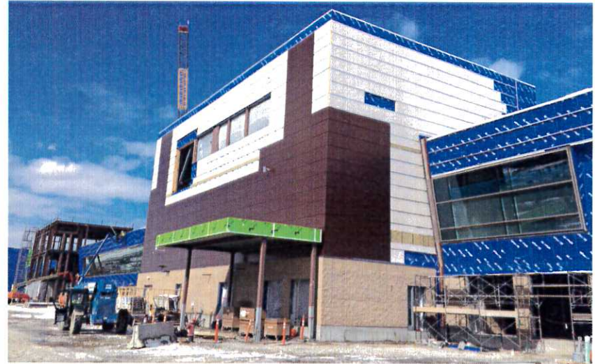
Metal panel installation at the SCW nodes
