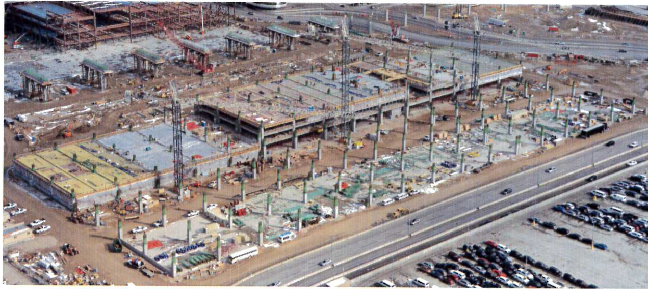
Parking Garage Progress
