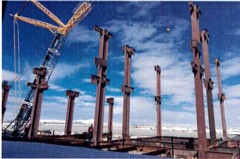
Mid-Concourse Steel progress.
